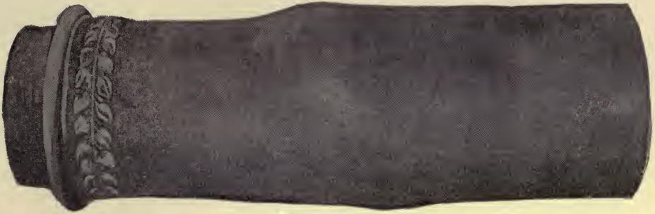
Column taken from Western Union Building (New York City) after fire.
