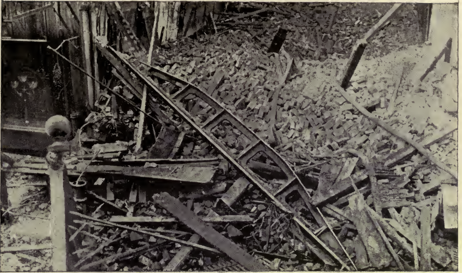
OLD-FASHIONED CAST-IRON LINTEL.
