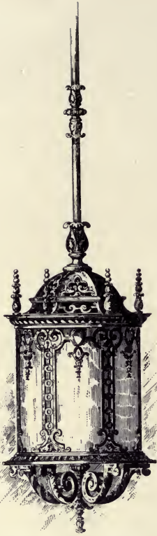
Lantern in Vestibule of Georgian Court.
