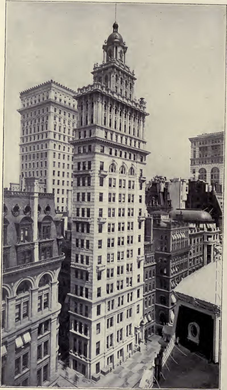
FIG. 2.—AMERICAN SURETY BUILDING (IN BACKGROUND.) (View from Southeast.)
