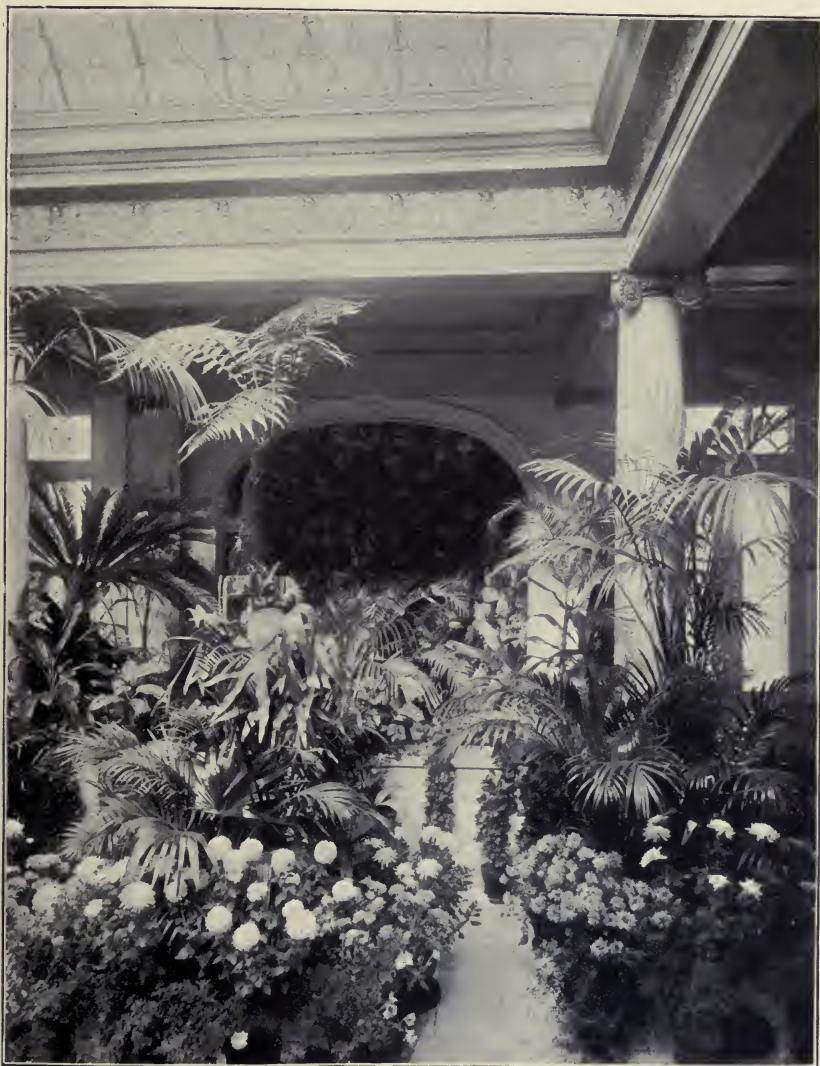
CORNER IN CONSERVATORY, GEORGIAN COURT.
