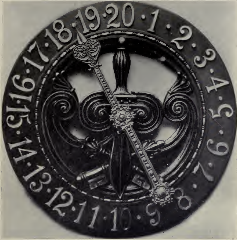
FIG. 4.—ELEVATOR INDICATOR, AMERICAN SURETY BUILDING.
