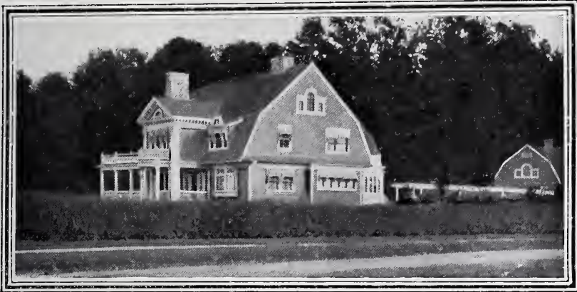
FIG. 9. HOUSE AT PLAINFIELD, N. J.
