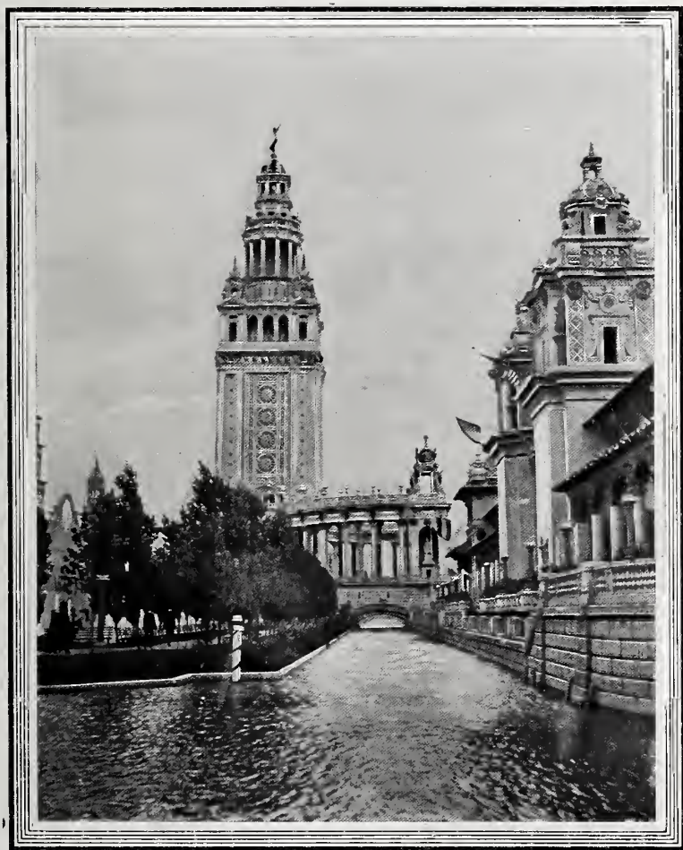
THE ELECTRIC TOWER. A LATERAL VIEW.
