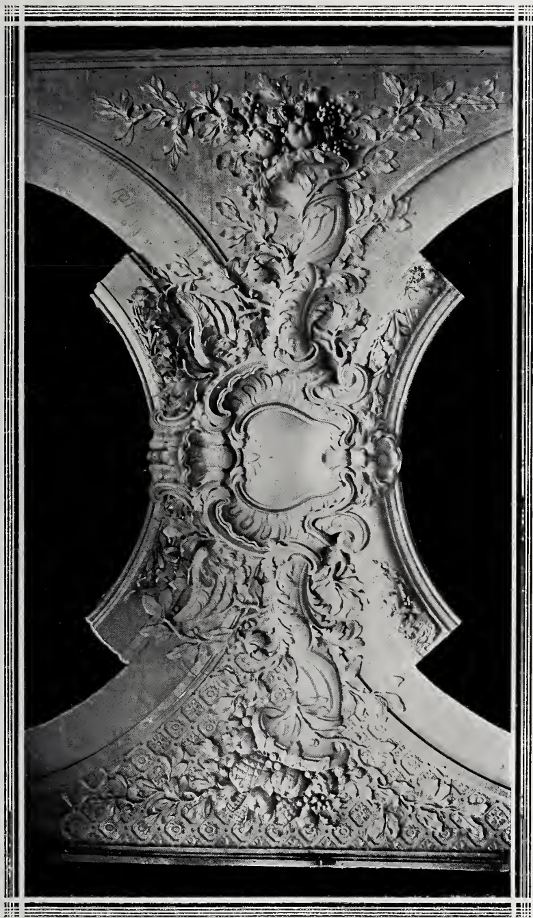
FIG. 15. QUAI D'ORSAY STATION.—A DECORATIVE DETAIL.
