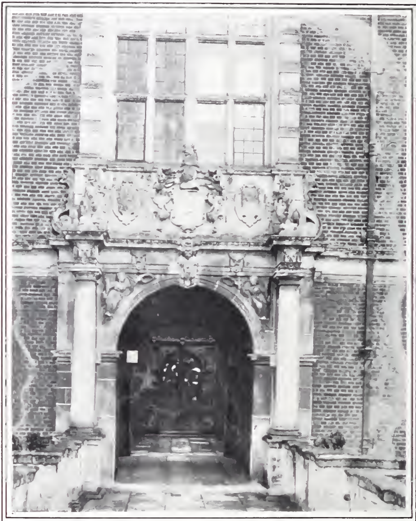
PLATE III. BLICKLING HALL.—This is a view on a still larger scale of the doorway taken by itself. The armorial bearings over the front door are stated to be those of the builder, Chief Justice Hobart, and this is highly probable; the escutcheon in the middle is charged with an inescutcheon bearing the open left hand which indicates the rank of a baronet; that is to say, of a wholly new order of honor, especially founded by James I. The quartered field, though much defaced, can still be made out in its more important features. The decorative escutcheons at the two sides are almost wholly defaced. The monsters set upon the two ressauts above the columns are bulls supporting escutcheons, presumably the supporters of Sir Henry Hobart's arms; and they are repeated with slight modifications on the two pillars which flank the bridge. The crest seen above the carved stone helmet is a bull's head and neck.
