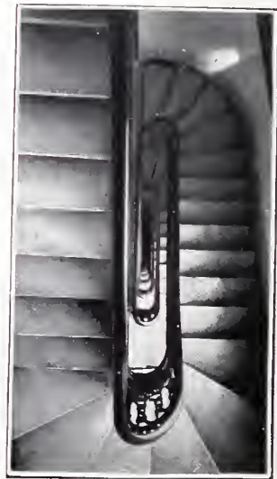
Staircase, Bourne Office Building, New York.
