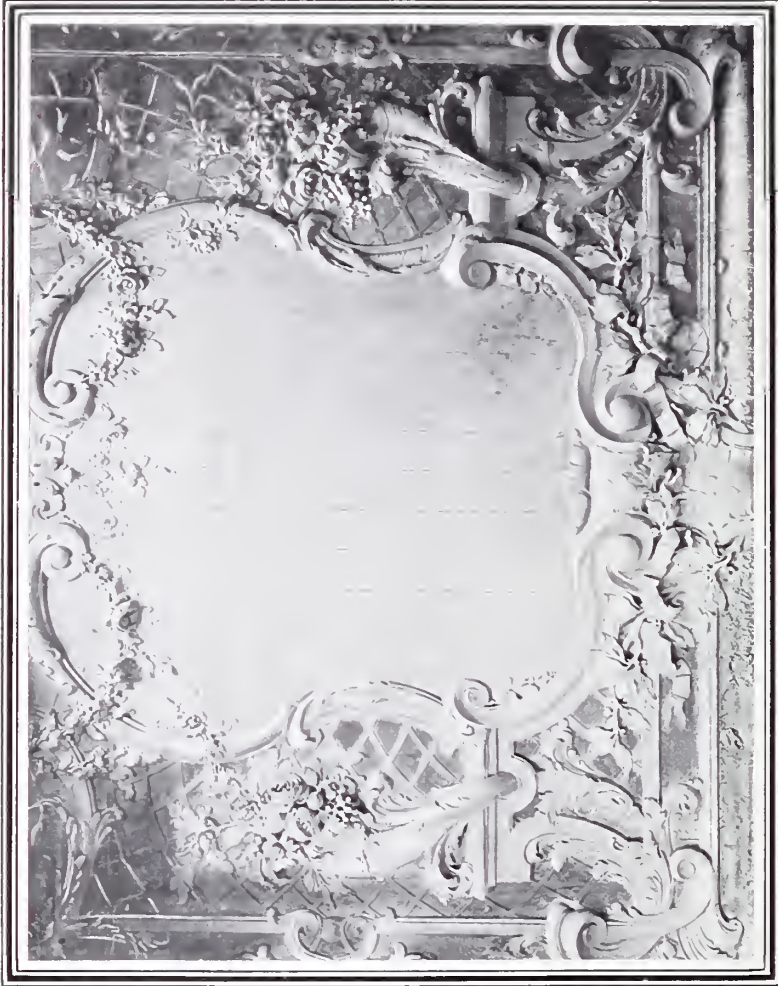
FIG. 14. QUAI D'ORSAY STATION.—A DECORATIVE DETAIL.
