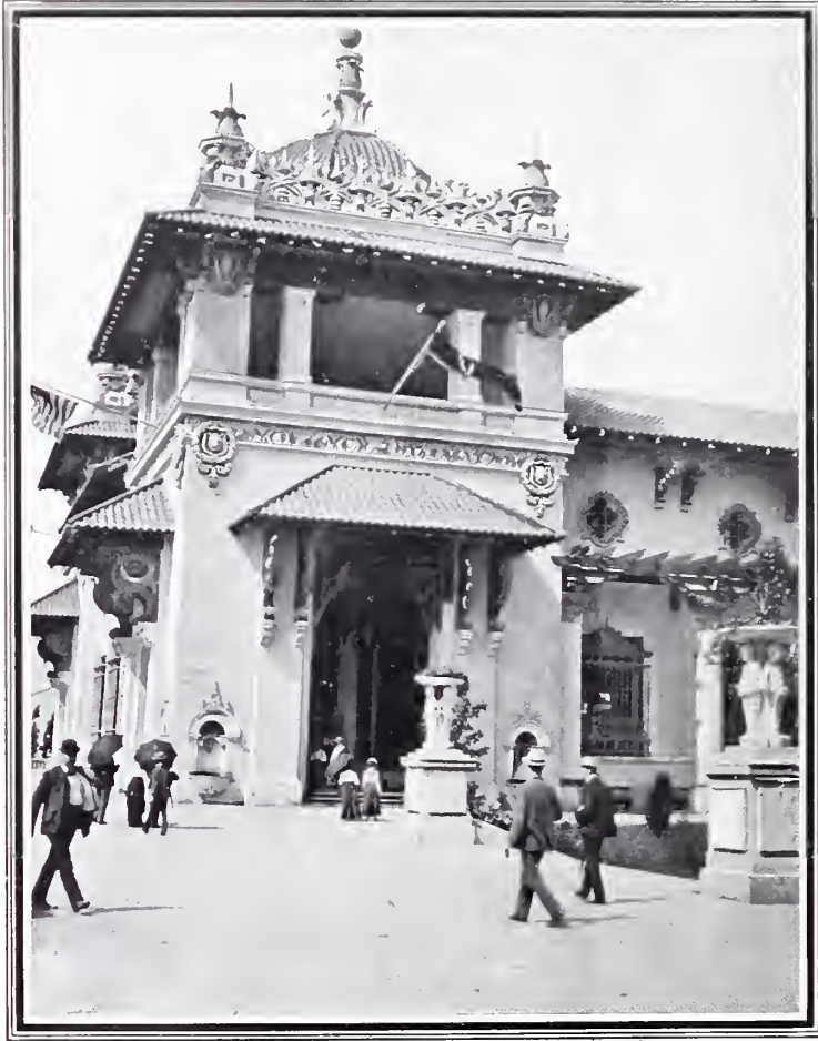
A CORNER OF THE MACHINERY BUILDING.
