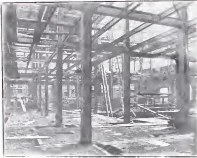
Connecticut Mutual Building, Hartford, Conn.
