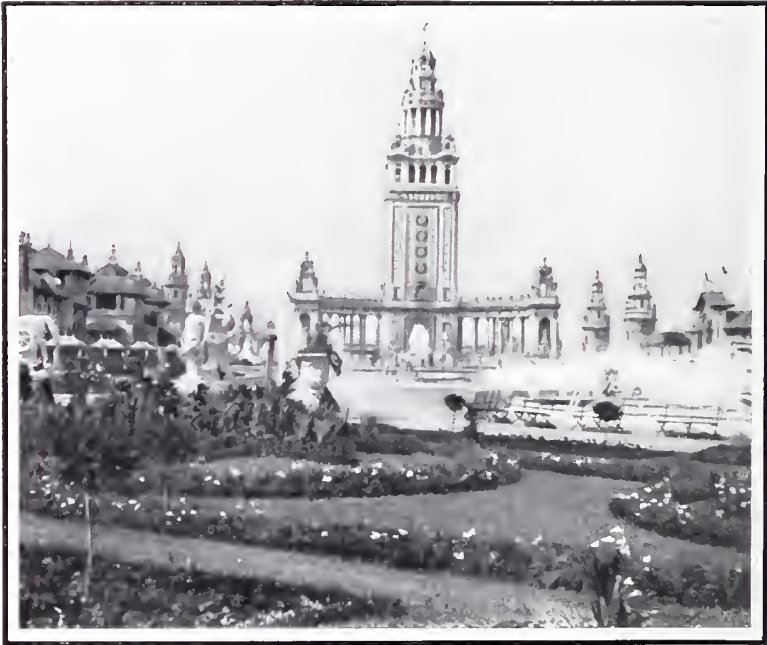
THE ELECTRICAL TOWER. A DIAGONAL VIEW.
