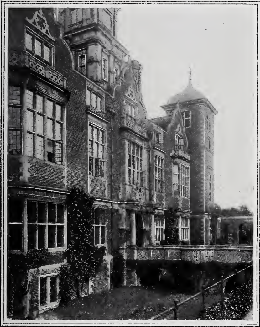
PLATE IV. BLICKLING HALL.—This illustration shows the west front from the northwest in steep perspective, and here we understand better the form of the bridge as well as the amount of projection of the columns and door-piece, and the bay-window above. There is certainly a very successful piece of proportioning in the gradual retreat of these projections and in the placing of the statuettes above to correspond with the heraldic supporters below, the whole leading gradually to the wall of the gable. The success in obtaining an architectural treatment of considerable importance, and sure to strike the eye of every beholder, while yet the materials are of the simplest and the expense incurred in stone-cutting proportionally very slight, is certainly worthy of great admiration.
