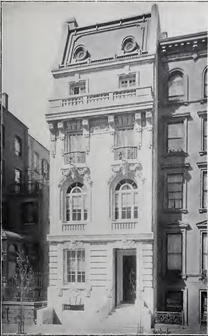
RESIDENCE, 35 EAST 68TH STREET.
