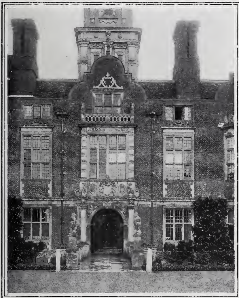
PLATE II. BLICKLING HALL.—The principal entrance on a larger scale than in Plate I., and it is interesting to see how the great bay-window over the entrance doorway, while it projects only a foot, more or less, from the brick wall, is given special consequence by the treatment of its stone flanking pieces as pilasters with a semblance of Ionic capitals and a decided frieze with swags above them, introduced in order that the window-head may have all the appearance of a full classical entablature. The two statuettes which occupy the corner pedestals of the parapet above the central bay-window have been introduced chiefly as echoes or repetitions of the heraldic monsters below. The free treatment of the heraldic creatures, their position being different, two attitudes used for each supporter, is characteristic of the days when heraldry was a real "power in the state," or at least in social matters.
