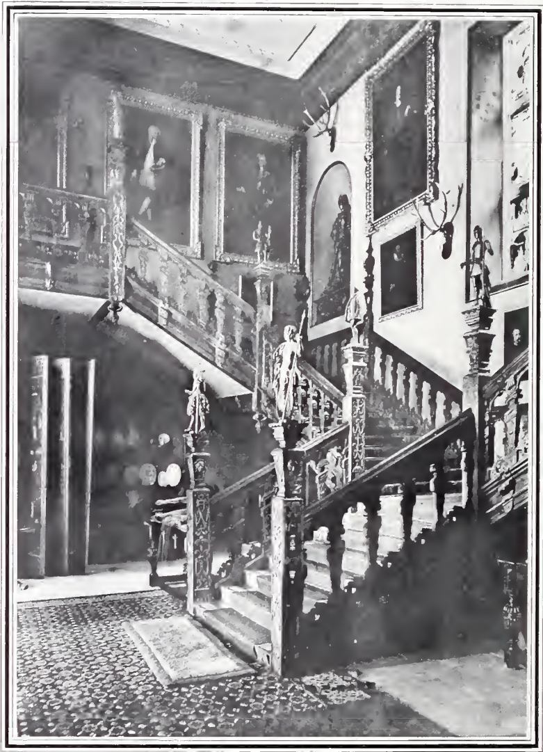
PLATE XI. BLICKLING HALL.—This illustrates the staircase with fine double stair of the same epoch as the house. The modern carpeting interferes with its dignity. There is no stair in England which is more rich in composition or in detail. Moreover, there is no instance of the raking or sloping capitals more agreeable and less of a solecism than the present one. The whole order of gables with Ionic capitals, now horizontal, as at the landing on the left, now sloping, as in all the ramps of the stair, is a remarkable achievement in conventional design. How far the statuettes on the newels are of the original epoch it is not safe to say, but they are strictly in keeping. The great window on the right looks out on an inner court. The large Oriental rug on the floor has been cut so as to fit around the foot of the stair, which seems a piece of vandalism; but it may be that the piece has not been removed but merely folded under, in which case it can be with partial success put in place again and repaired.
