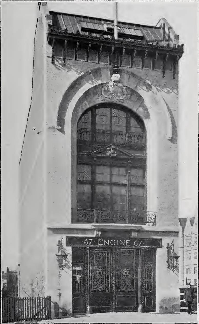
FIG. 46. FIRE-ENGINE HOUSE IN 170TH STREET.
