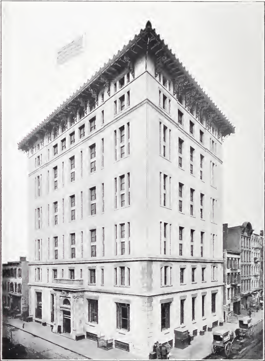
FIG. 43. MILLS HOUSE NO. 2, RIVINGTON STREET, NEW YORK CITY.
