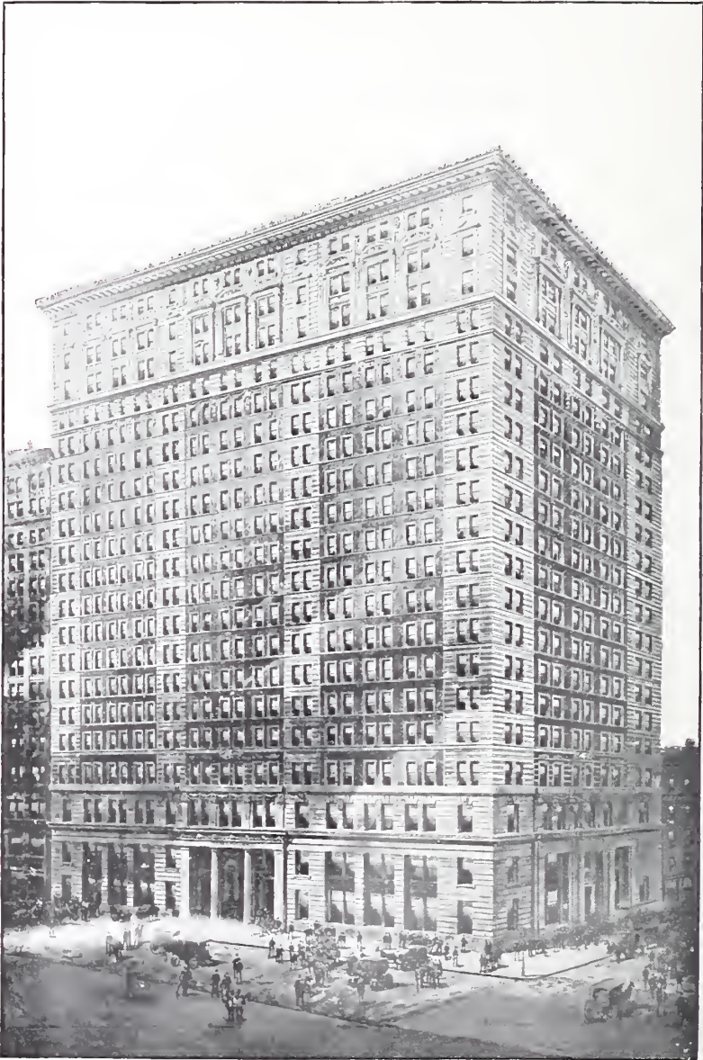
THE BROAD-EXCHANGE BUILDING.
