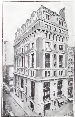
The Singer Building. Ernest Flagg, Architect. C. T. Wills, Builder.
