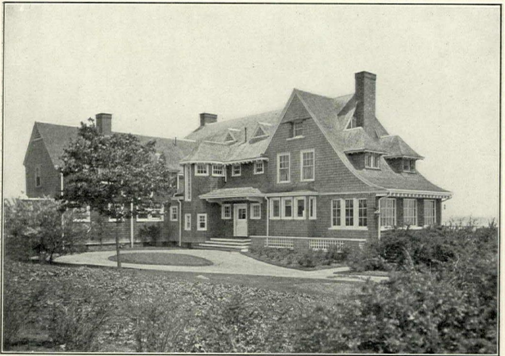
View from the Driveway.
