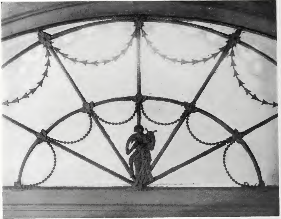
DETAIL OF FANLIGHT OVER THE FRONT DOOR OF THE HOPPER HOUSE.
