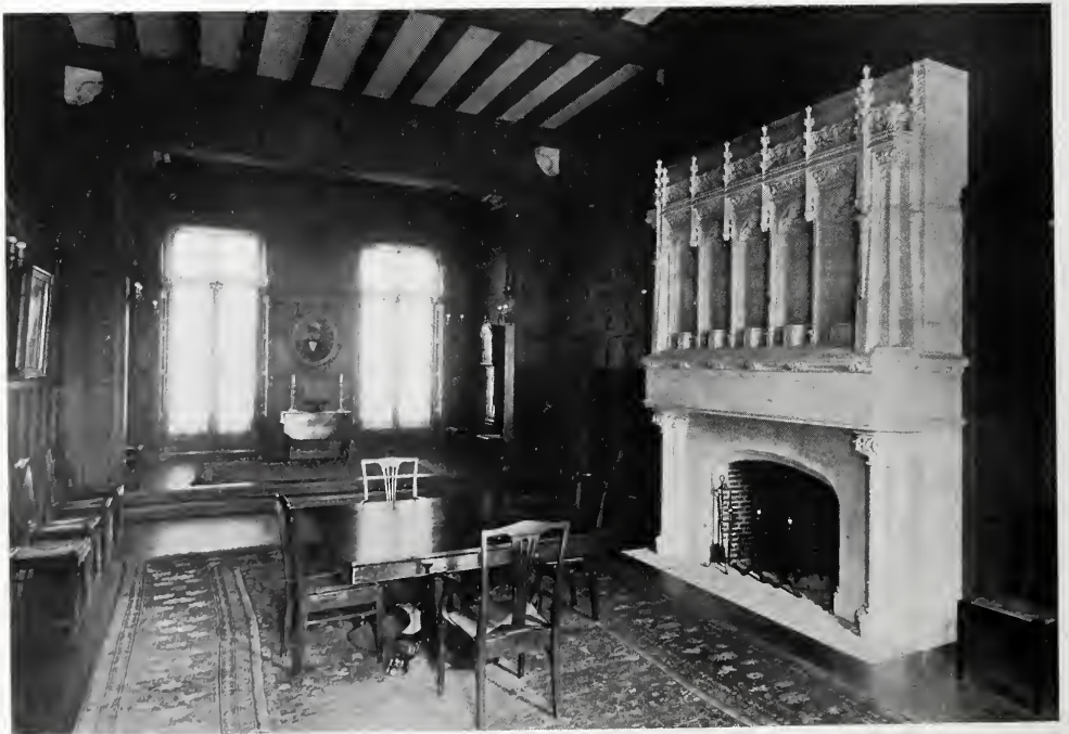
DINING ROOM—BISHOP'S HOUSE AT THE CATHEDRAL OF ST. JOHN THE DIVINE, NEW YORK. Cram, Goodhue & Ferguson (Boston Office), Architects.
