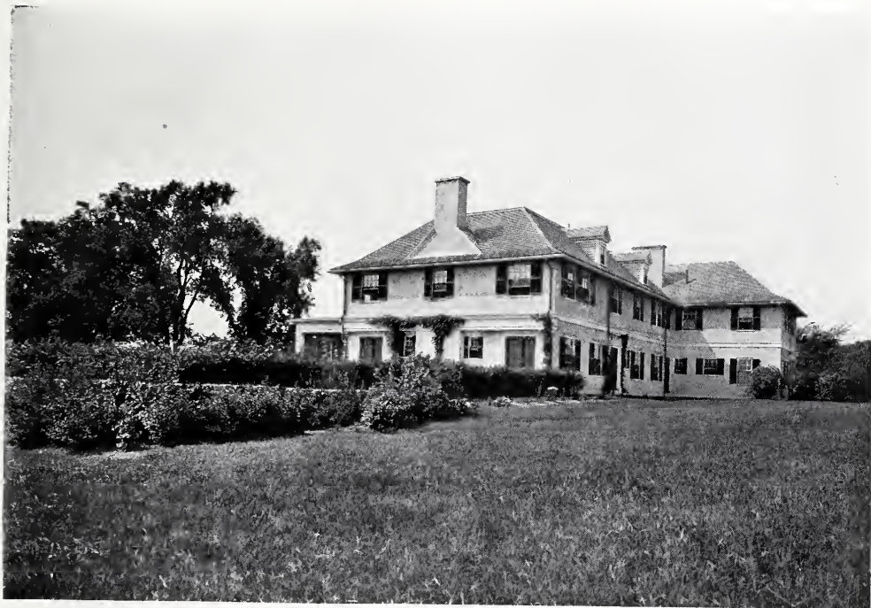
NORTH AND EAST FRONTS—RESIDENCE OF MRS. GENEVIEVE N. FULLER, DOVER, MASS. Kilham & Hopkins, Architects.
