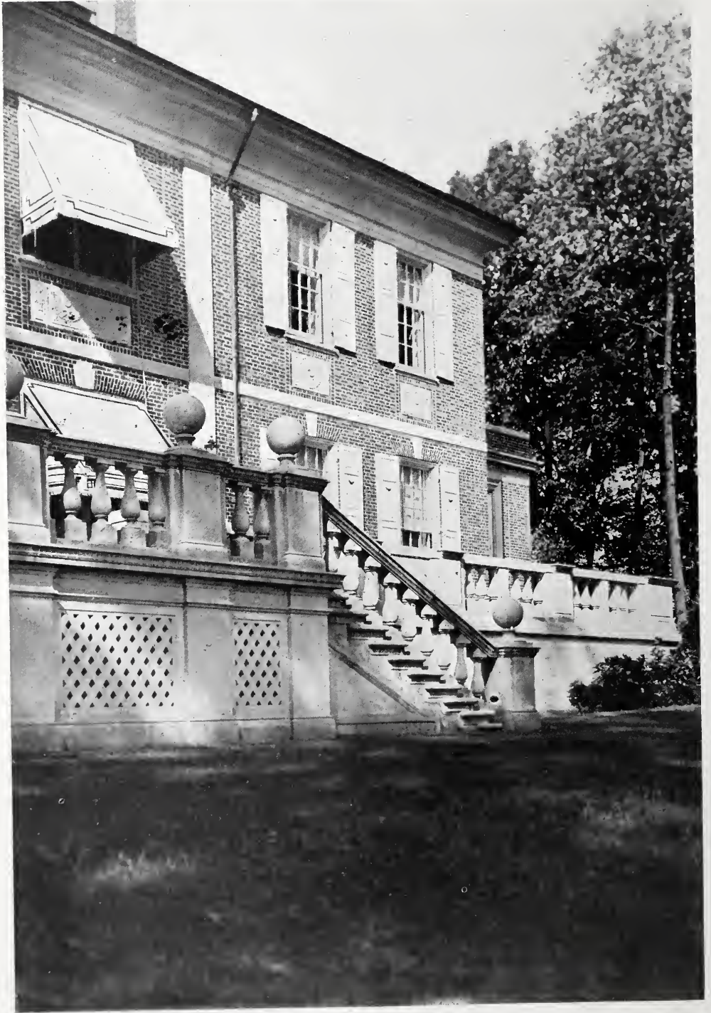
TERRACE FRONT, HOUSE OF JAMES PARMELEE, ESQ., WASHINGTON, D. C. CHARLES A. PLATT, ARCHITECT.
