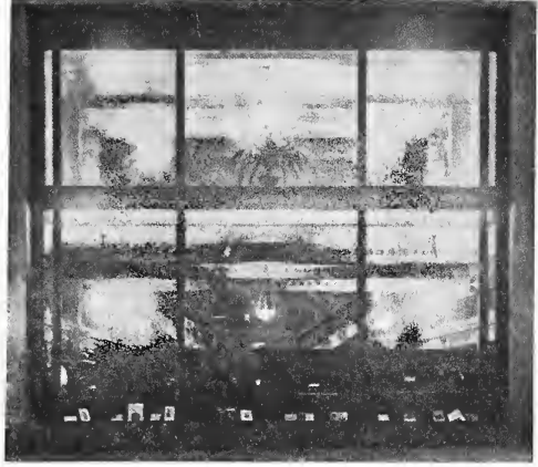
Fig. 3. Improvement effected by utilizing every third outlet, with silver-plated reflectors behind a valance.
