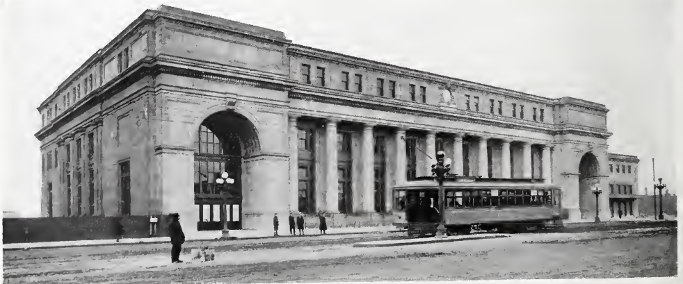
STREET FRONT OF THE GREAT NORTHERN STATION AT MINNEAPOLIS. Charles S. Frost, Architect.
