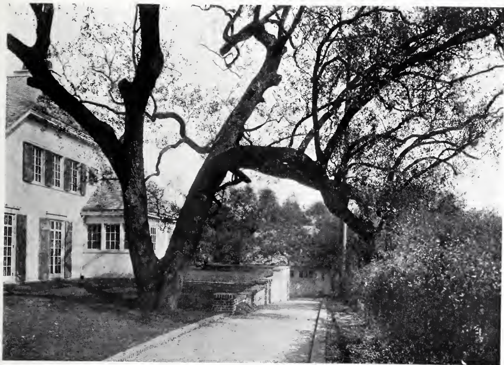
GARDEN OF THE RESIDENCE OF J. H. BURNES, ESQ., PASADENA, CAL. Myron Hunt and Elmer Grey, Architects.
