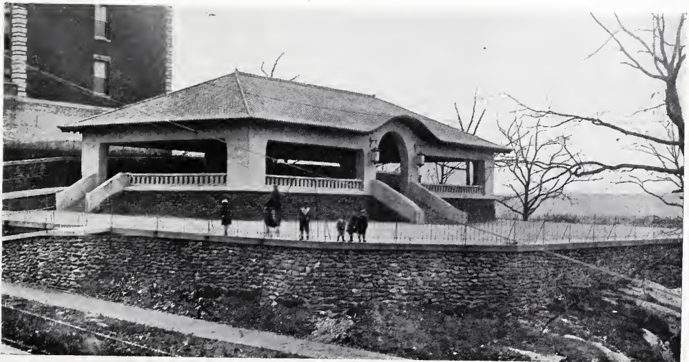
REST HOUSE IN COLUMBUS PARK, YONKERS, N. Y. Harold A. Caparn, Landscape Architect.
