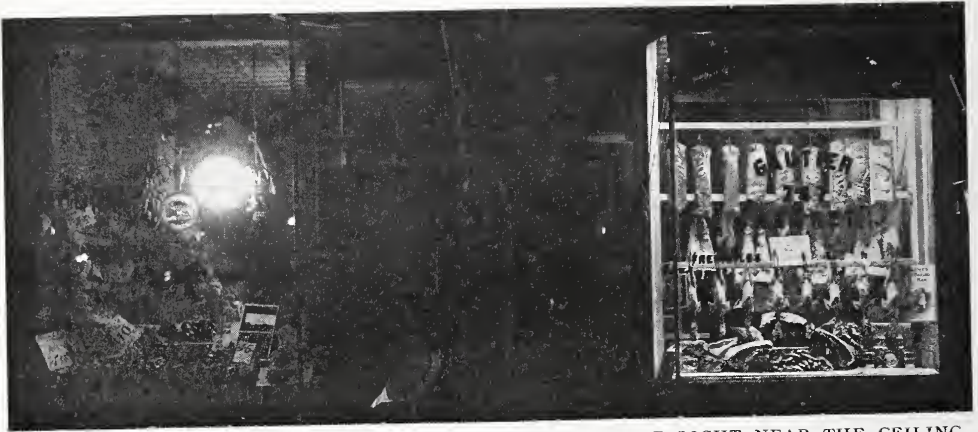
FIG. 1. BY ELIMINATING THE FIXTURE AND PLACING THE LIGHT NEAR THE CEILING THE ILLUMINATION IN THE WINDOW TO THE RIGHT WAS IMPROVED AND THE COST OF LIGHT REDUCED.
