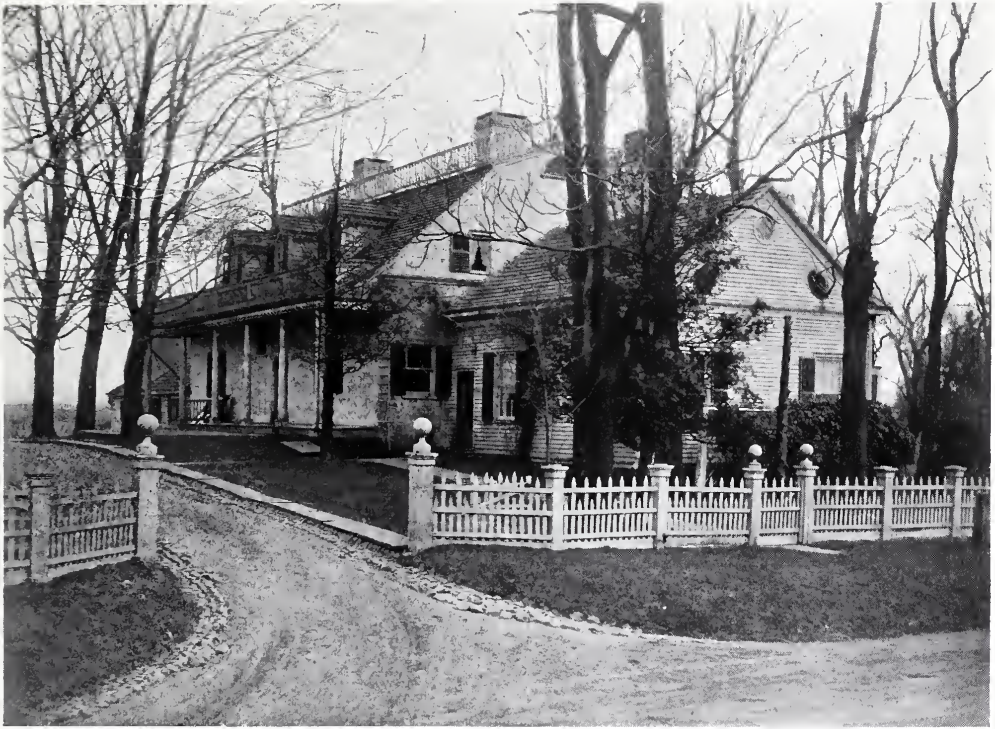
BOARD-ZABRISKIE HOUSE, ON PARAMUS ROAD, NEAR HACKENSACK, N. J. DATED 1790.
