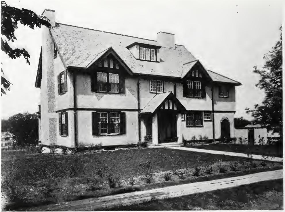
THERE IS AN INTERESTING NOTE IN THE HALF-TIMBER TREATMENT UNDER THE SMALL GABLES AND IN THE LATTICE WORK.
