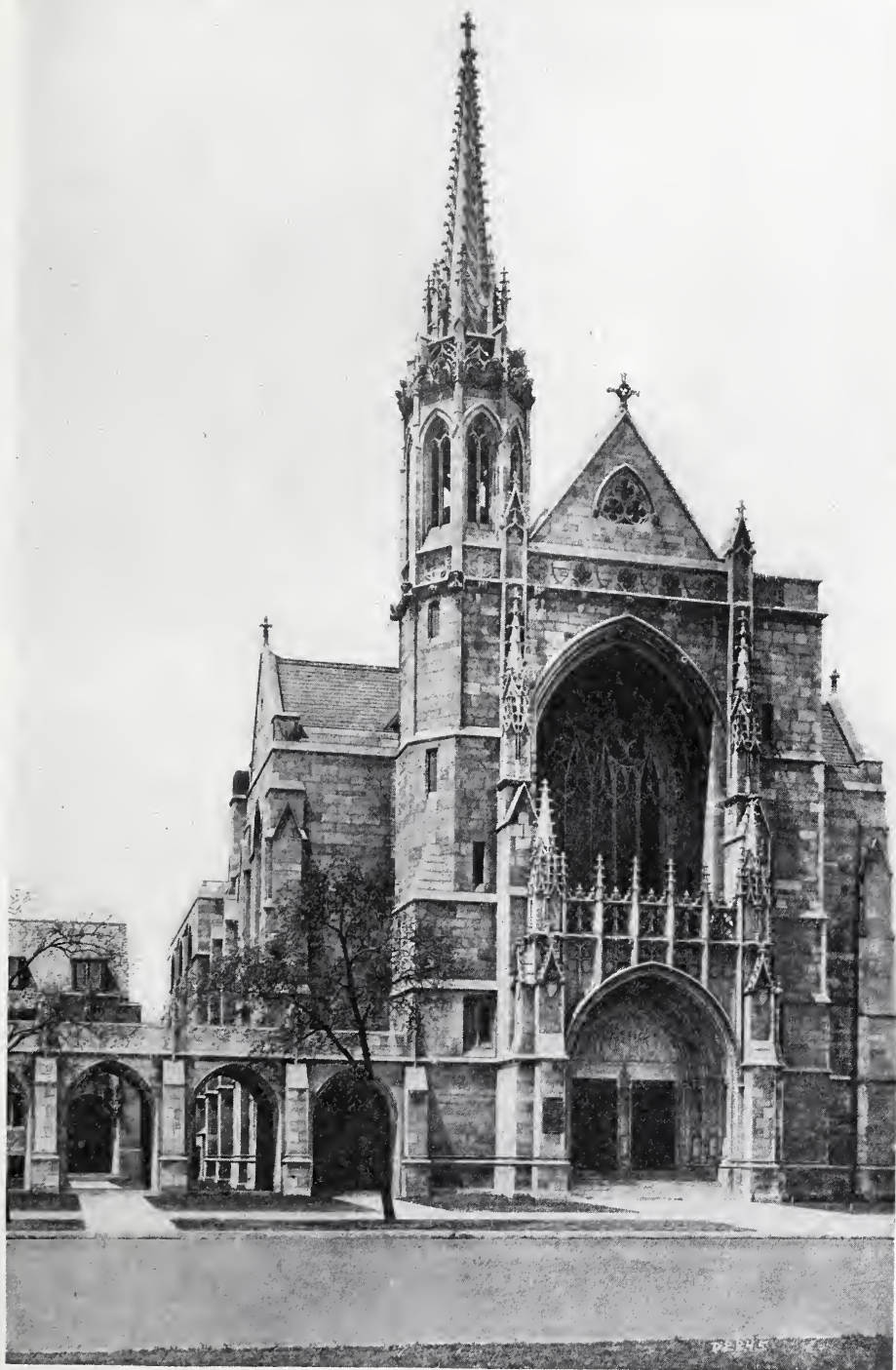
FOURTH PRESBYTERIAN CHURCH OF CHICAGO. CRAM, GOODHUE & FERGUSON, BOSTON, AND HOWARD VAN DORN SHAW, CHICAGO, ASSOCIATE ARCHITECTS.
