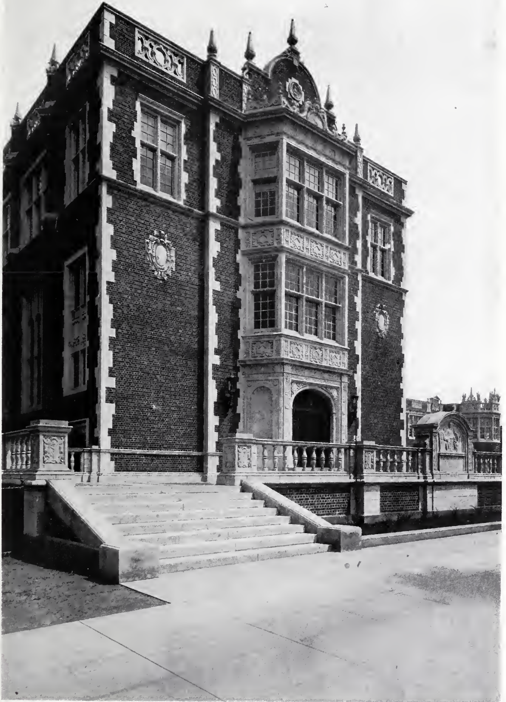
AUDITORIUM BAY—NEWARK NORMAL SCHOOL. E. F. GUILBERT, ARCHITECT.
