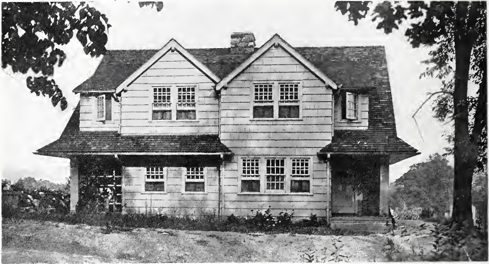
A TWO-FAMILY LABORERS' COTTAGE AT HAYMOUNT, WESTCHESTER COUNTY, N. Y. Arthur T. Remick, Architect.
