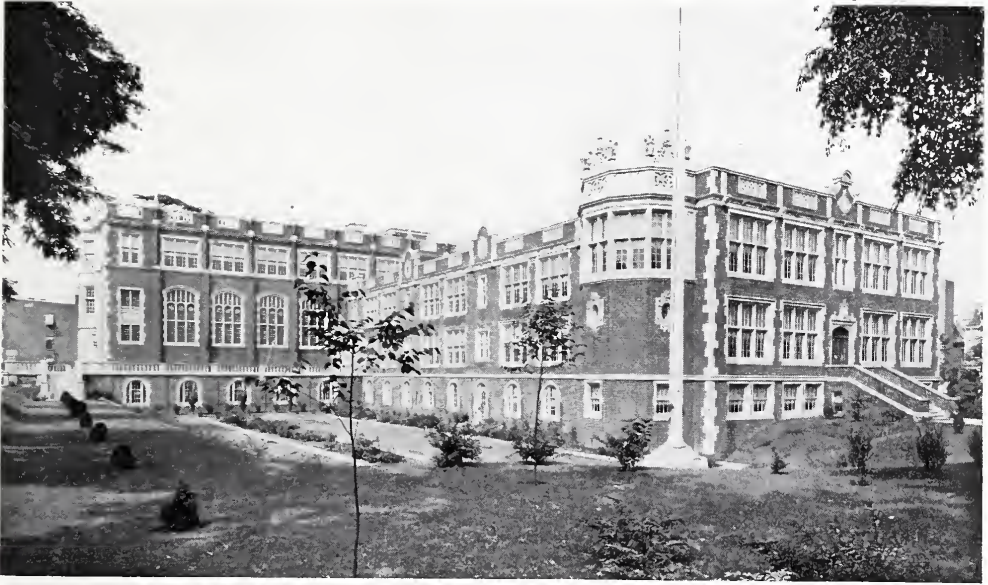
GENERAL VIEW OF THE NEWARK NORMAL SCHOOL. E. F. Guilbert, Architect.
