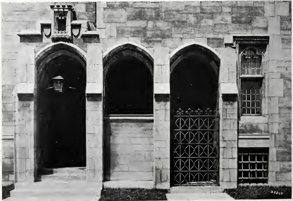
ENTRANCE TO MANSE AND CLUB BUILDING—FOURTH PRESBYTERIAN CHURCH OF CHICAGO. Cram, Goodhue & Ferguson, Boston, and Howard Van Doren Shaw, Chicago, Associate Architects.
