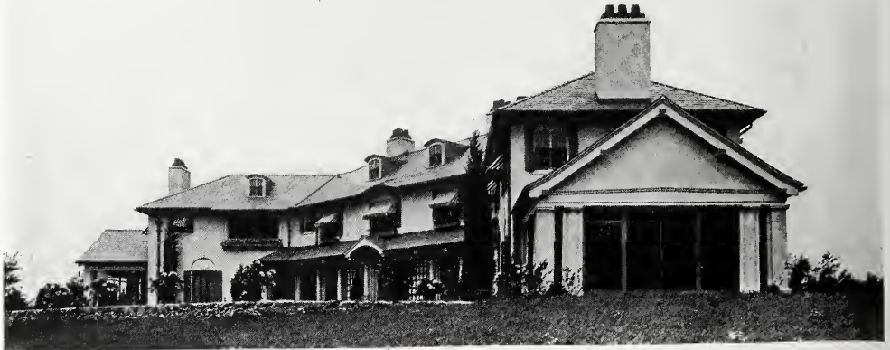
SOUTH VIEW—RESIDENCE OF HARRY L. RICE, ESQ., DOVER, MASS. Kilham & Hopkins, Architects.
