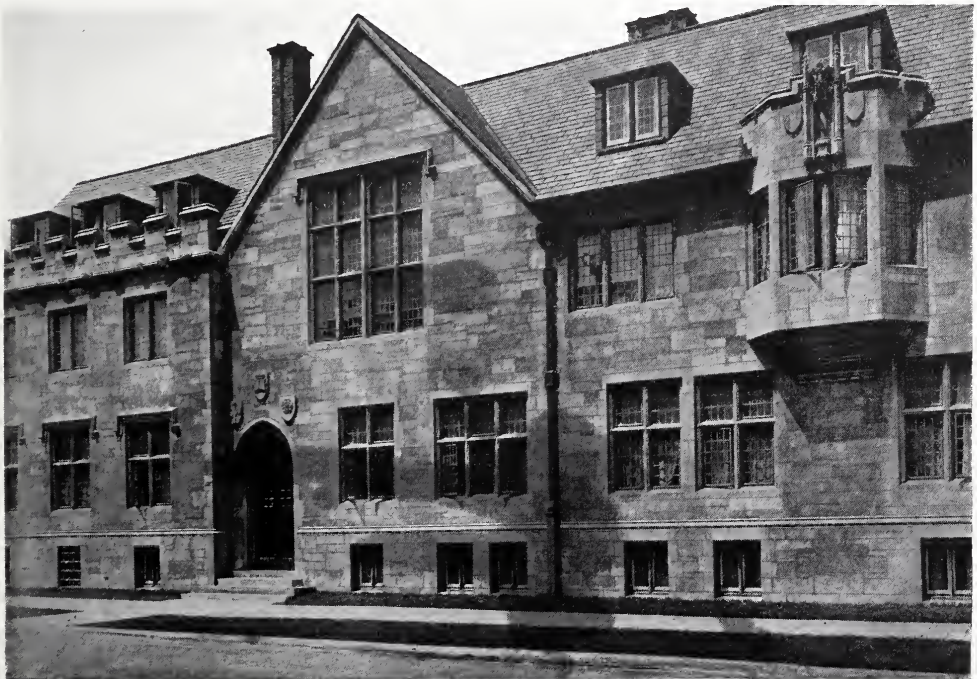
ENTRANCE TO MEN'S CLUB—FOURTH PRESBYTERIAN CHURCH OF CHICAGO. Cram, Goodhue & Ferguson, Boston, and Howard Van Doren Shaw, Chicago, Associate Architects.
