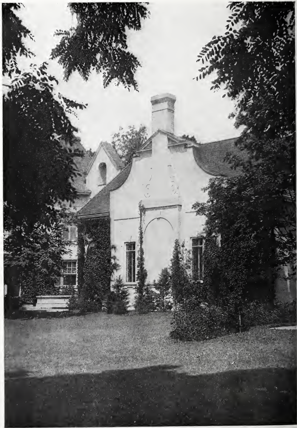
WEST WALL OF THE STUDIO—RESIDENCE OF C. E. PROCTOR, ESQ., GREAT NECK, L. I. LITTLE & BROWNE, ARCHITECTS.
