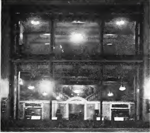
Fig. 2. Lights placed in opal cups leave the merchandise in almost complete darkness.
