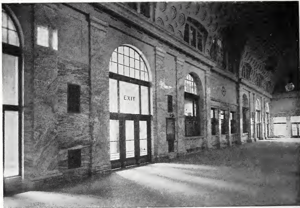
ENTRANCE LOBBY IN UTICA STATION, SHOWING LOCATION OF TICKET OFFICE AT THE DOOR. Fellheimer & Long and Allen H. Stem, Associated, Architects.
