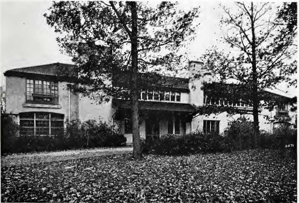
HOUSE OF H. F. MILLER, ESQ., BARRINGTON, ILL. Marshall & Fox, Architects.
