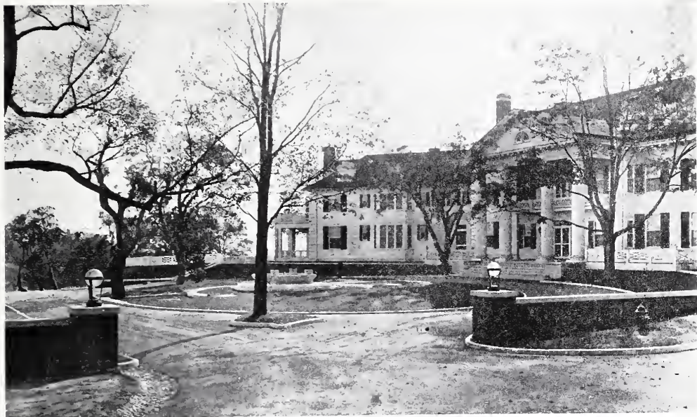
PART OF FRONT ELEVATION OF HAYMOUNT, WESTCHESTER COUNTY, N. Y. Arthur T. Remick, Architect.
