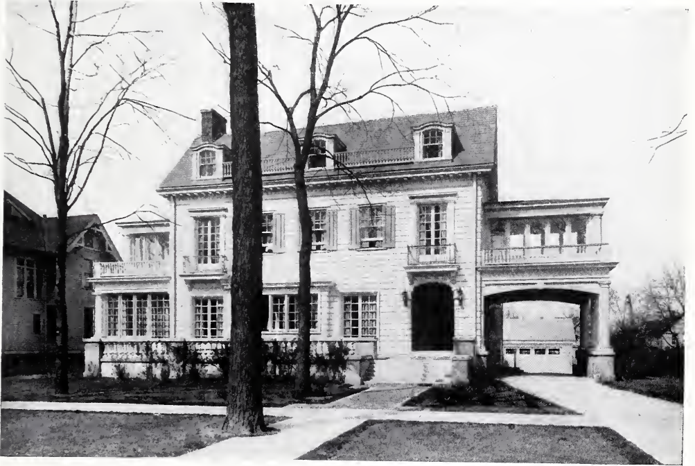
HOUSE OF K. L. AMES, EVANSTON, ILL. Ernest A. Mayo, Architect.
