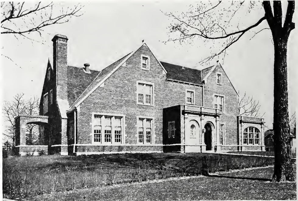
HOUSE OF GEORGE A. MERRYWEATHER, ESQ., HIGHLAND PARK, ILL. Marshall & Fox, Architects.
