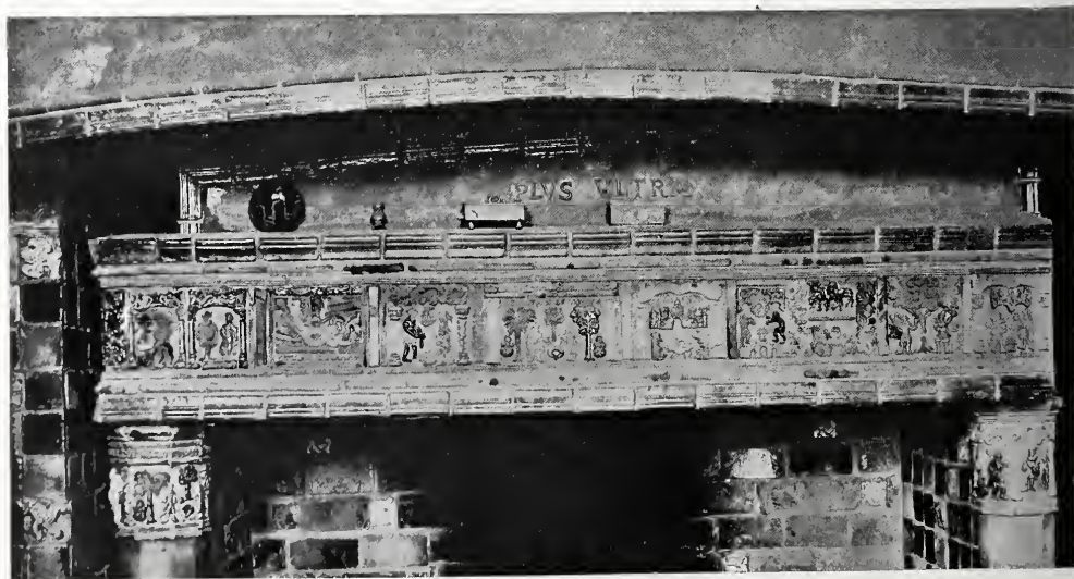
MANTEL OF GLAZED AND UNGLAZED FILIGREE TILE IN CEMENT GROUND. FONTHILL, DOYLESTOWN, BUCKS, PA.
