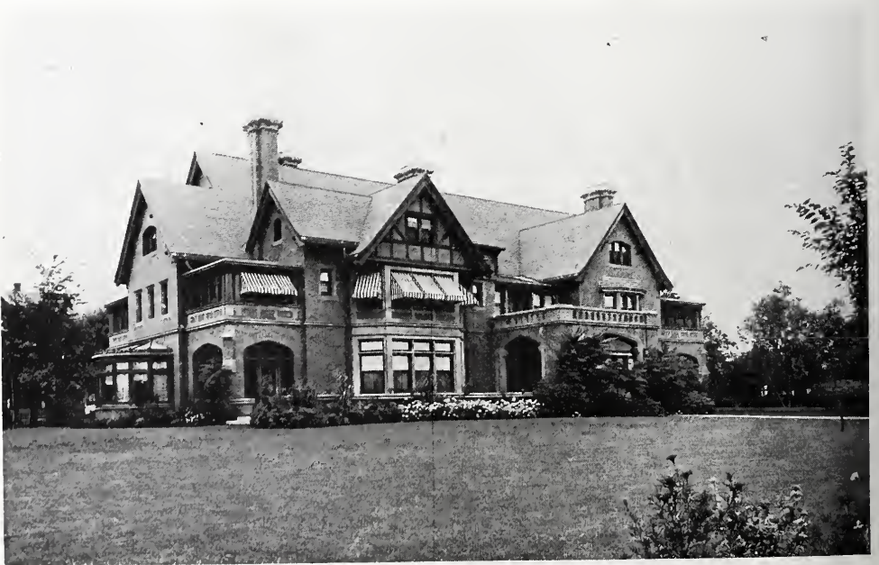
HOUSE OF A. A. SCHLESINGER, ESQ., MILWAUKEE. Fitzhugh Scott, Architect.
