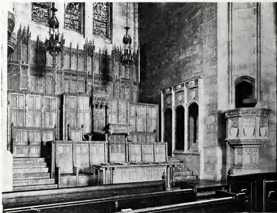
DETAIL OF CHANCEL—FOURTH PRESBYTERIAN CHURCH OF CHICAGO. Cram, Goodhue & Ferguson, Boston, and Howard Van Doren Shaw, Chicago, Associate Architects.
