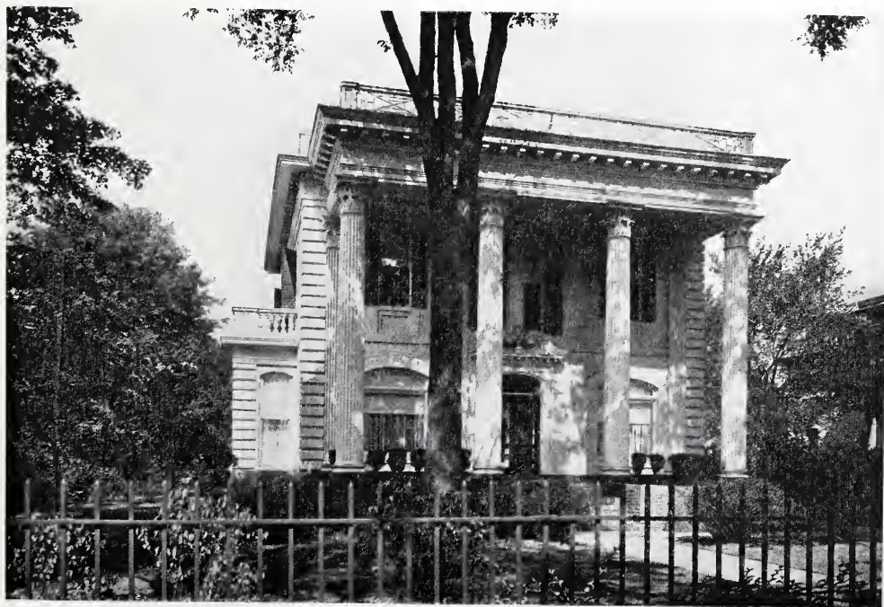
ENTRANCE FRONT—HOUSE OF ELMER MURPHY, ESQ., EVANSTON, ILL. Childs & Smith, Architects.
