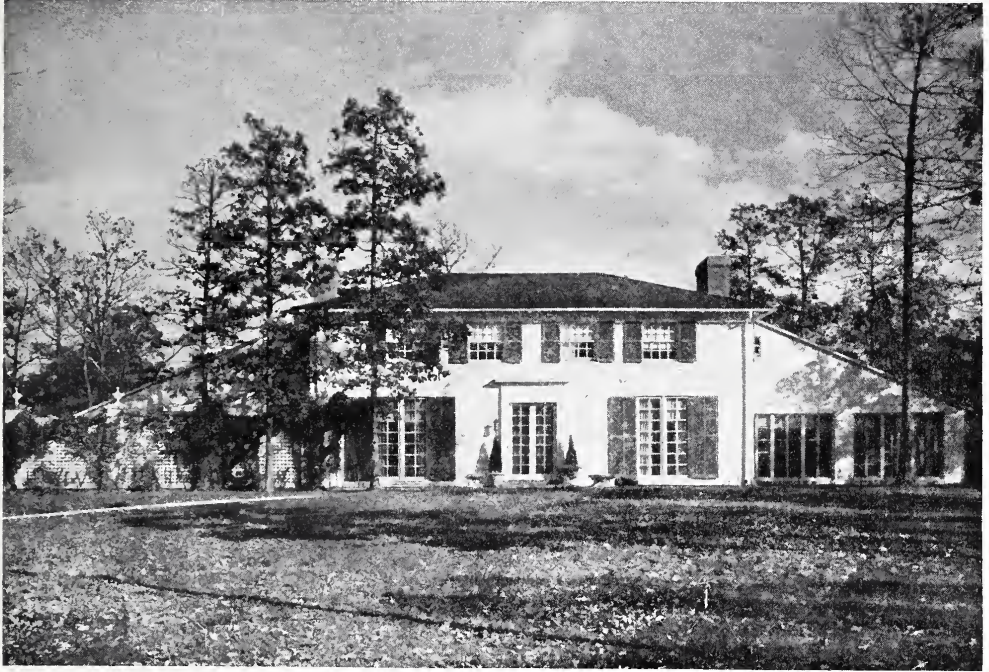
HOUSE OF M. W. KOZMINSKI, ESQ., HIGHLAND PARK, ILL. Robert Seyfarth, Architect.
