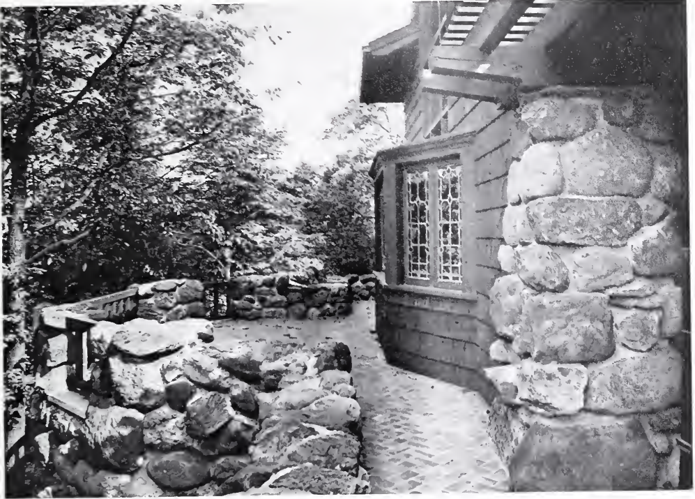
DETAIL OF STONE WORK ON STUDIO AT HAYMOUNT, WESTCHESTER COUNTY, N. Y. Arthur T. Remick, Architect.
