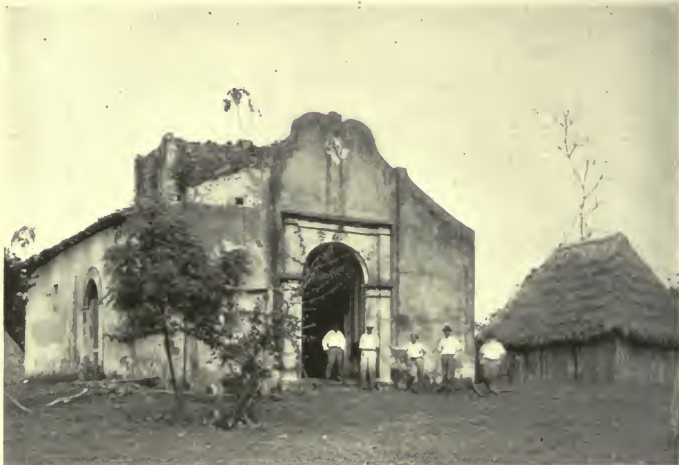
CHURCH AND SCHOOL HOUSE, ARRAJAN, PANAMA.
