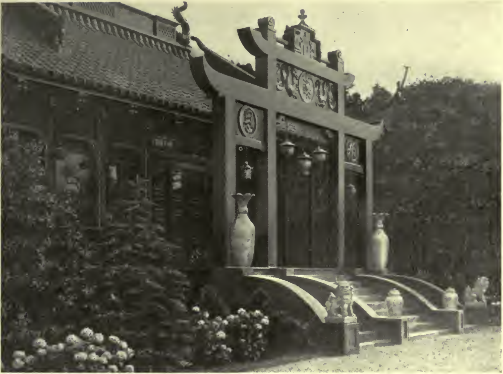
ENTRANCE TO TEA-HOUSE OF MRS. O. H. P. BELMONT, NEWPORT, R. I. Hunt & Hunt, Architects.
