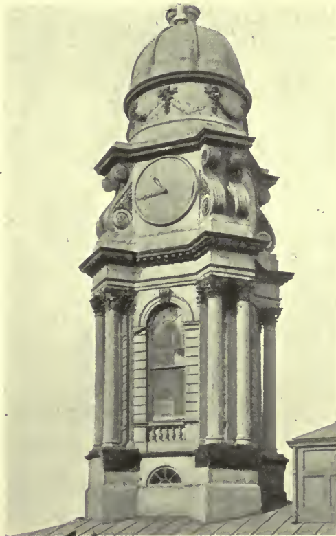
THE CUPOLA, AS REBUILT AFTER THE FIRE OF 1858.
