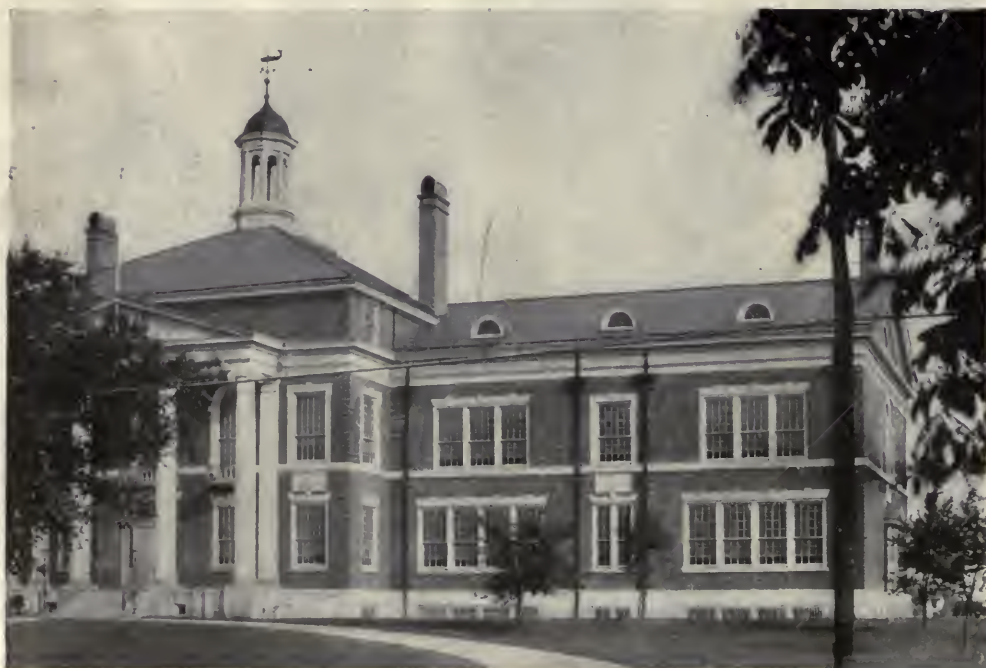
WEST WING—HIGH SCHOOL, SOUTHAMPTON, L. I. William Lawrence Bottomley, Architect.
