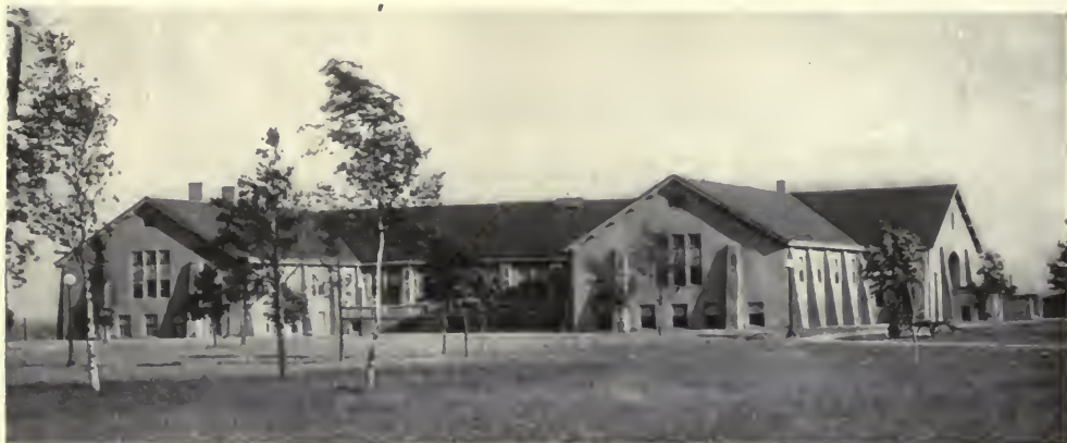
CLUB BUILDING, MORGAN PARK, DULUTH, MINN. Dean & Dean, Architects.
