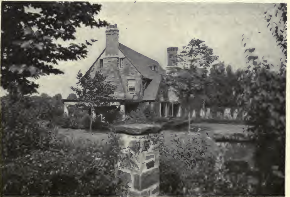
FRONT VIEW—HOUSE AT CYNWYD, PA. Mellor & Meigs, Architects.
