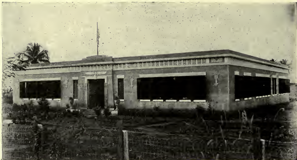
SCHOOLHOUSE FOR CONSOLIDATED RURAL SCHOOLS, BARRIO SANTANA, ARECIBO, P. R.
