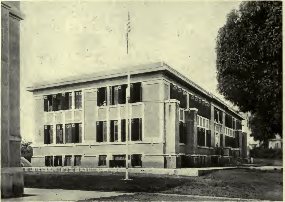
HIGH SCHOOL IN MAYAGUEZ, P. R., OF REINFORCED CONCRETE CONSTRUCTION. IT SURVIVED UNINJURED THE EARTHQUAKE OF 1918, WHICH DESTROYED NEARLY THE WHOLE OF THE CITY.
