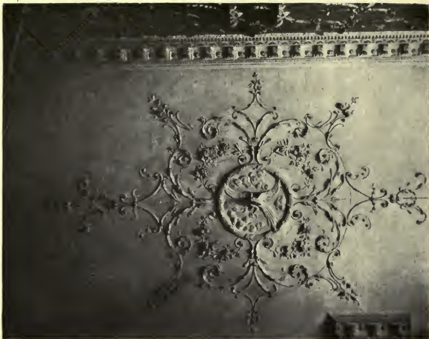
STAIRCASE CEILING—BEACON HOUSE, PAINSWICK, GLOUCESTER.
