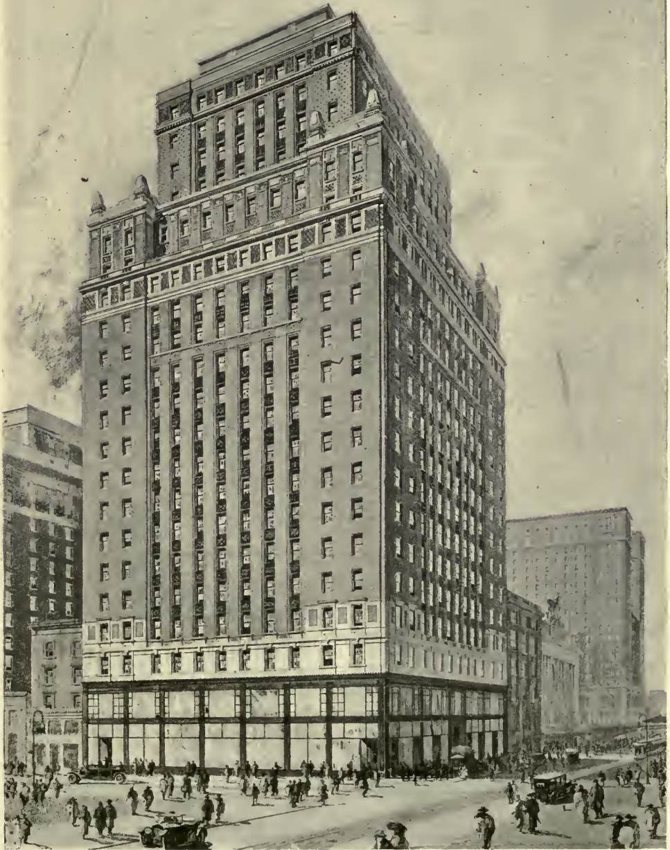
LIGGETT-WINCHESTER-LEY CORPORATION BUILDING, NEW YORK CITY. CARRERE & HASTINGS, AND R. H. SHREVE, CONSULTING ARCHITECTS.
