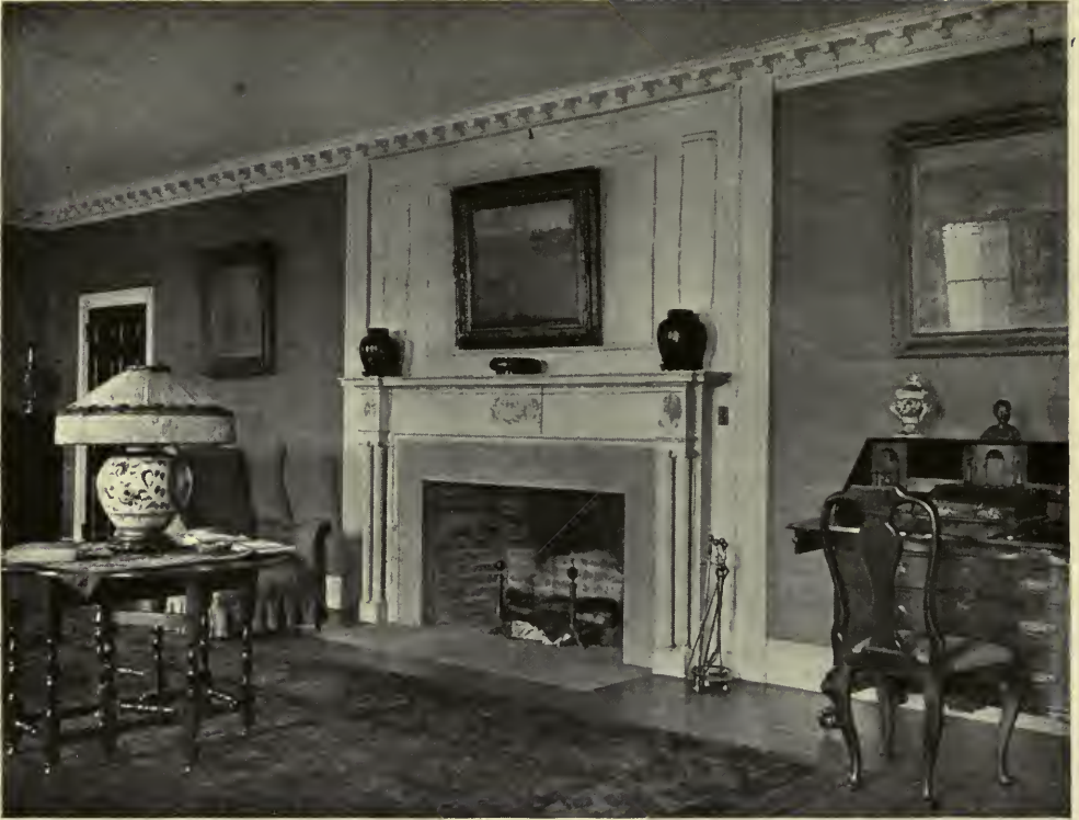
LIVING ROOM—HOUSE AT LLOYD'S NECK, L. I. Murphy & Dana, Architects.
