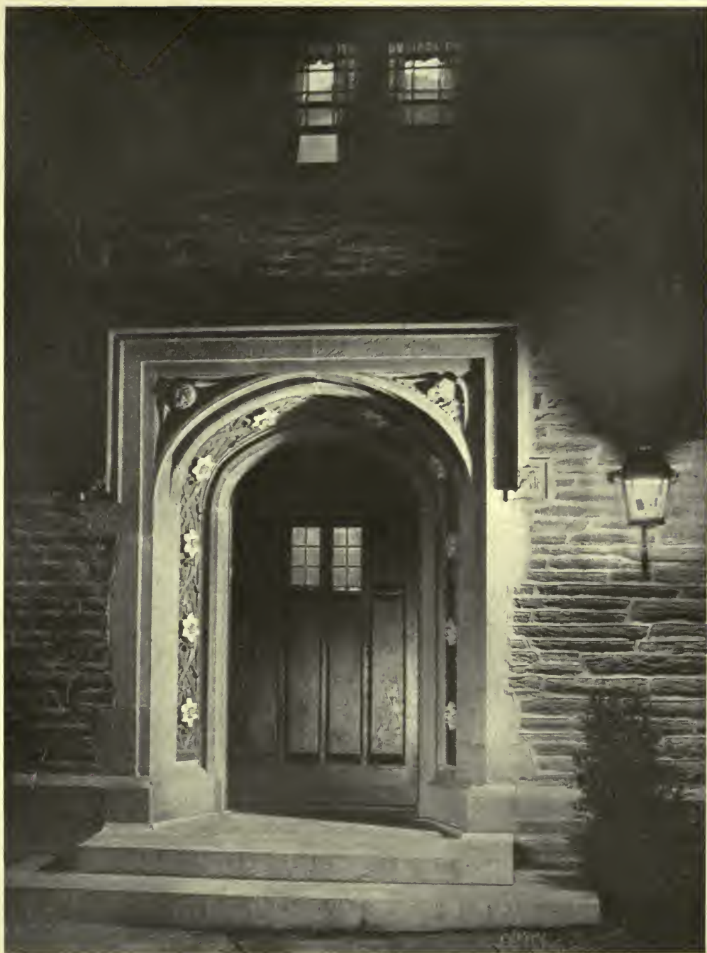
NIGHT VIEW OF FRONT DOOR OF NARCISSUS COTTAGE, SHOWING EFFECT OF INDIRECT LIGHT IN DOORWAYS, EAVES, GABLES, ETC. THERE ARE NO STREET LAMPS ON THE COLLEGE GROUNDS.
