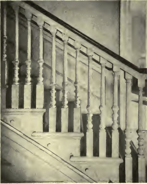
DETAIL OF STAIR BALUSTRADE, CLIVEDEN, GERMANTOWN (1763).
