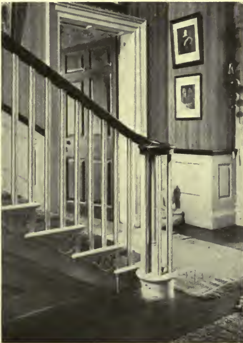
DETAIL OF STAIR BALUSTRADE, UPSALA, GERMANTOWN (1798)
