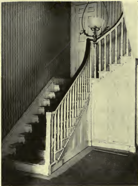
STAIRWAY, MACLAY MANSION, HARRISBURG (1790) Example of "Open Newelled Stairs."
