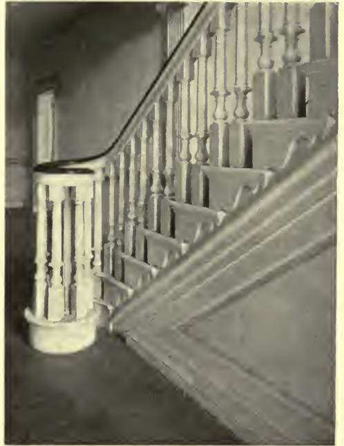
STAIRWAY AT WHITBY HALL, PHILADELPHIA (1754).
