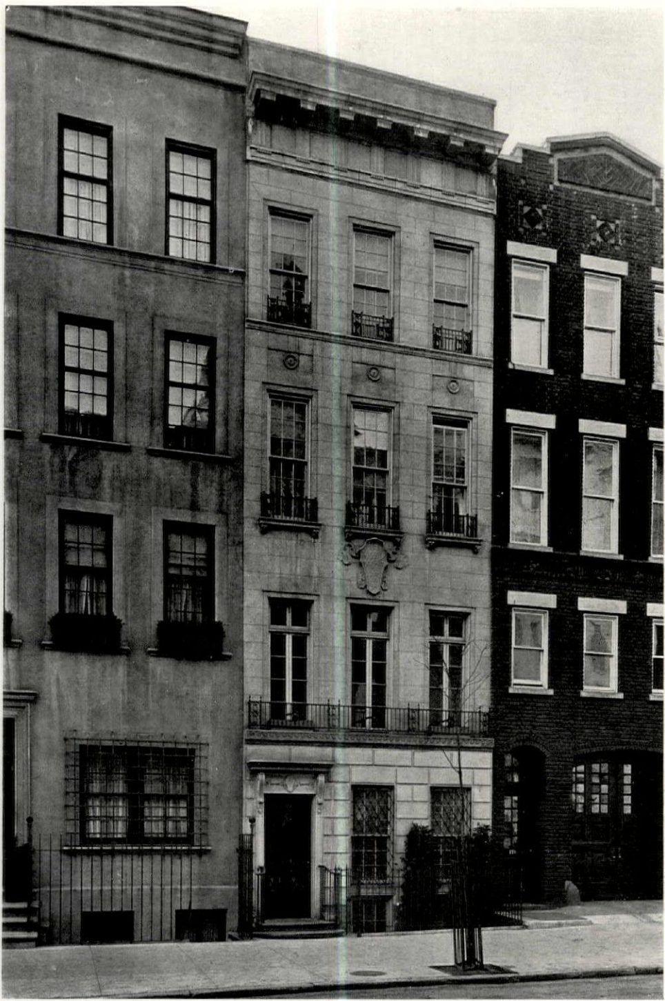
GENERAL ELEVATION—RESIDENCE ON 75TH STREET, NEW YORK CITY. HARRY M. CLAWSON, ARCHITECT.
