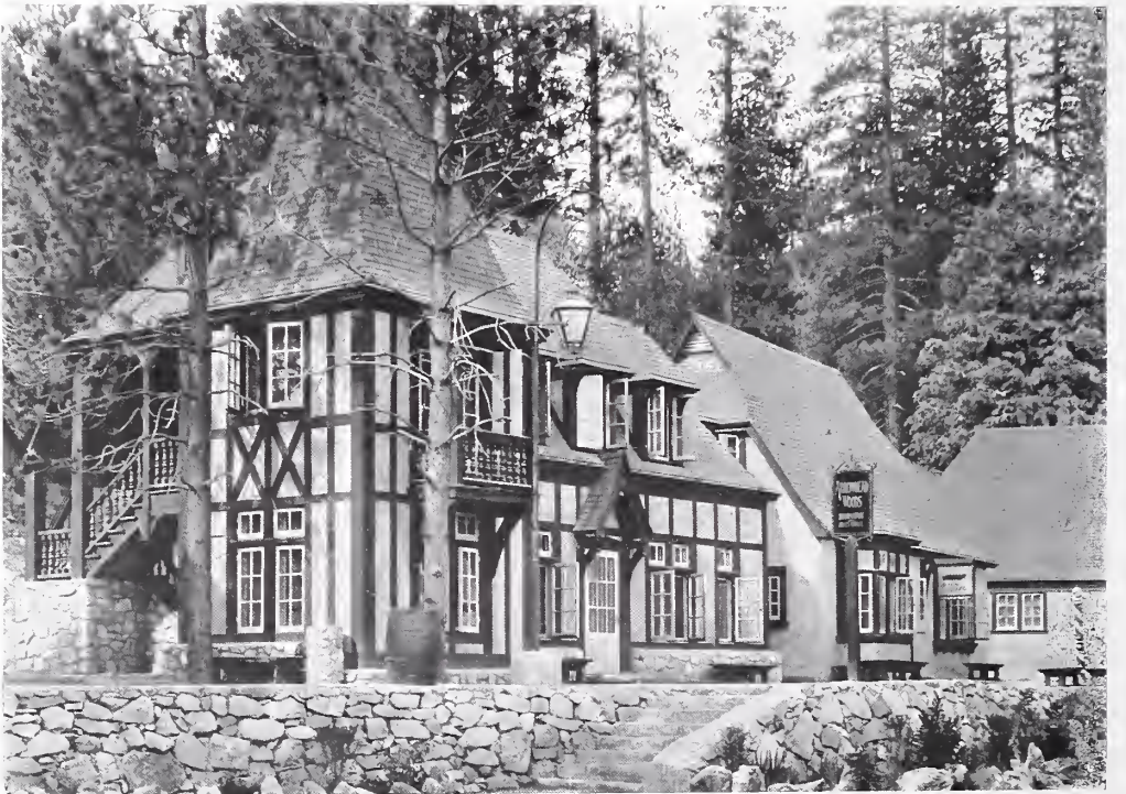
Real Estate Office and Barber Shop ARROWHEAD LAKE, CALIFORNIA McNeal Swasey, Architect. H. C. McAfee, Associate
