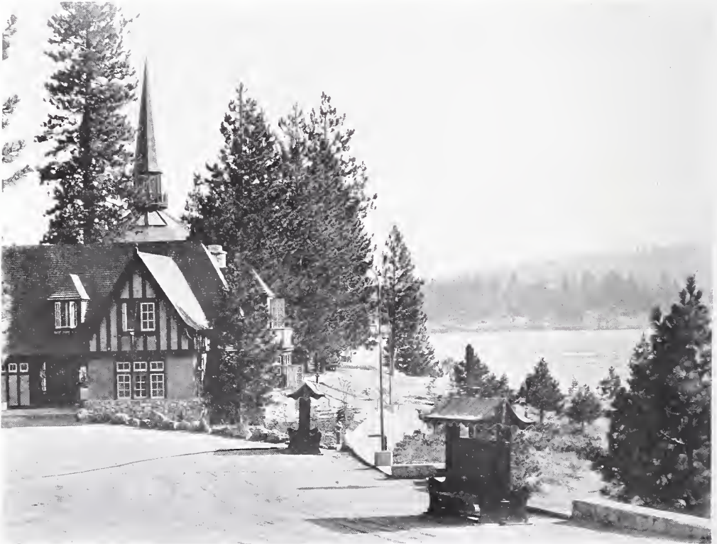
Art Store ARROWHEAD LAKE, CALIFORNIA McNeal Swasey, Architect. H. C. McAfee, Associate
