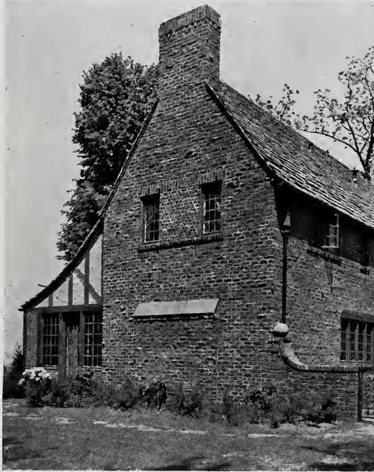
End Elevation RESIDENCE OF W. JULE DAY, ESQ., DOUGLASTON, LONG ISLAND Frank J. Forster, Architect
