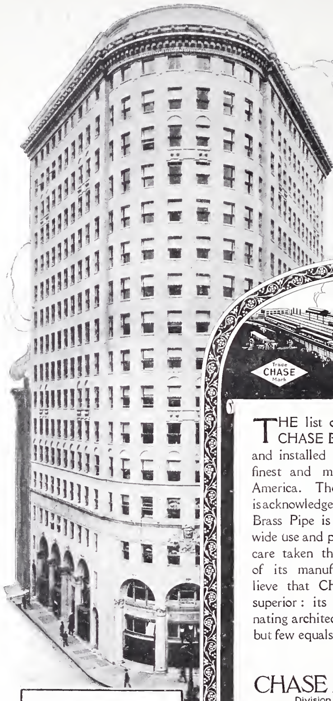
Turk's Head Building, Providence, R. I. John Mead Howells, architect. Equipped with CHASE Brass Pipe.
