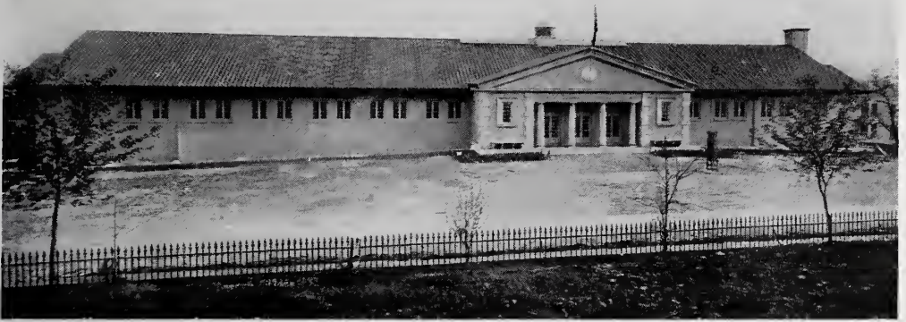
THE U. S. FREE BATH HOUSE, HOT SPRINGS NATIONAL PARK, ARKANSAS Mann & Stern, Architects
