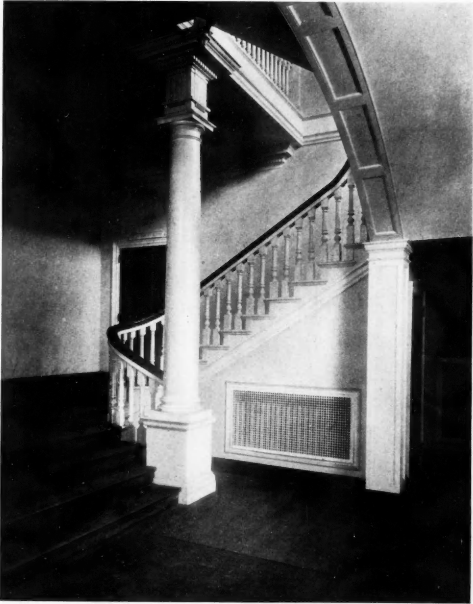
Stair Hall THE TOWN HOUSE, PETERBOROUGH, NEW HAMPSHIRE Little & Russell, Architects
