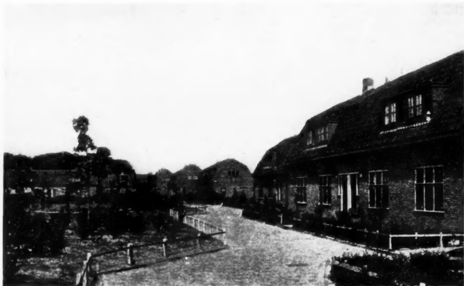
Fig. 44—Cottage Type of Municipal Housing GARDEN CITY SUBURB OF OOSTZAAN, AMSTERDAM, HOLLAND
