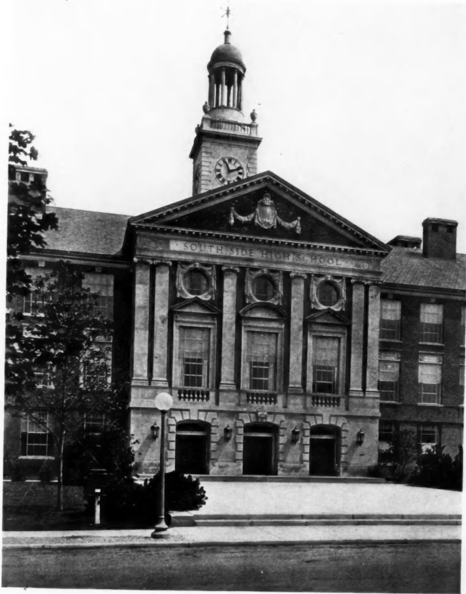
Entrance Detail SOUTH SIDE HIGH SCHOOL, ROCKVILLE CENTRE, NEW YORK Huse Templeton Blanchard, Architect
