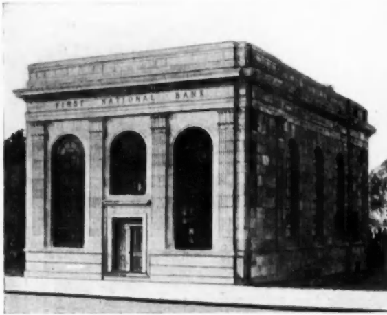
First National Bank, Perkasie, Pa. Tilghman Moyer Co., Architects.
