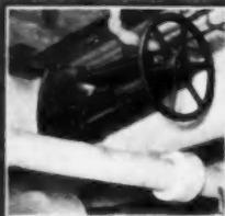
10-inch Jenkins Standard Fire Line Valve. Range, with rising spindle installed in the main street line.
