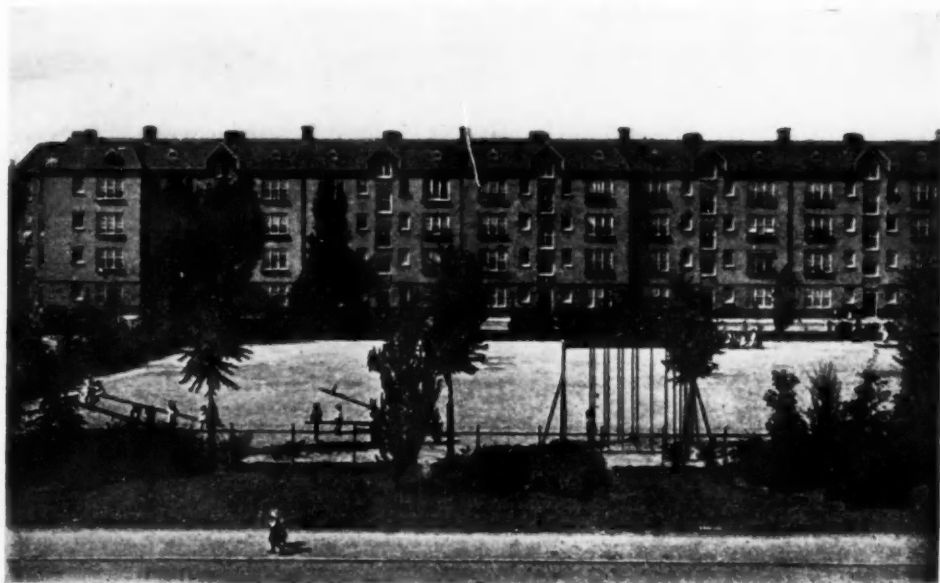
Fig. 46—Façade on Playground APARTMENT BUILDING OF MUNICIPAL HOUSING DEPARTMENT, AMSTERDAM, HOLLAND
