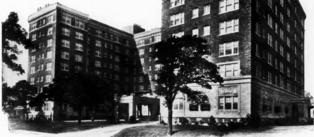
MELROSE COURT, Dallas, Tex. Architects—C. D. Hill & Co., Dallas. Plaster Contr.—Walter Williamson, Dallas. Solid 2" partitions of KNO-BURN Metal Lath thruout. LONGSPAN Metal Lath used for ceilings under steel floor tile.
