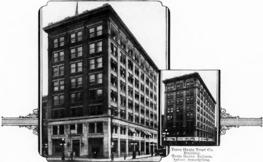
Terre Haute Trust Co. Building, Terre Haute, Indiana, Remodelled. Weary & Alford, Architects.
