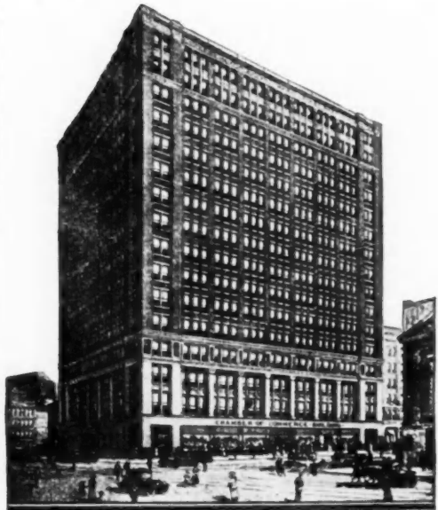
Chamber of Commerce Building, Pittsburgh, Penna. Architect—E. B. Lee, Chamber of Commerce Bldg., Pittsburgh
