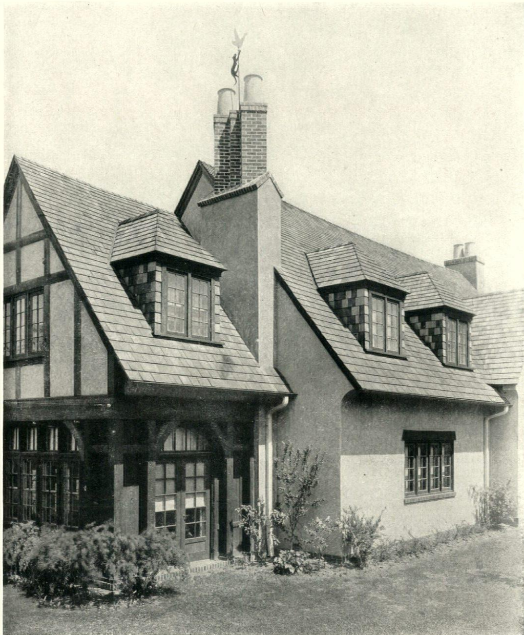
WEST HOUSE, KANSAS CITY, MISSOURI Edward Buehler Delk, Architect
