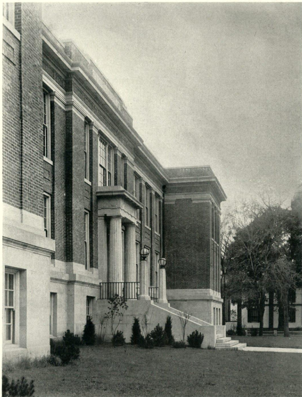
Entrance Detail NORTH JUNIOR HIGH SCHOOL, WALTHAM, MASSACHUSETTS Charles G. Loring, Architect
