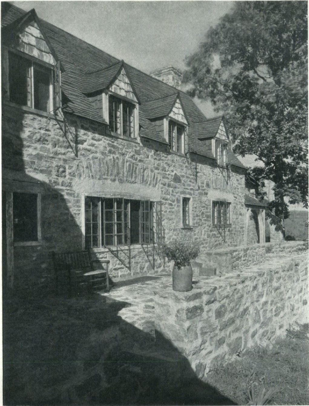
RESIDENCE OF WALDO SHELDON, ESQ., WILSON POINT, SOUTH NORWALK, CONN. Frank J. Forster, Architect
