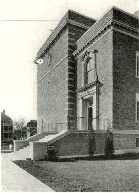
Entrance Detail HIGH SCHOOL, NORWOOD, MASS. Ritchie, Parsons & Taylor, Architects
