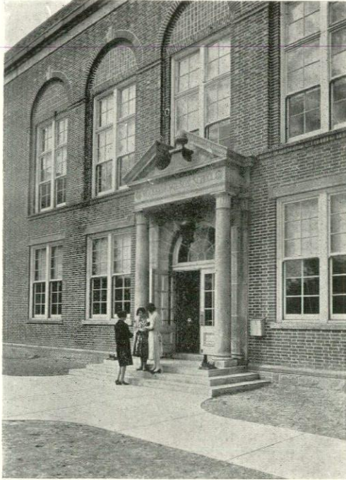
Entrance Detail HIGH SCHOOL, BECKLEY, WEST VIRGINIA Wm. B. Ittner, Architect
