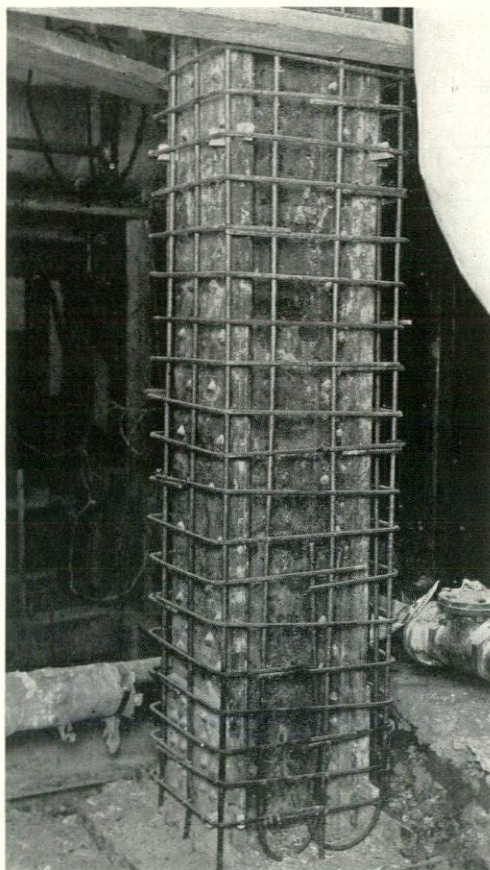
Reinforcing a Column
