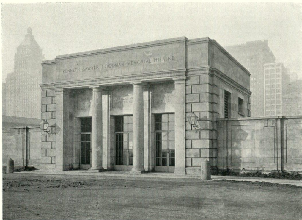
Main Entrance KENNETH SAWYER GOODMAN MEMORIAL THEATRE, CHICAGO Howard Van Doren Shaw, Architect
