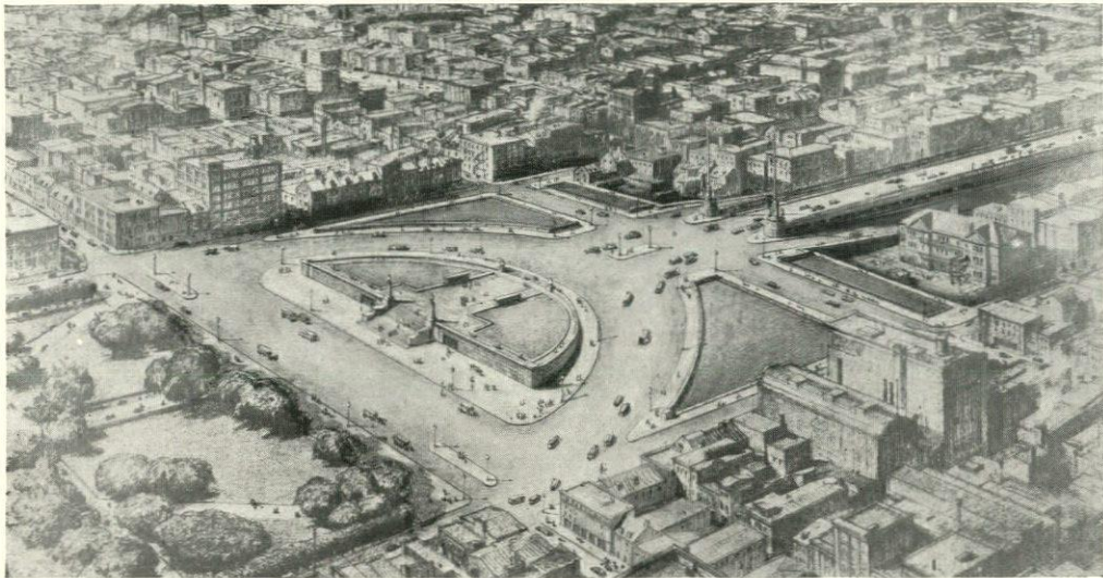
PLAZA AT WEST APPROACH—DELAWARE RIVER BRIDGE Paul P. Cret, Architect. Ralph Modjeski, Engineer
