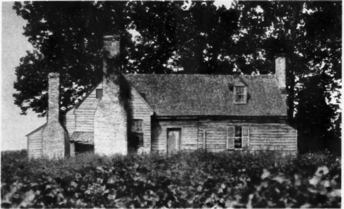
HOUSE NEAR PETERSBURG, VA. INFORMAL CHIMNEY GROUPING
