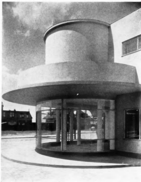
DETAIL, WORKMEN'S DWELLINGS WITH SHOPS, HOOK OF HOLLAND J. J. P. OUD, ARCHITECT
