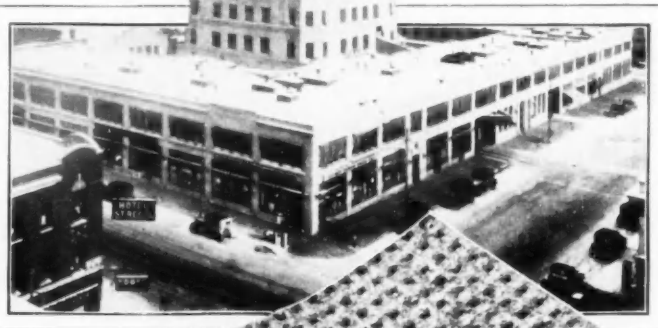
Architects and Engineers Magney & Tusler, Inc. Contractors—National Con- tracting Co. and Maurice Schumacher. Roofers—Krukeberg Roof- ing and Cornice Works. All of Minneapolis.
