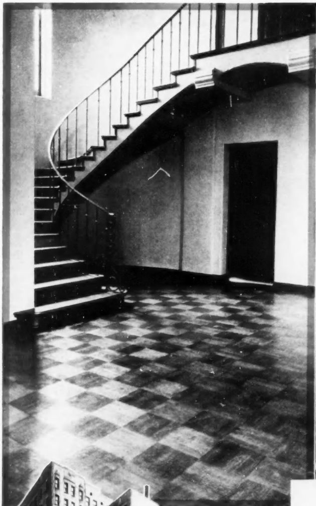
222 E. Chestnut St. Rissman & Hirschfeld, Architects Trimmer-Nydele Co., Contractors 100,000 sq. ft.—9" and 11 1/4" blocks
