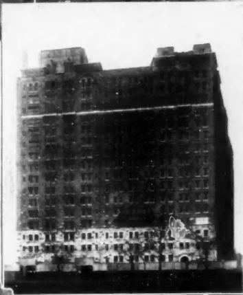
3260-70 Sheridan Road Hooper & Janisch, Architects Reliance Co., Inc., Contractors 100,000 sq. ft.—6 1/2", 9", 11 1/4" blocks
