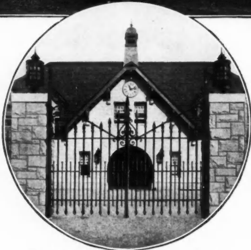
ENTRANCE GATE—STABLES OF WM. ZIEGLER, JR.
