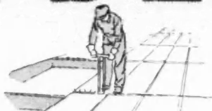
Tying the reinforcement
