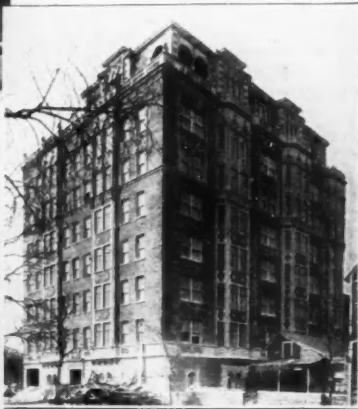
Albert O'Rourke Apts, 76th and South Shore Drive Leichenko & Esser, Architects 30,000 sq. ft.—6 1/2" and 9" blocks
