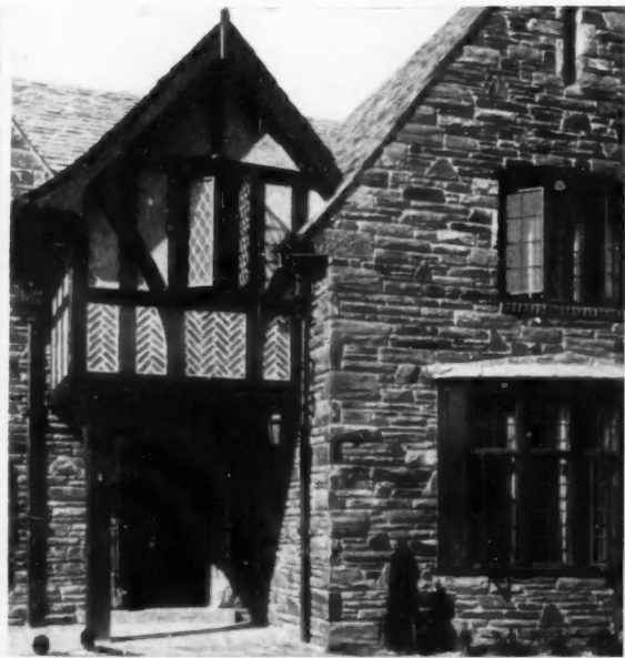
Residence of L. M. Seiver, Drexel Park, Pa. William J. Carlson, Builder
