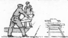
Laying a Gypsteel slab
