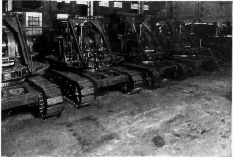
Abrasive wear from heavy equipment or loaded trucks is at best a severe test. Failure starts at spots where oil drippings have been absorbed and the concrete weakened by the consequent disintegration.
