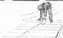
Grouting the joints between slabs
