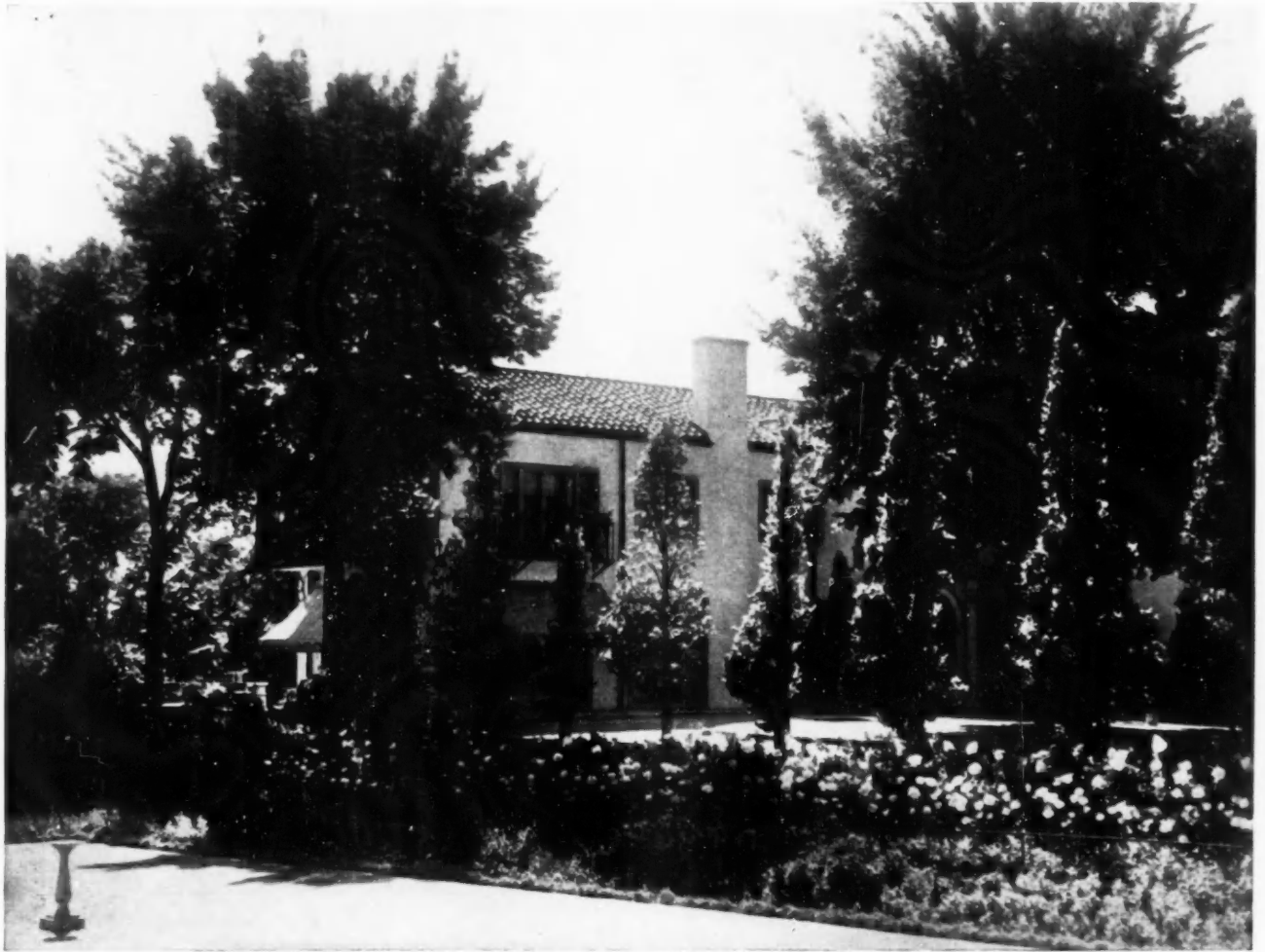
Reproduction from a color photograph of El Contento , the estate of Warren Wright, Golf, Illinois, by Wilfred O. Flotig © The D. T. E. Co., Inc., 1929
