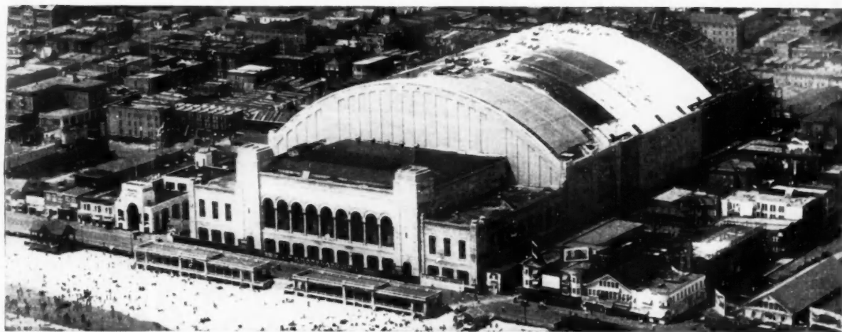
The Convention Hall at Atlantic City has a roof area of 220,000 square feet. The roof deck is of Gypsteel Pre-Cast Gypsum Slabs. Lockwood, Green & Co., Engineers
