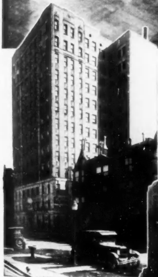
73 E. Elm St. M. Nally & Quinn, Architects 50,000 sq. ft.—6 1/2" and 9" blocks
