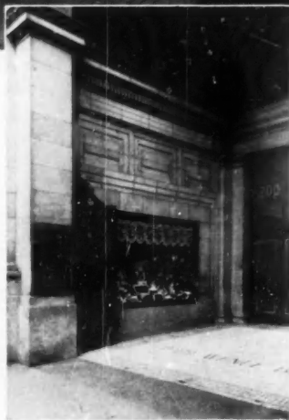
Fifth Avenue Building, New York City. Architect, Maynicke & Fanke. Contractor, Hadden Construction Co. These unretouched photographs of a 21 year old building forcibly demonstrate the non-staining qualities of our product
