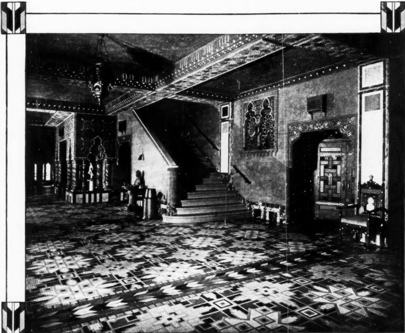
A dramatic use of Ceramic Tiles in the lobby of the Avalon Theatre, Chicago. Ceramic mosaic and faience tiles were used to create the strikingly effective floor. John Ebersson, Architect.
