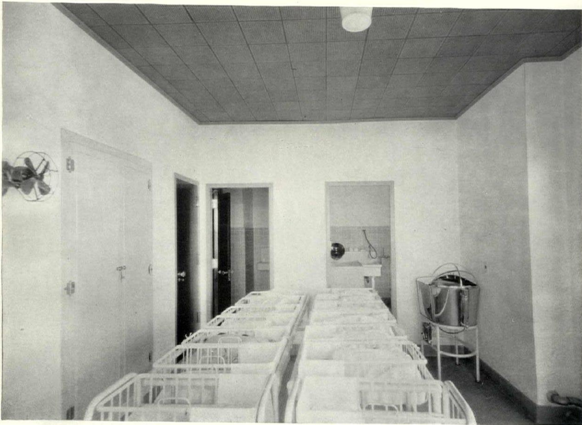
NURSERY WITH ACOUSTI-CELOTEX CEILING ST. JOHN'S HOSPITAL, TULSA, OKLA. WIGHT & WIGHT, ARCHITECTS
