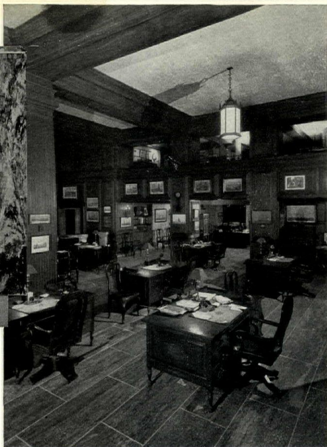
General Offices, State Street Trust Company, Boston. Large rectangles of cream and red grainings against a black field, with inner lines of cream. This floor expresses the feeling of stability achieved by the massive beams and columns, and the wide panelling.
