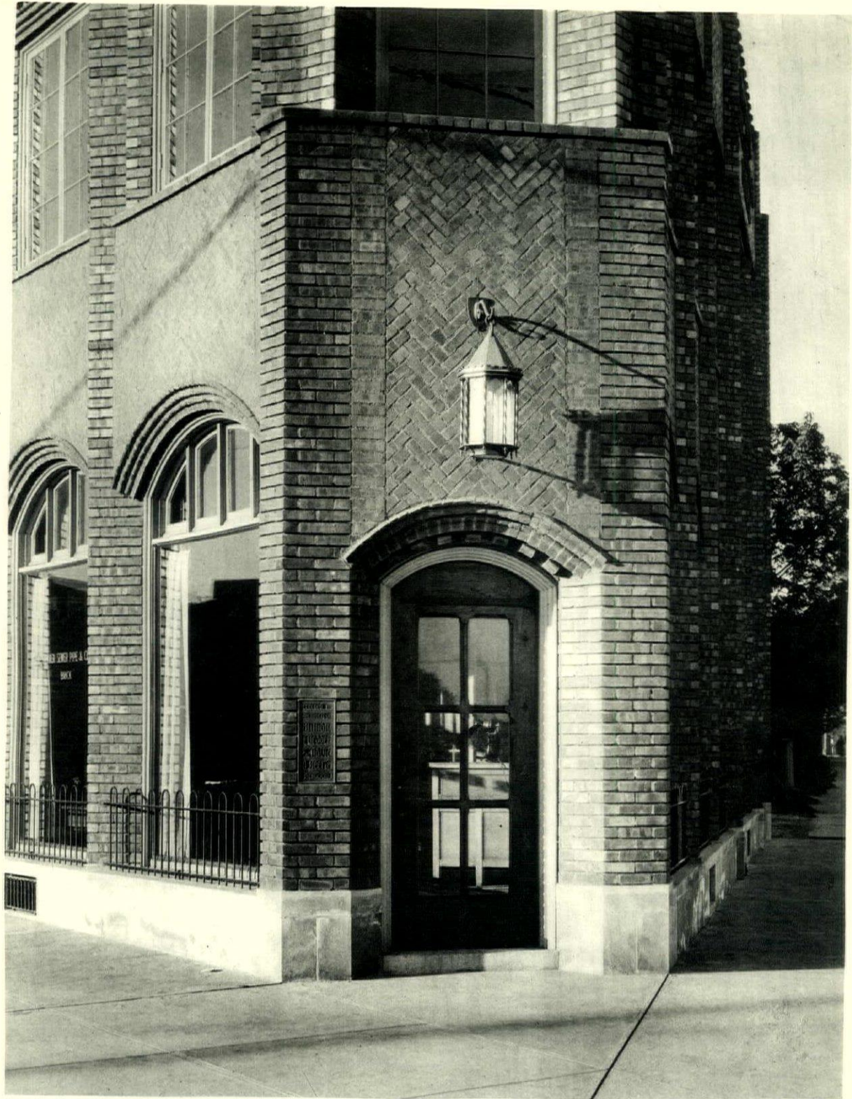
Entrance to Display Room The Denver Sewer Pipe and Clay Co. Building M. H. AND B. HOYT, ARCHITECTS
