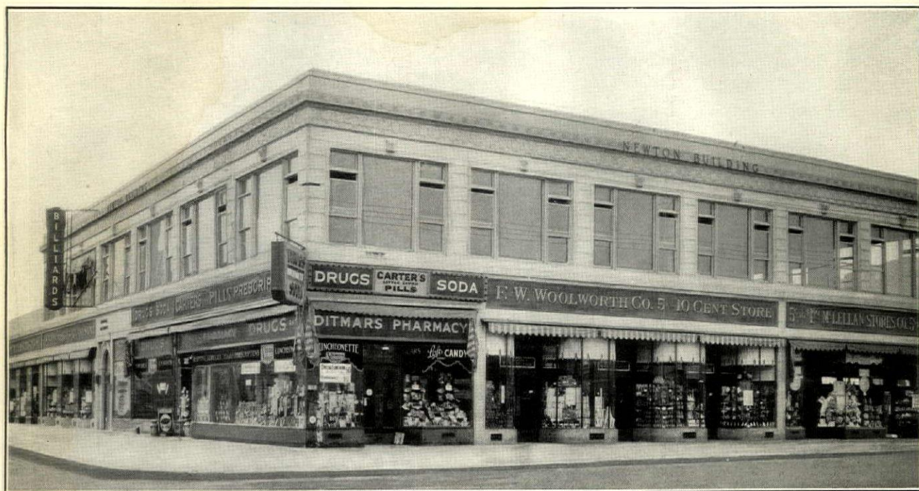
Newton Building—New York, N. Y. Desco Store Fronts are achieving growing popularity for chain stores. The Newton Building is an interesting example.
