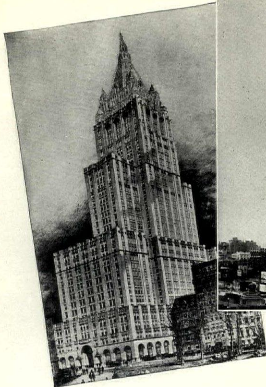
New York Life Insurance Building New York, N. Y. Cass Gilbert, Architect Starrett Bros., Inc., General Contractors
