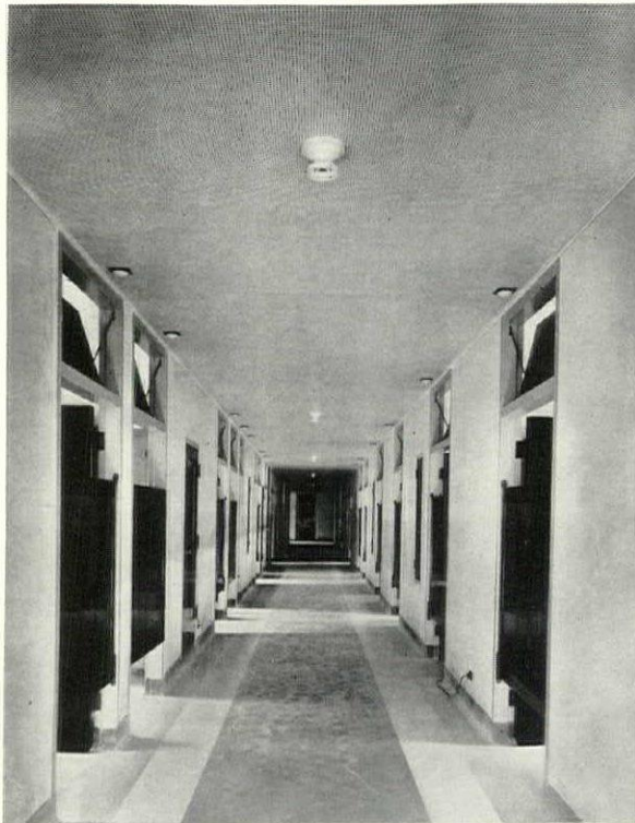
CORRIDOR CEILING OF NASHKOTE B
