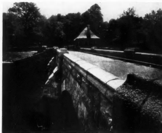
BRIDGE ON J. P. MORGAN ESTATE GLEN COVE, LONG ISLAND CHARLES W. LEAVITT & SON, LANDSCAPE ARCHITECTS
