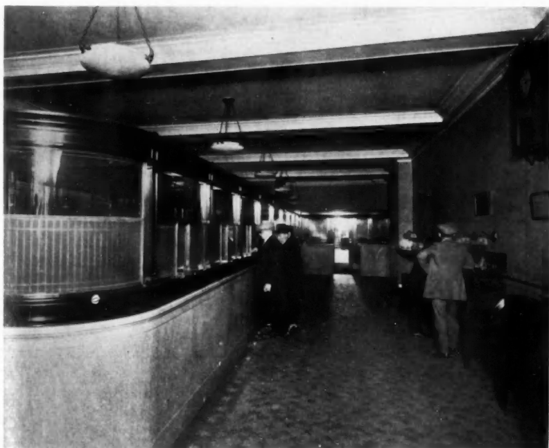
VIEW BEFORE REMODELING
