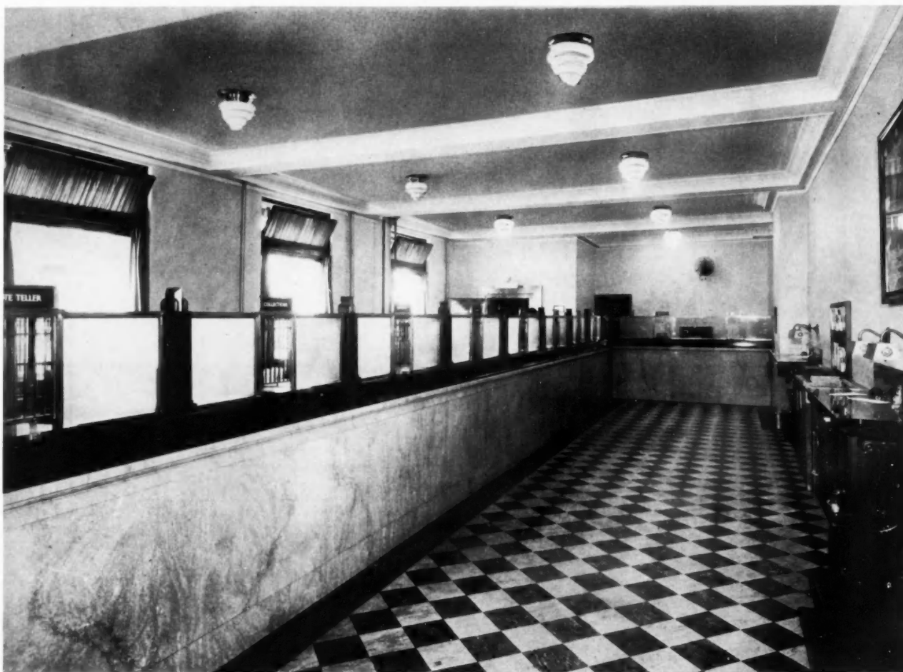
INTERIOR OF BANK AFTER REMODELING
