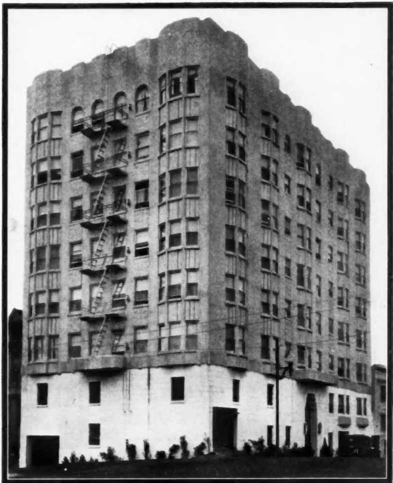
The Epp Apartments, San Francisco, California. Architect, H. C. Bowman, Electrical Contractor, David Grandi, Steeltubes supplied by the Westinghouse Electric Supply Co.
