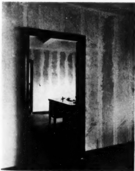
GYPSUM PLANK (GYPSTEEL), 2" in thickness, as interior partition. This wall can be painted without other finish. Adapted to exterior construction when protected.
