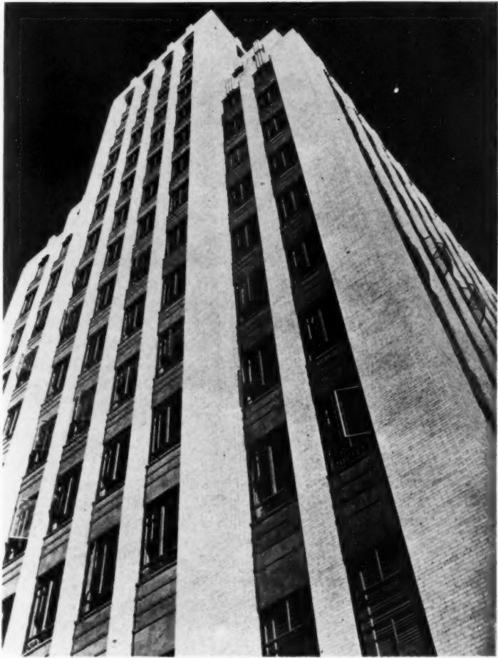
Detail of Exterior.
