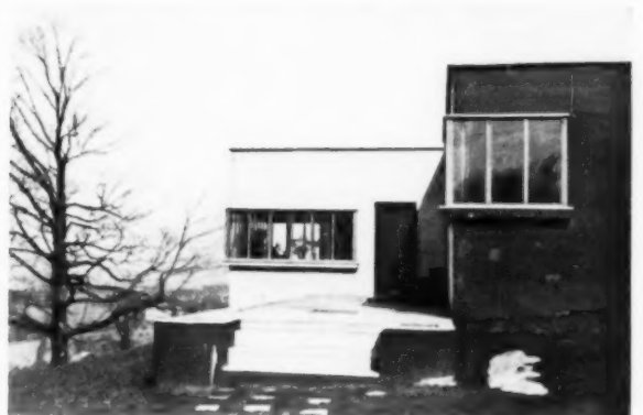
HOUSE OF REX STOUT in Connecticut near Brewster, New York. By A. Lawrence Kocher and Gerhard Ziegler, 1929. Exterior walls double, each 3" concrete poured in Van Guilder forms. There is a 2" air space. Aluminum window sills.
