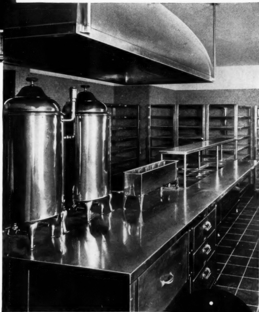
● View in one of the Patients Kitchens in the main hospital building showing Monel Metal equipment made and installed by THE ARKAY COMPANY, New York, N. Y. This equipment includes refrigerator cabinet, food trucks, Thermotainer roll warmer, steam table, coffee urns and urn stand.
