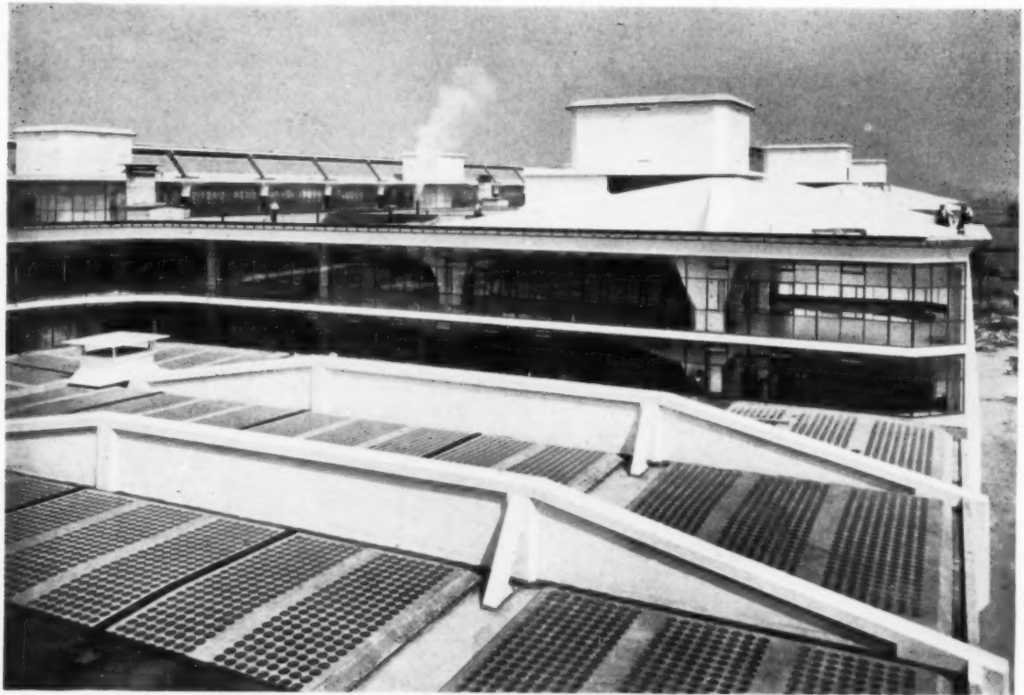
General view of roofs, showing cantilever beams over unloading docks.
