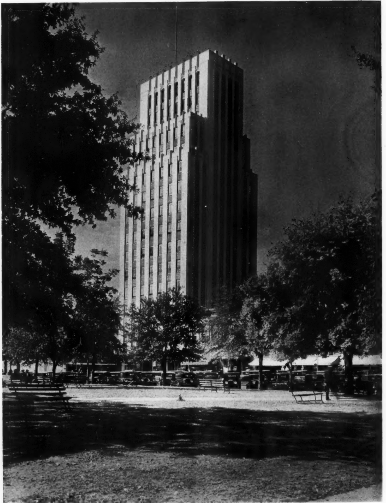
View from the Square. Building is 15 stories and basement in height.
