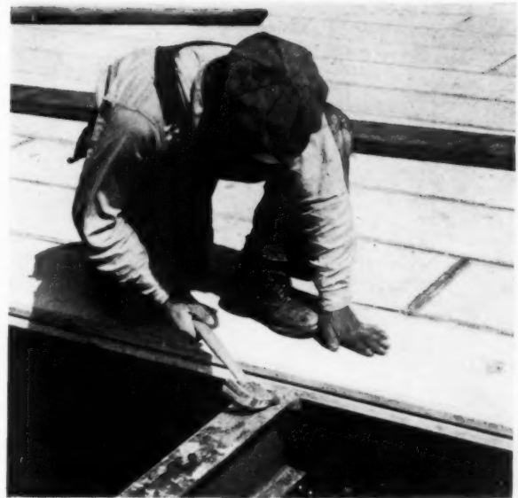
GYPSUM PLANK (GYPSTEEL), 2" in thickness, for floors and roofs. Edges and ends are tongued and grooved with steel. Can be surfaced with cement, linoleum or mastic.
