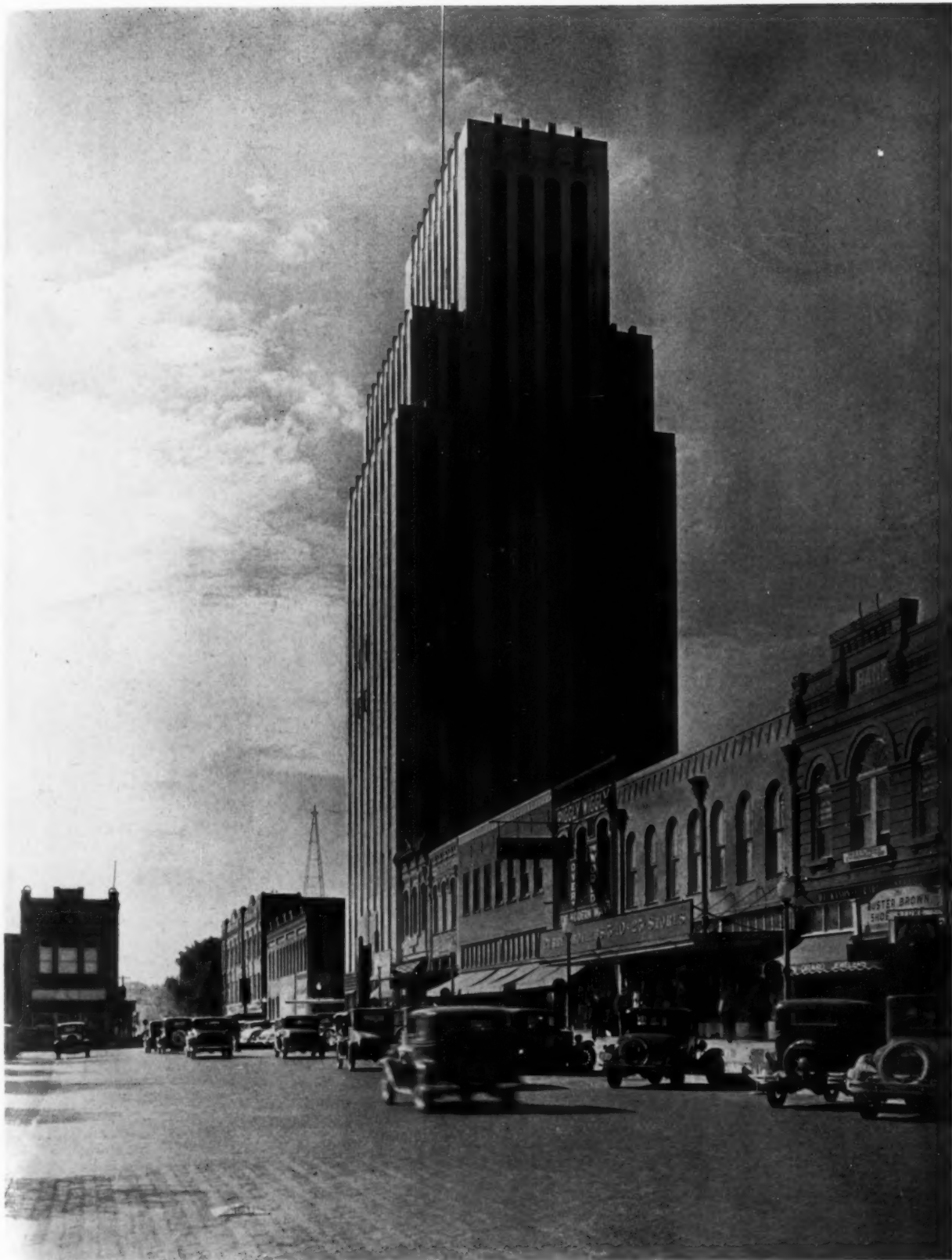
View down North College Avenue. First story is of black granite; upper stories of buff brick with cast stone spandrels.
