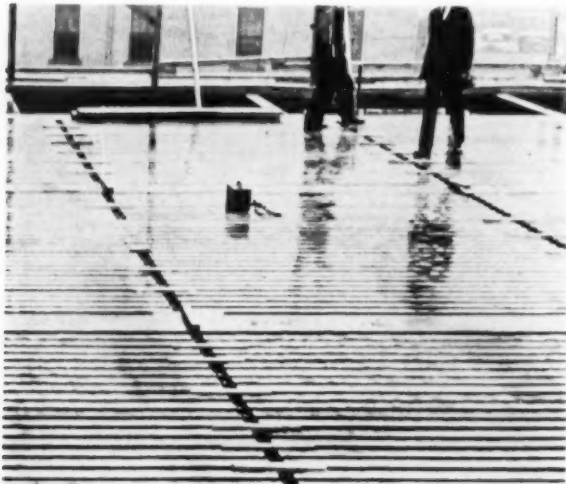
ROBERTSON STEEL FLOOR. A pressed steel, cellular type floor, factory-fabricated in lengths up to 12' and in 2' side units.
