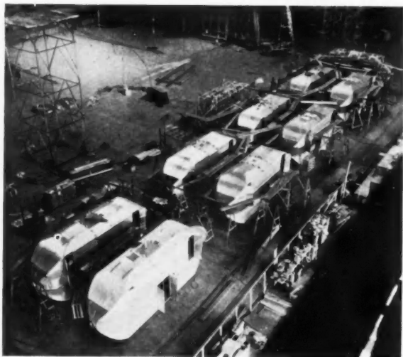
Rocket cars for the "Skyride" being constructed at Akron, Ohio.
