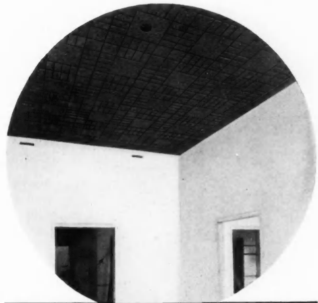
Construction photograph showing the application of Armstrong's Corkoustic to an office ceiling. Easily installed, this efficient sound-absorbing material insures quiet working conditions.
