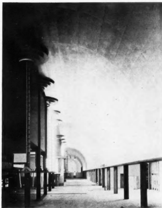
Agricultural Building. Ceiling in aluminum. Light shelf on right has orange-red lip, midnight blue soffit; reverse on left side.
