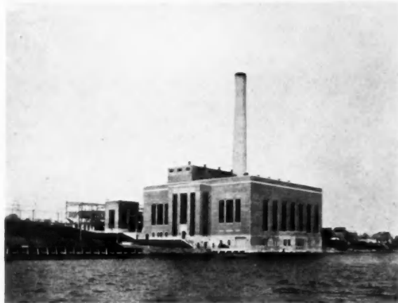
Somerset power station, designed and built by Stone and Webster, Inc.
