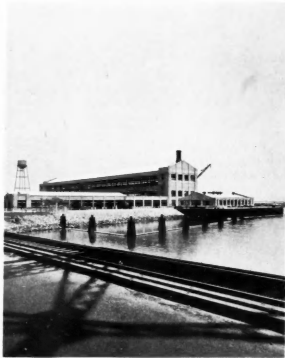
Ford Assembly Plant at Long Beach, California. Albert Kahn, Inc., architects.
