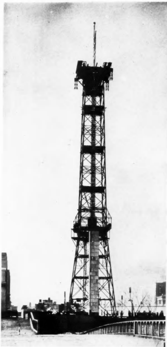
Progress photograph showing Tower under construction.
