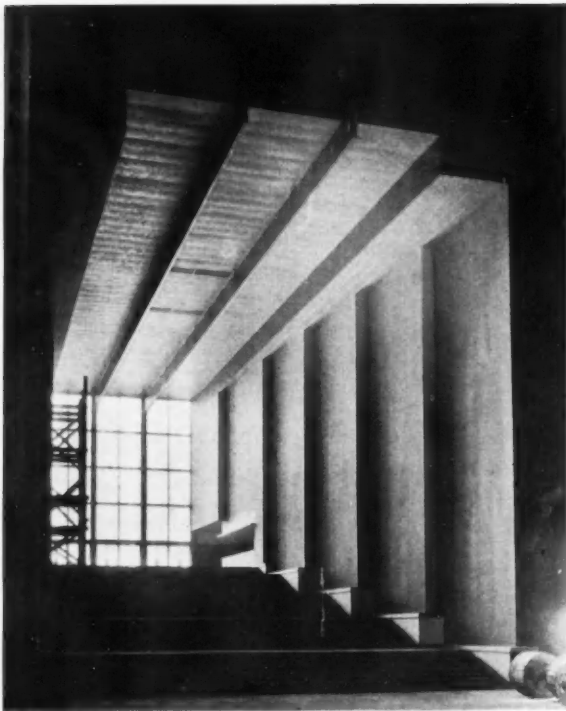
Electrical Building. Blue red ceiling; Federal red walls with orange effects; black walls at foot of stairs. Steel trusses painted aluminum; copper fins conceal red neon tubes.
