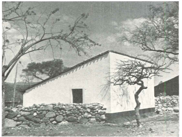
ADOBE WALLS, PLASTERED — TRADITIONAL METHOD
