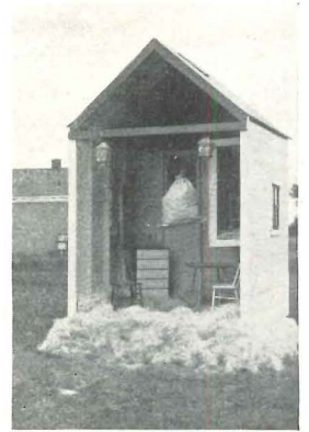
No. 1 These houses—No. 1 untreated, No. 2 flameproofed—were set afire to test a new paint.
