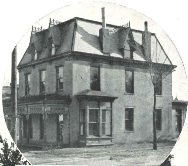
Before and after pictures of Petersburg, Illinois, residence modernized with the help of Atlas White stucco. Architects, Deal & Ginzel, Lincoln, Ill.; General & stucco contractor, Ed. Claussen; Owners, Thompson & Harms; Dealer, Apken Lumber Co.—all of Petersburg, Ill.
