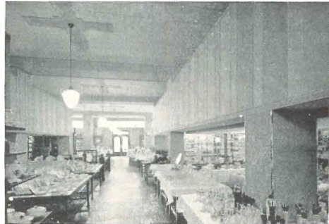
STORE —Modern effects like this are easily created with Nu-Wood. Notice the horizontal treatment of the walls with Nu-Wood Plank . . . the interesting ceiling pattern achieved by the use of Nu-Wood Tile between beams and Nu-Wood Board over the beams.
