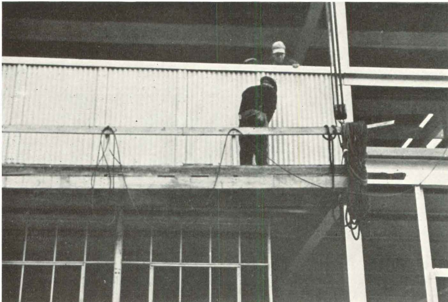
Large, lightweight rigid units make it possible for a small crew to erect many hundred square feet of curtain wall per day. The units come surfaced in either Flexboard (top) or corrugated Transite (below).
