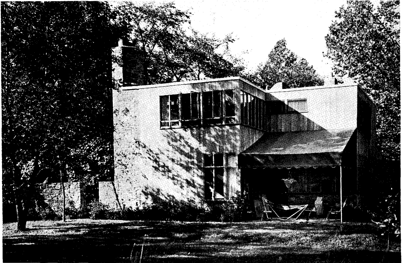
Taking advantage of previous excavations, the entrance court and garages (top) are located one level below the main living floor with its walled garden (below).
