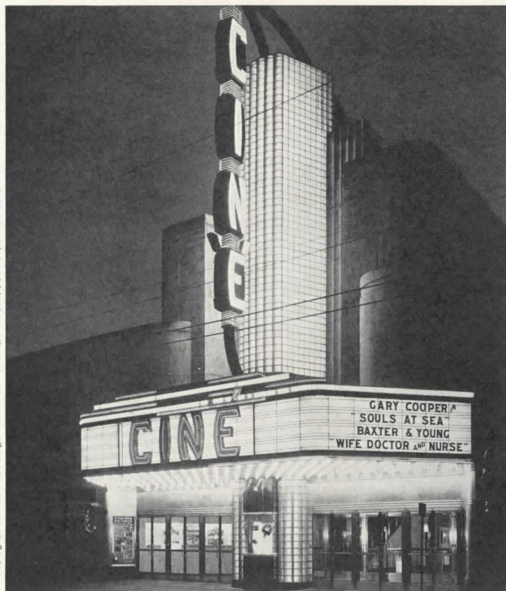
Photo by Hedrick-Blessing. G. W. & George L. Rapp, Inc., architects
