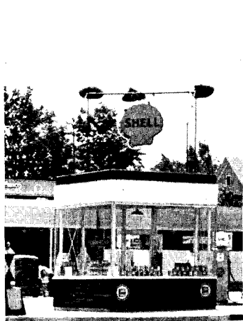
Glass-walled service station
