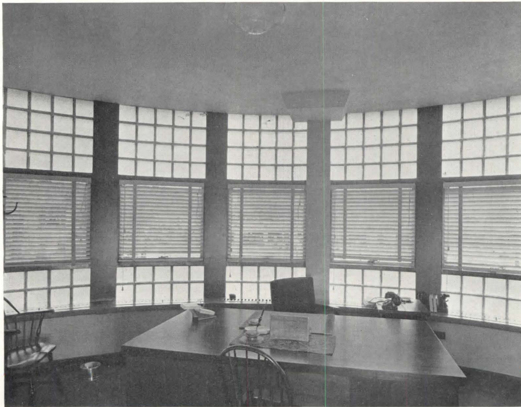
TOP: Retail shops have interior frontage on a spacious corridor leading both to street and to parking area. Use of glass block in wall reduces lighting costs. BOTTOM: Typical office. Each glass panel is about two-thirds glass block and one-third metal sash.
