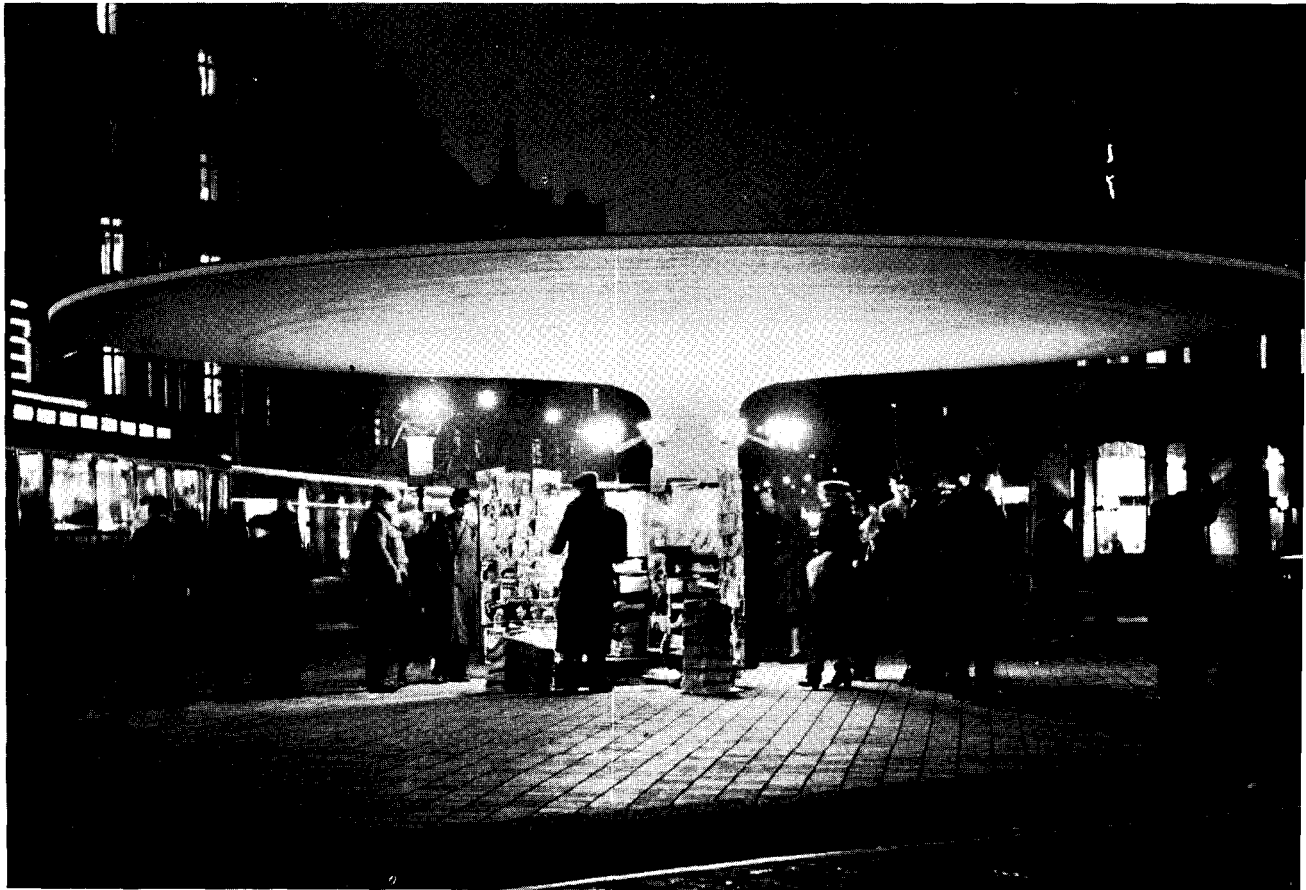
View of shelter at evening. This is a busy street intersection; trolley cars pass on three sides. In inclement weather, waiting commuters are shielded from snow and rain.
