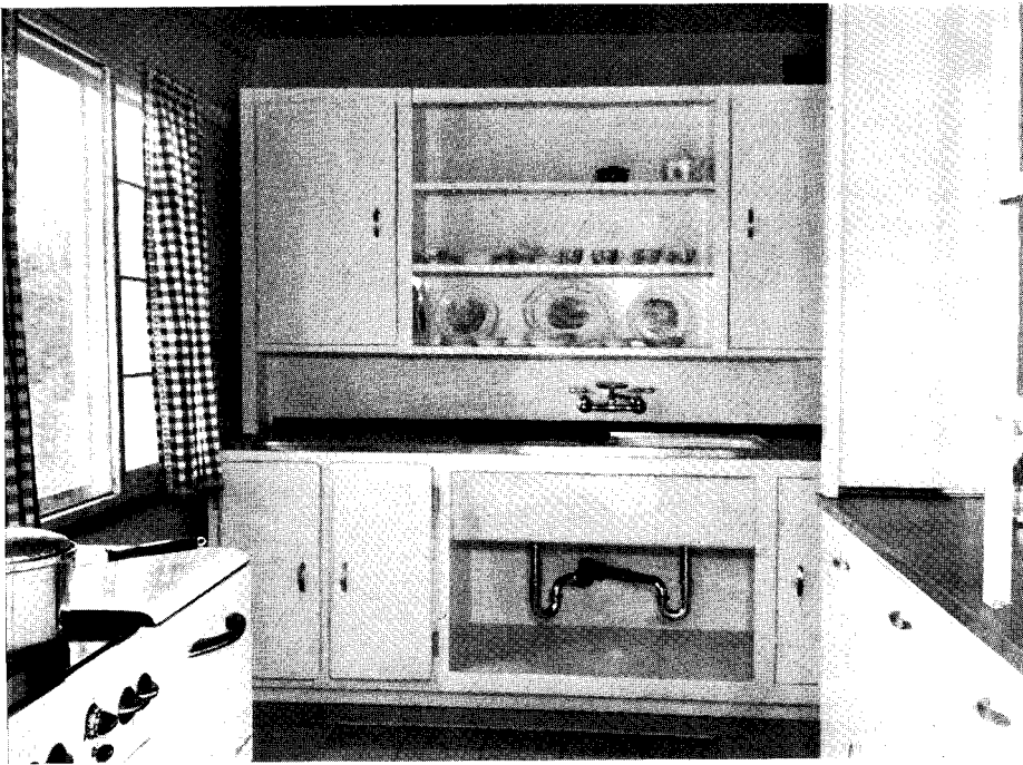
The kitchen (left) of the experimental house of the John B. Pierce Foundation at Lebanon, N. J. (AR, 8/39, pp. 41-45) contains a single large prefabricated unit embodying sink, icebox, storage cabinets, and shelves. All plumbing is in one wall; and bathroom waste pipes (right) are compactly assembled in a single unit above the floor.
