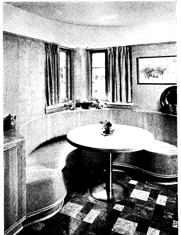
In dining alcove, plywood is red birch.
