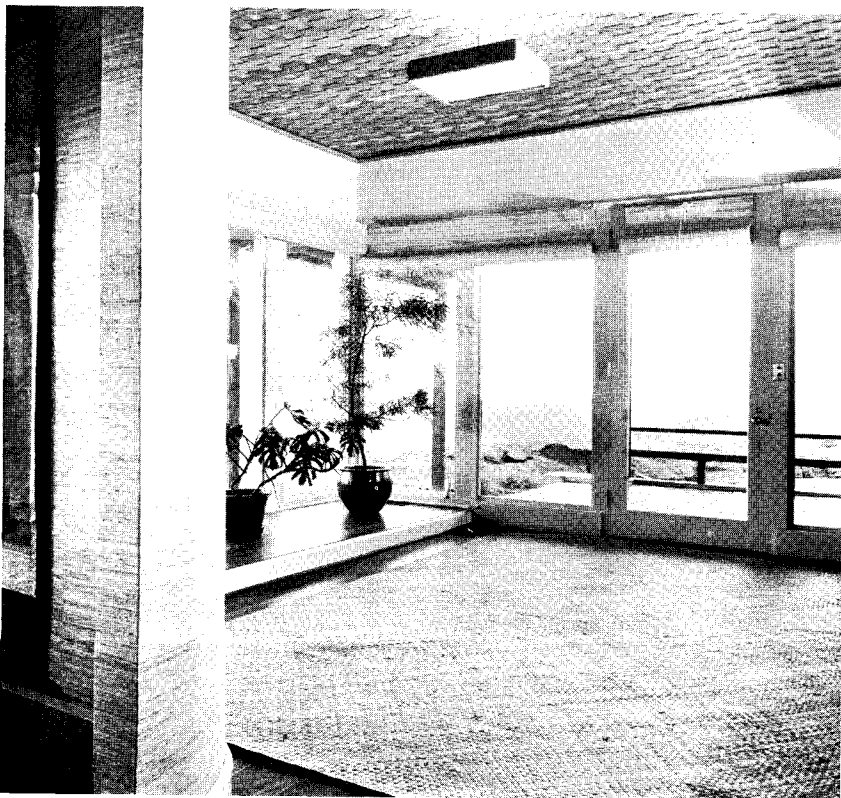
Entrance hall has two walls entirely glazed. Curved wall is surfaced with gold Japanese straw paper. Ceiling is of 3-in. woven fir slats.
