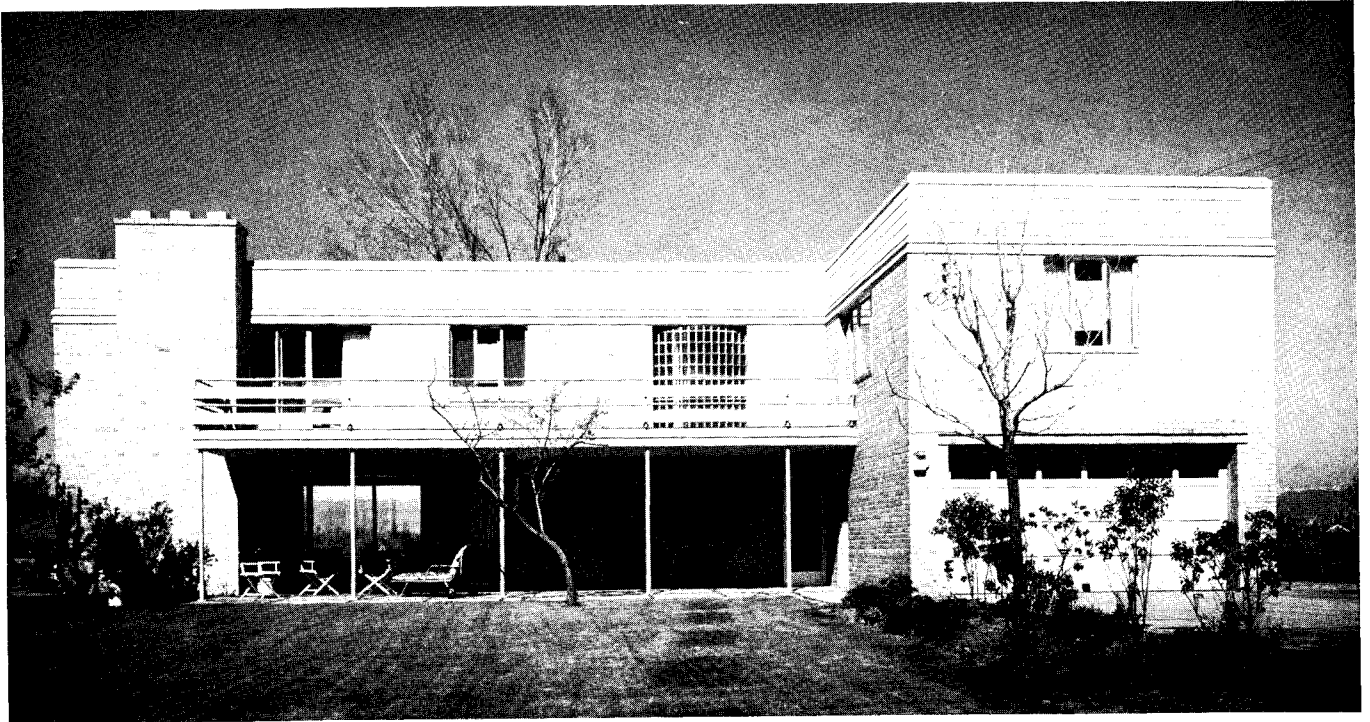
View from rear, showing living terrace which has colored cement floor, canvas-covered deck over.
