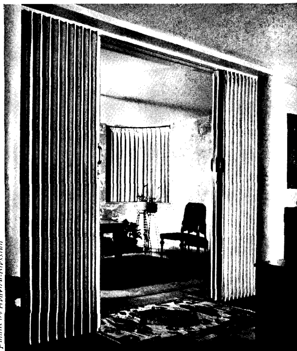
Penthouse: modernfold accordion doors are used between dining and living rooms; a vertical light trough is concealed behind pilasters at either side.
