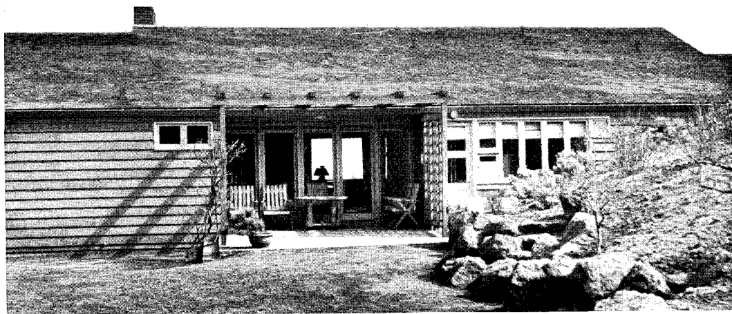
View from west, showing dining terrace in relation to service portion of the house.
