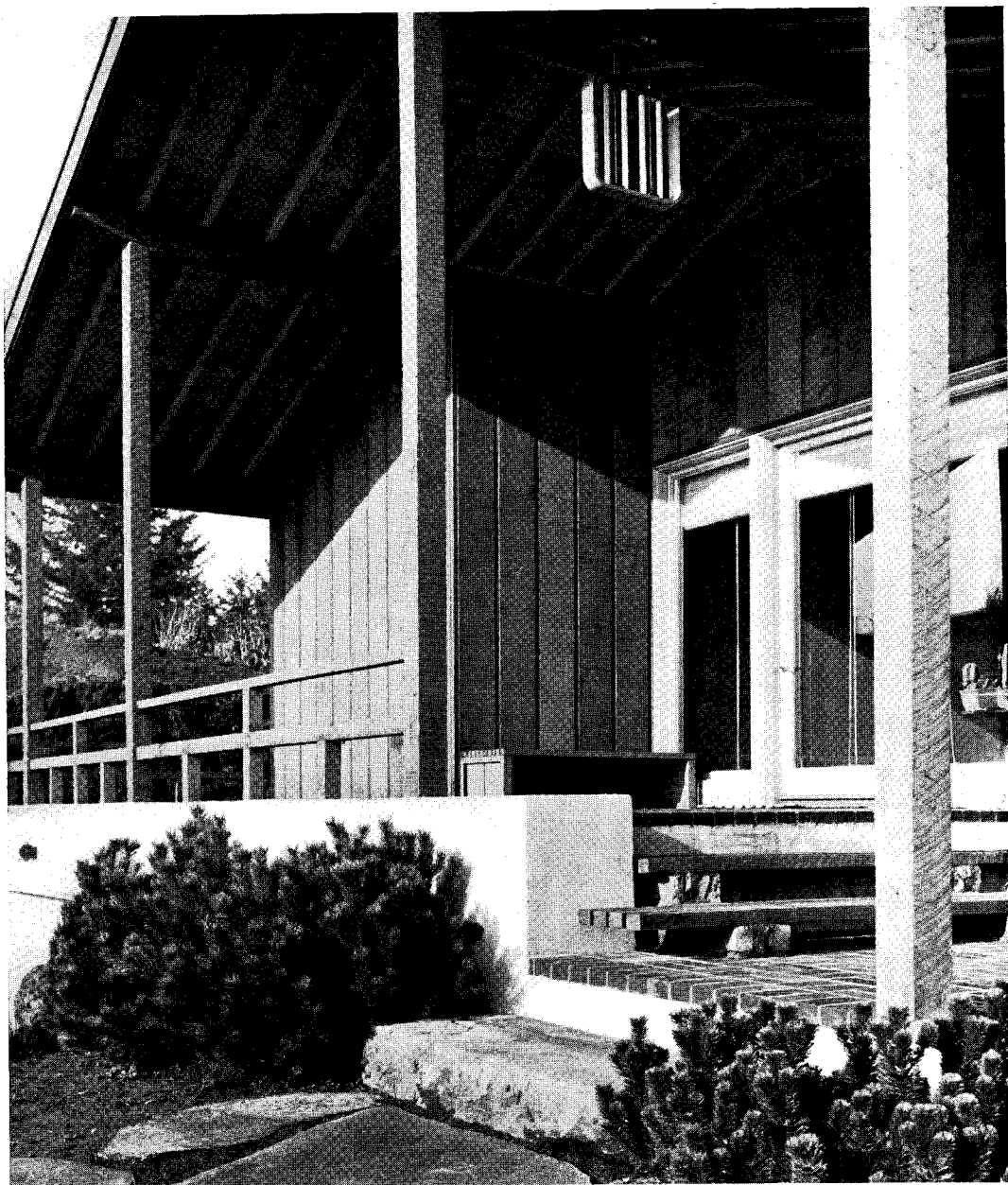
Detail at entrance. Rough spruce timbers and siding are treated with iron chloride stain and with Minwax.
