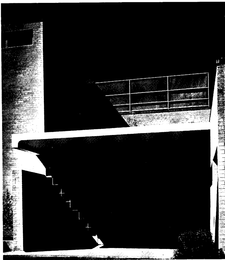
Entrance on south. Circulation is from the lobby to the right into main locker room, to the left into corridors leading to visiting-team rooms, coaches' offices, officials' room, and track entrance on west.
