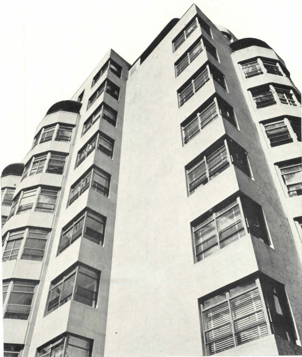
Frame is reinforced concrete construction cantilevered over bays and corner windows.
