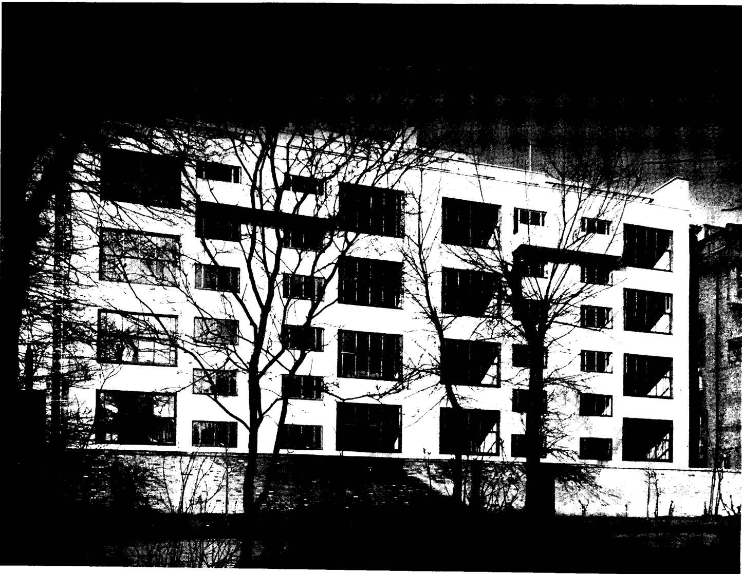
The garden front of the Palace Gate building gives a graphic picture of the "three-two" planning system. Although superficially reminiscent of the "studio type" plan, the Coates system provides much more flexible and satisfactory organization of interior space.
