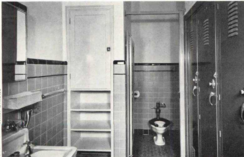
Service room, four-bed ward, St. John's Hospital, Springfield, Ill.; Henry R. Helmle, architect.
