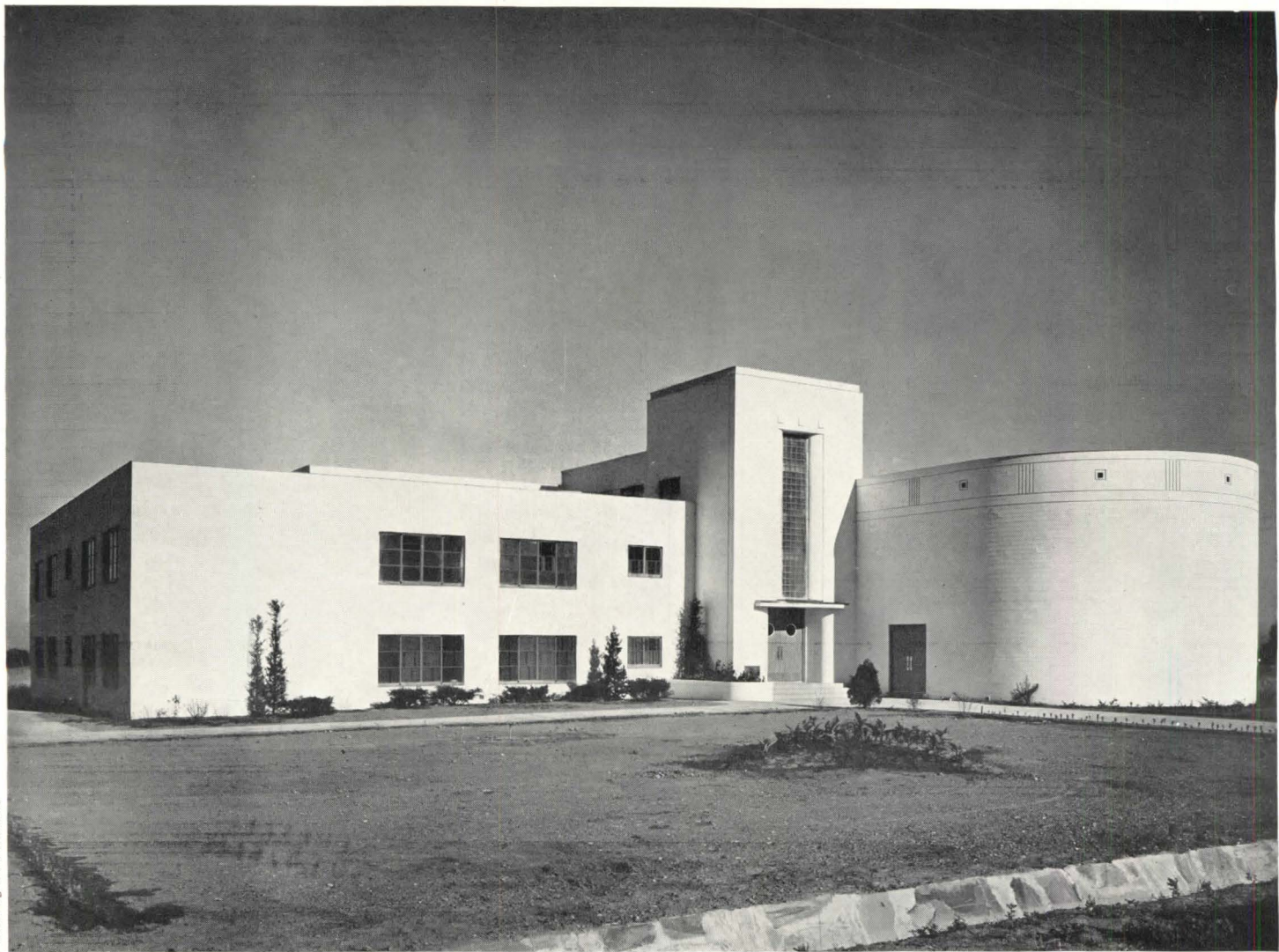
The marks of the form boards are left as a surface texture. All the sash are Soulé steel with felt weatherstrip.
