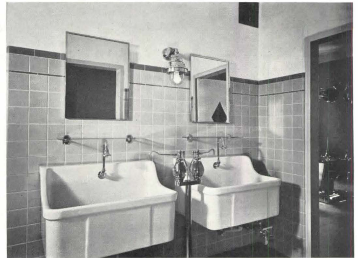
Scrub-up room, adjoining operating room at left; note knee-operated faucets and "explosion-proof" lights.
