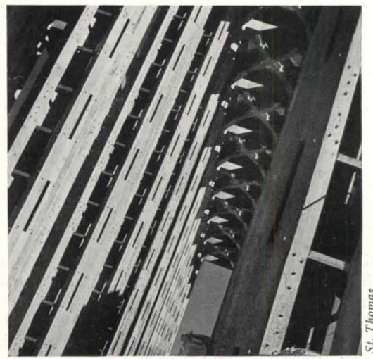
Fig. 8. Columns built up of timber and plywood.
