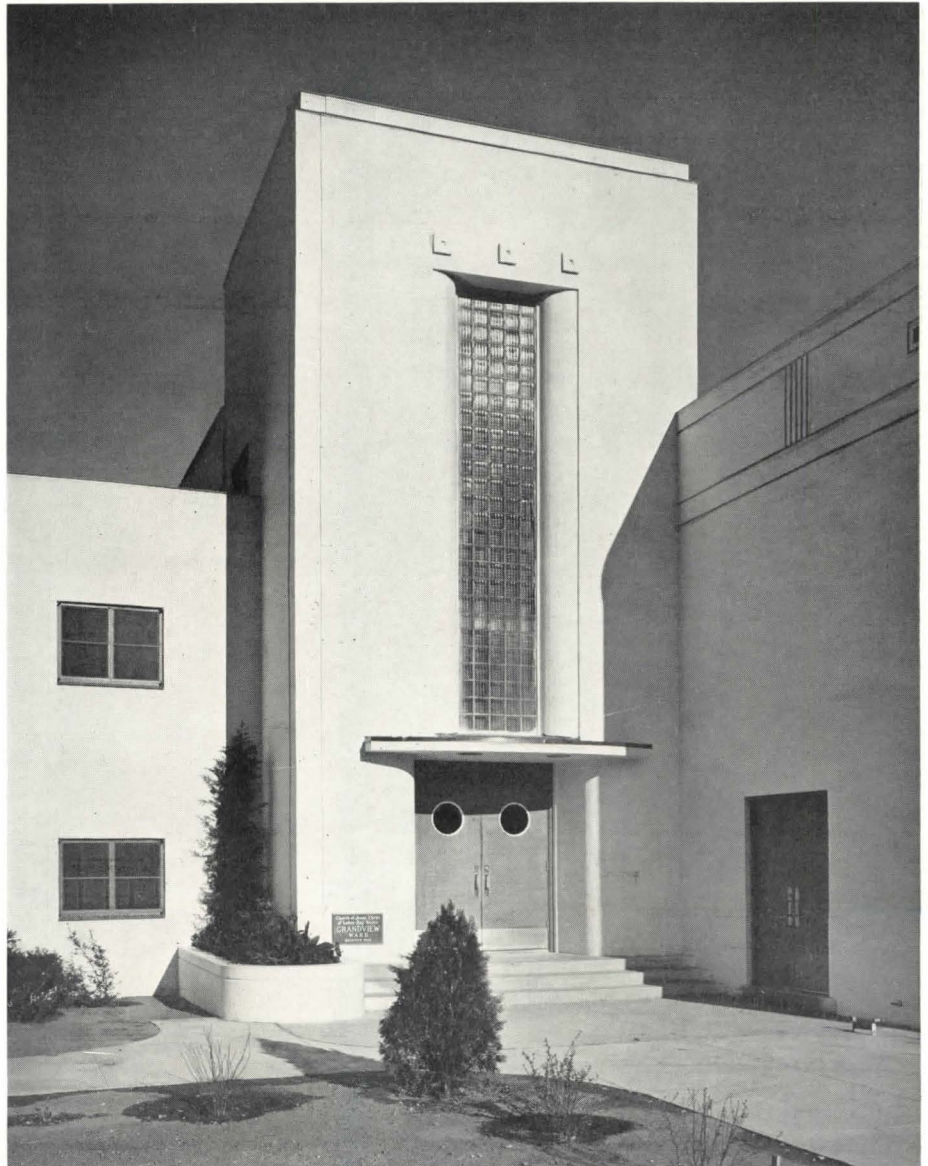
The two-story entrance tower dominates the design and separates the public and semi-public functions of the building. The vertical panel over the entrance is Insulux glass block.
