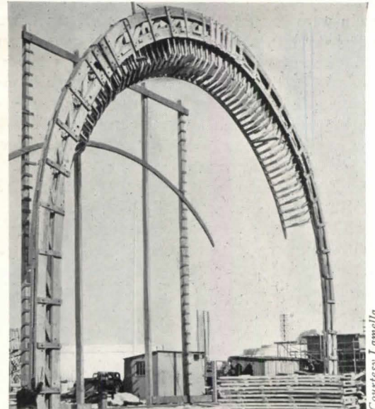
Fig. 6. A timber frame for a monumental arch.
