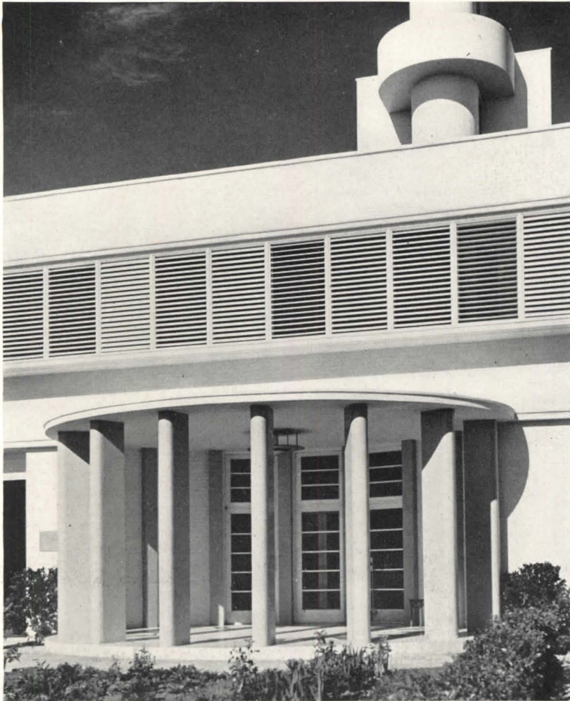
Detail of the adjustable louvered shutters outside the dormitory windows, shown in the photo at left
