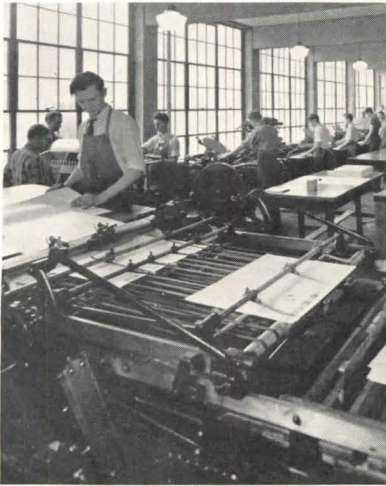
Printing shop, New Britain, Conn., Trade School; Warren S. Holmes Co., Architects.
