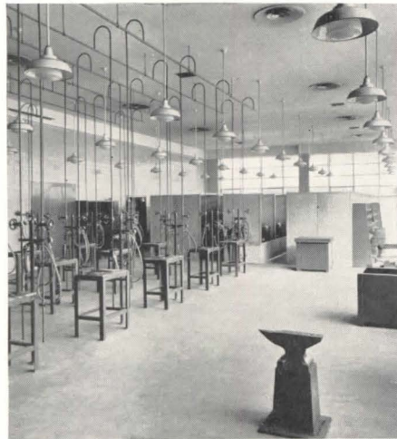
Overhead services, welding shop, South Vocational High School.
