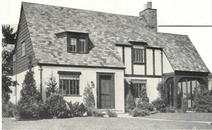
One of the many houses Mr. Cheel has built in the past 15 years with exterior walls of stucco. Prices range from $8,500 to $45,000. Mr. Cheel finds stucco, made with Atlas White, creates the appearance and economy that ring up sales. Architect for above, J. Norman Hunter, Teaneck, N. J. Stucco made by Artstone Rocor Corp., Brooklyn, N. Y.
