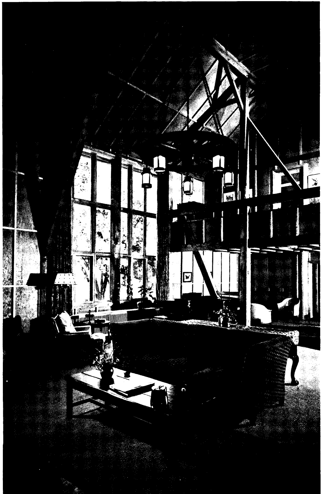
View of living room, facing north. This room is three stories high, with a balcony over one end of it. Beyond, on the balcony level, are six bedrooms and a sitting room. The walls of the living room are fir plywood; finish is natural stain. Sash are stock, cut to required size.
