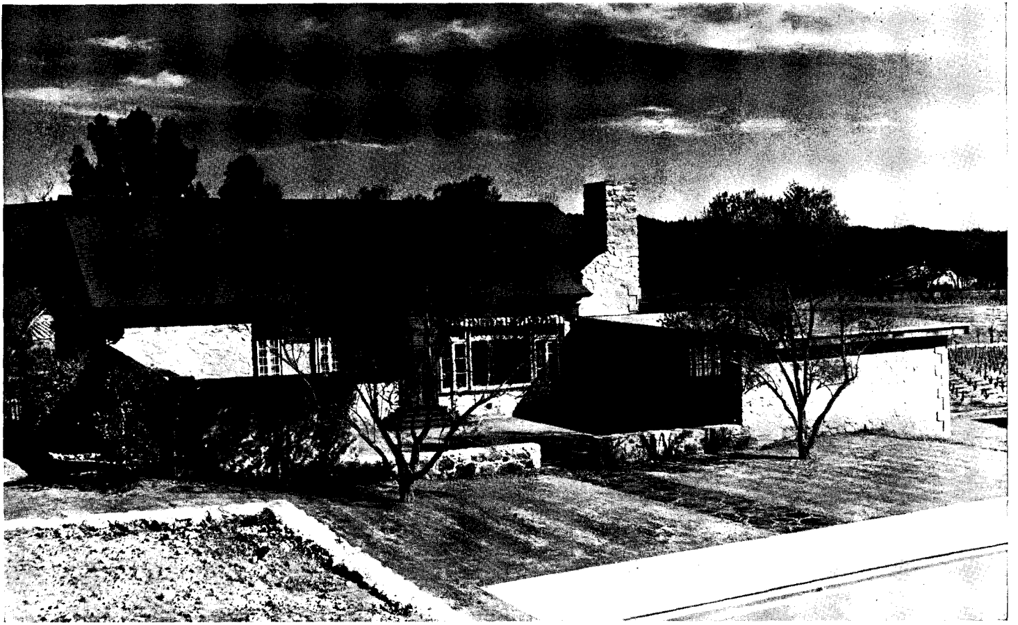
View from the south. The terrace and the flat roof over part of it are pitched slightly; the roof was originally the second floor of the winery and was pitched this way so that water used in washing the wine vats would run off.
