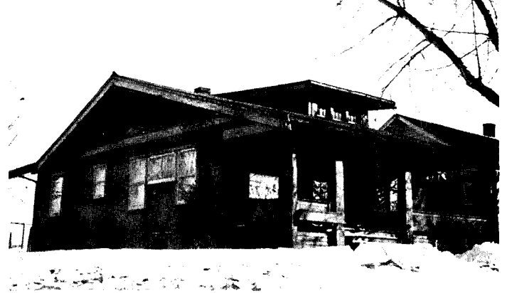
Iowa house: original market value, $3,800. New siding, exterior, redesigning, painting cost $696; sale price, $4,500.
