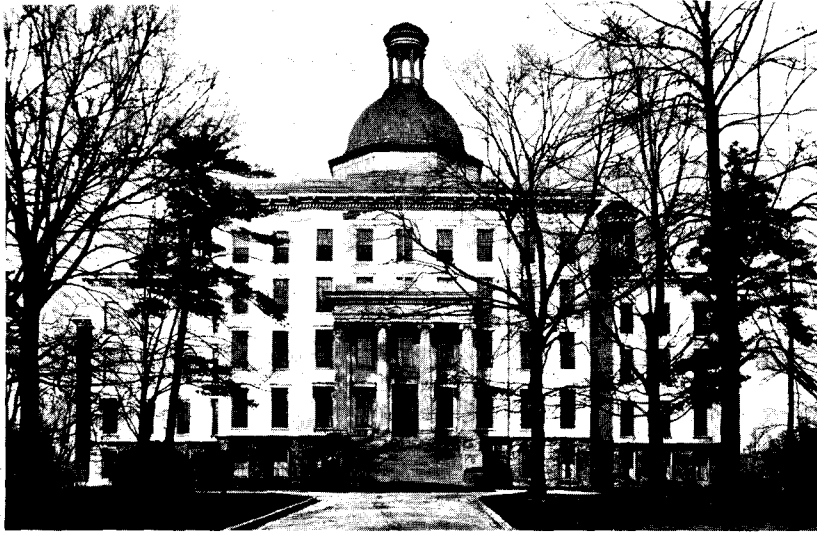
FIVE VOTES: Kentucky School for the Blind, erected 1855. Francis Costigan (1810-1865) was architect for this example of Greek Revival.
