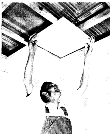
Metal ceilings can easily be furred down
