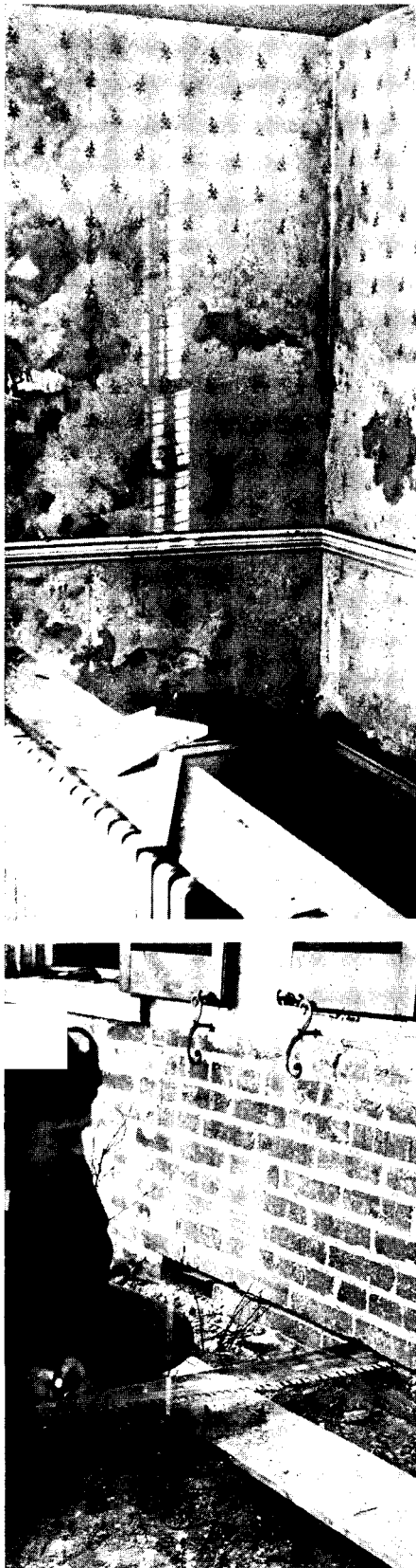
Top, damage caused by water seepage from masonry foundations. Below, preparing to install membrane waterproof by sawing wall at a brick joint
