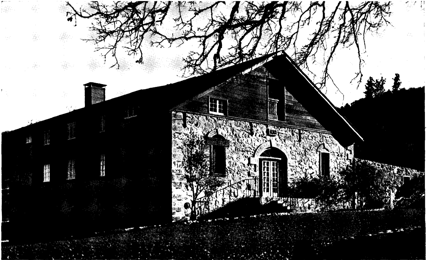
View from the east. The structure is located about 150 yards from a main highway. Wood gables replace original stone.
