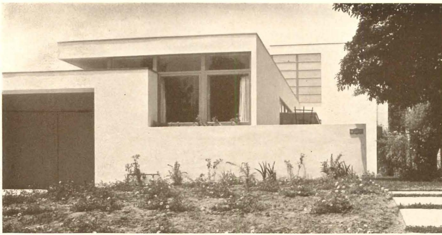
Street elevation: note clerestory windows which give added light to the den.
