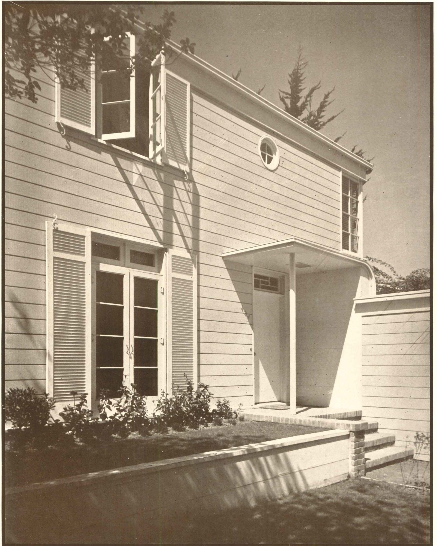
Presented herewith is a group of houses selected for their variety of solutions to a common planning problem. Some are suburban; others offer ingenious answers to the problem of a narrow lot. First in the group is this residence in San Mateo, Calif.
