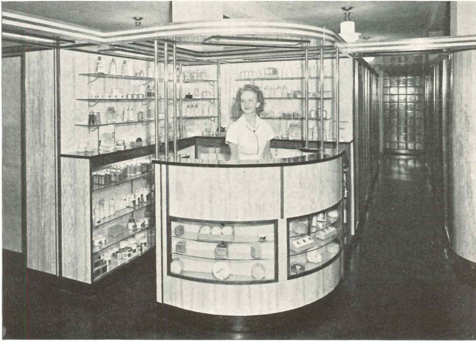
Top, elevator lobby; below, interior of ground-floor shop
