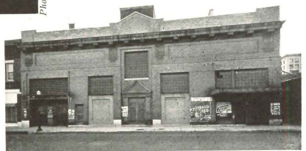
Old theater building before remodeling
