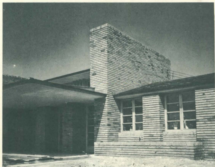
ENTRANCE DETAIL, north side.
