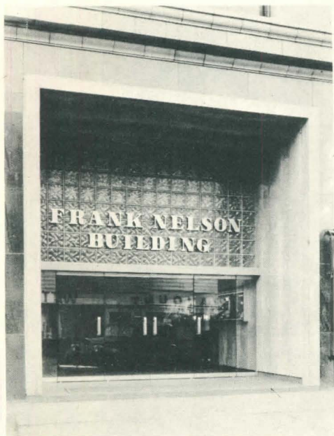
ENTRANCE after remodeling
