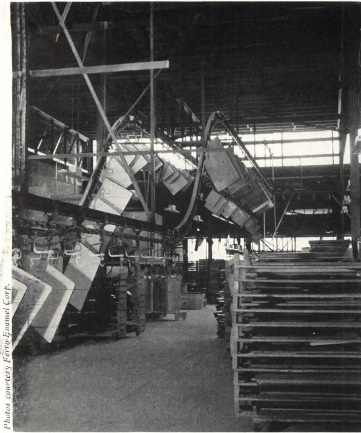
Conveyor takes finished ware to assembly line
