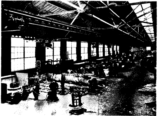
Suspended conveyors add to truss load
