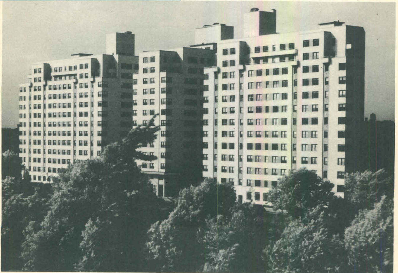
ABOVE: Aaron Colish, Architect; 2601 Parkway Apartments, Philadelphia.
