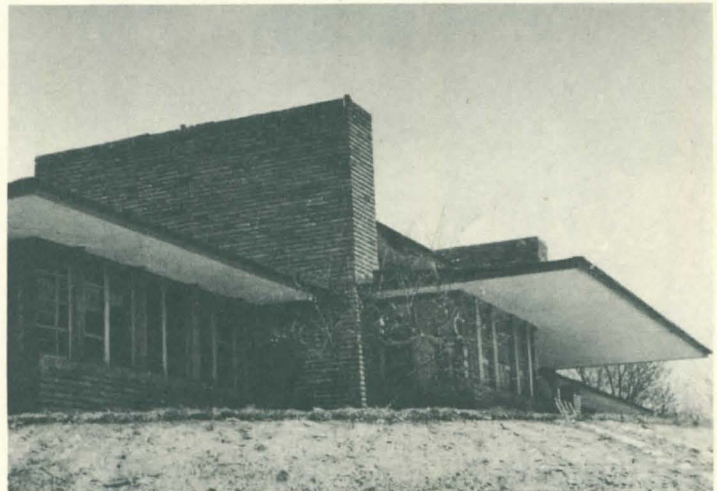
DETAIL OF CANOPY on south side.
