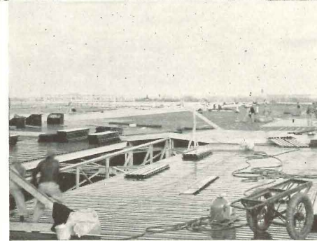
As soon as the first area of Q-Deck is laid, application of insulation and waterproofing is carried on concurrently, thus making sp
