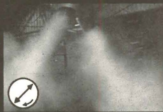
4 Still turning through 270° the streams of heated air are covering every part of the working level.
