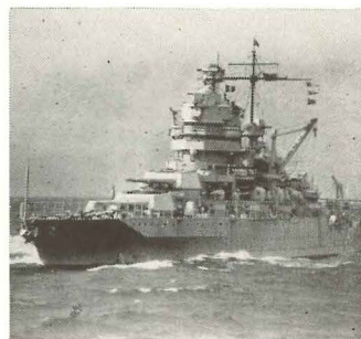
BATTLESHIPS are a maze of pipe and tubes, from stem to stern.
