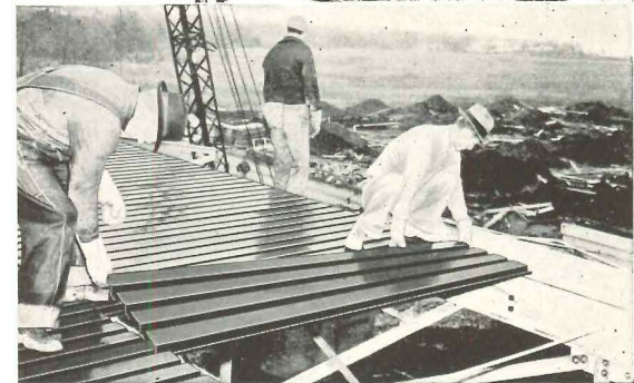
The speed with which these units are laid is an important factor in making possible the construction of an acre of roof in one day.
