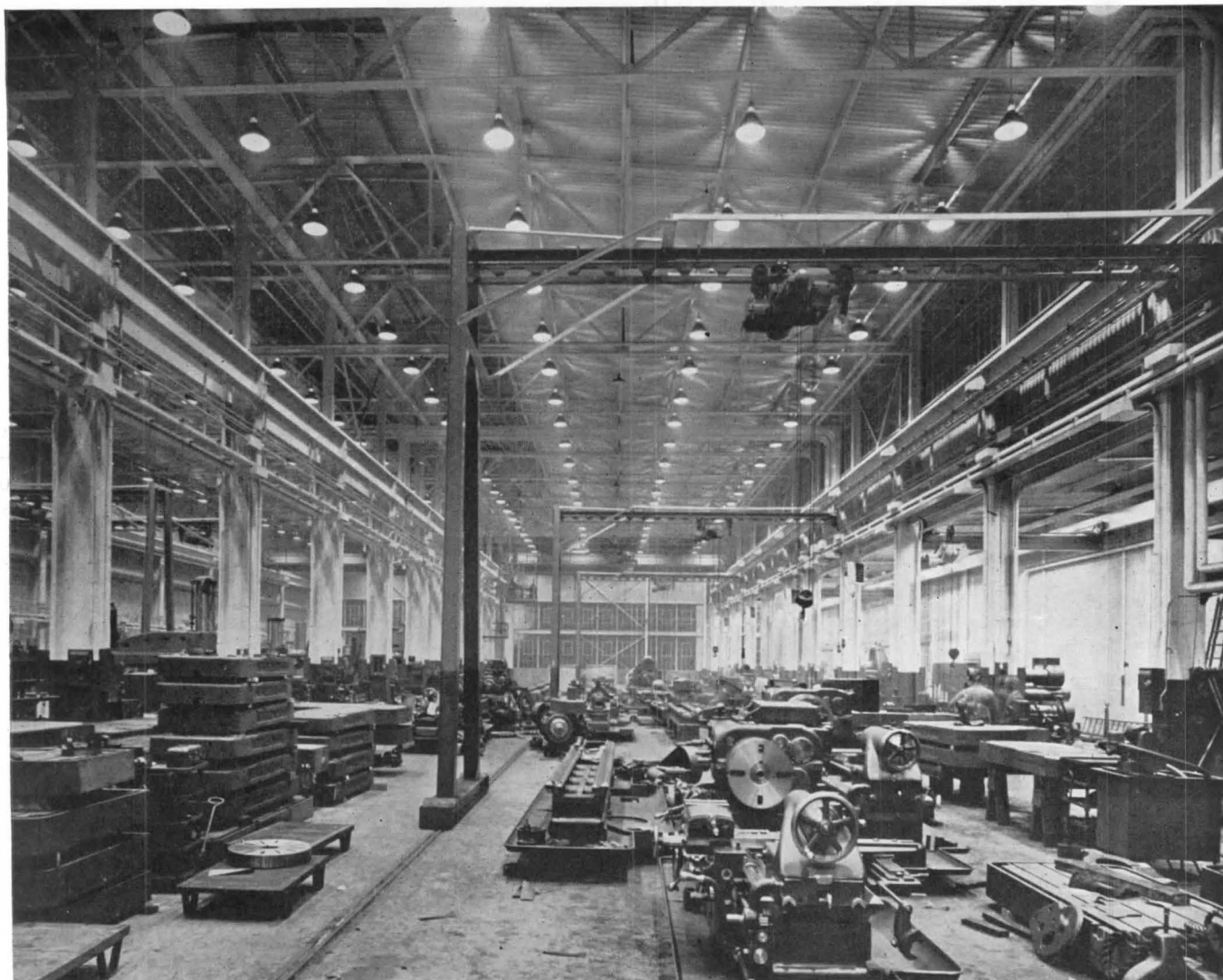
3000-watt mercury lamps in porcelain enamel reflectors located on nominal 35 ft. by 40 ft. centers. The illumination in service is about 35 foot-candles. Fixtures may be lowered for cleaning or relamping
