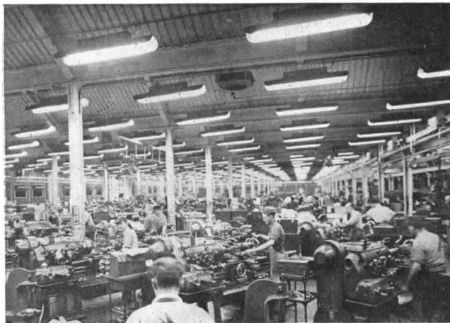
The maximum utilization of floor space is accomplished by well distributed lighting. The system employs 2-lamp fluorescent units on 10 ft. by 10 ft. spacing, 12 ft. and 13 ft. high
