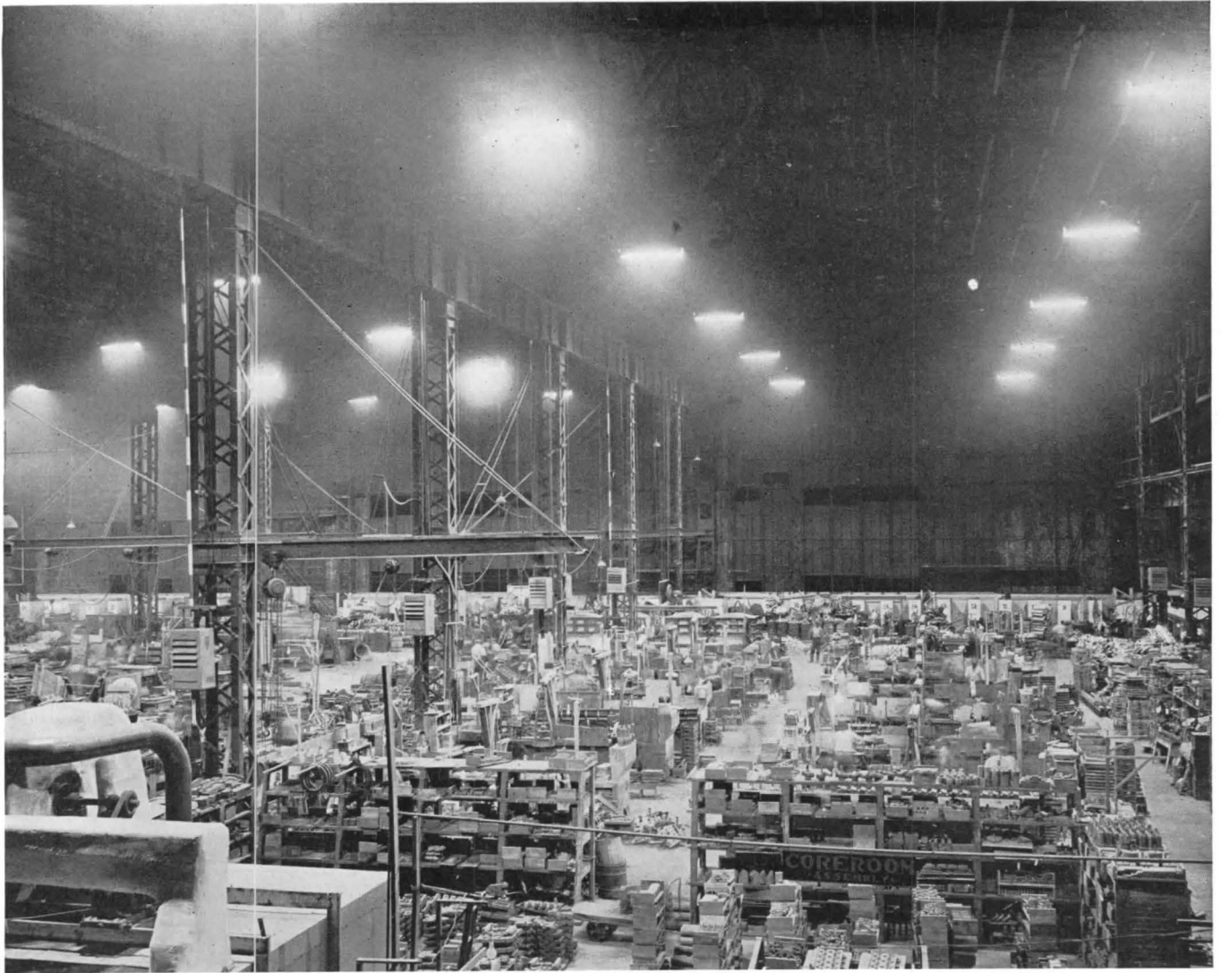
An area of 22,000 sq. ft. is lighted by 220-400 watt mercury lamps mounted at a height of 32 ft. They provide about 60 foot-candles of illumination for the critical visual task performed
