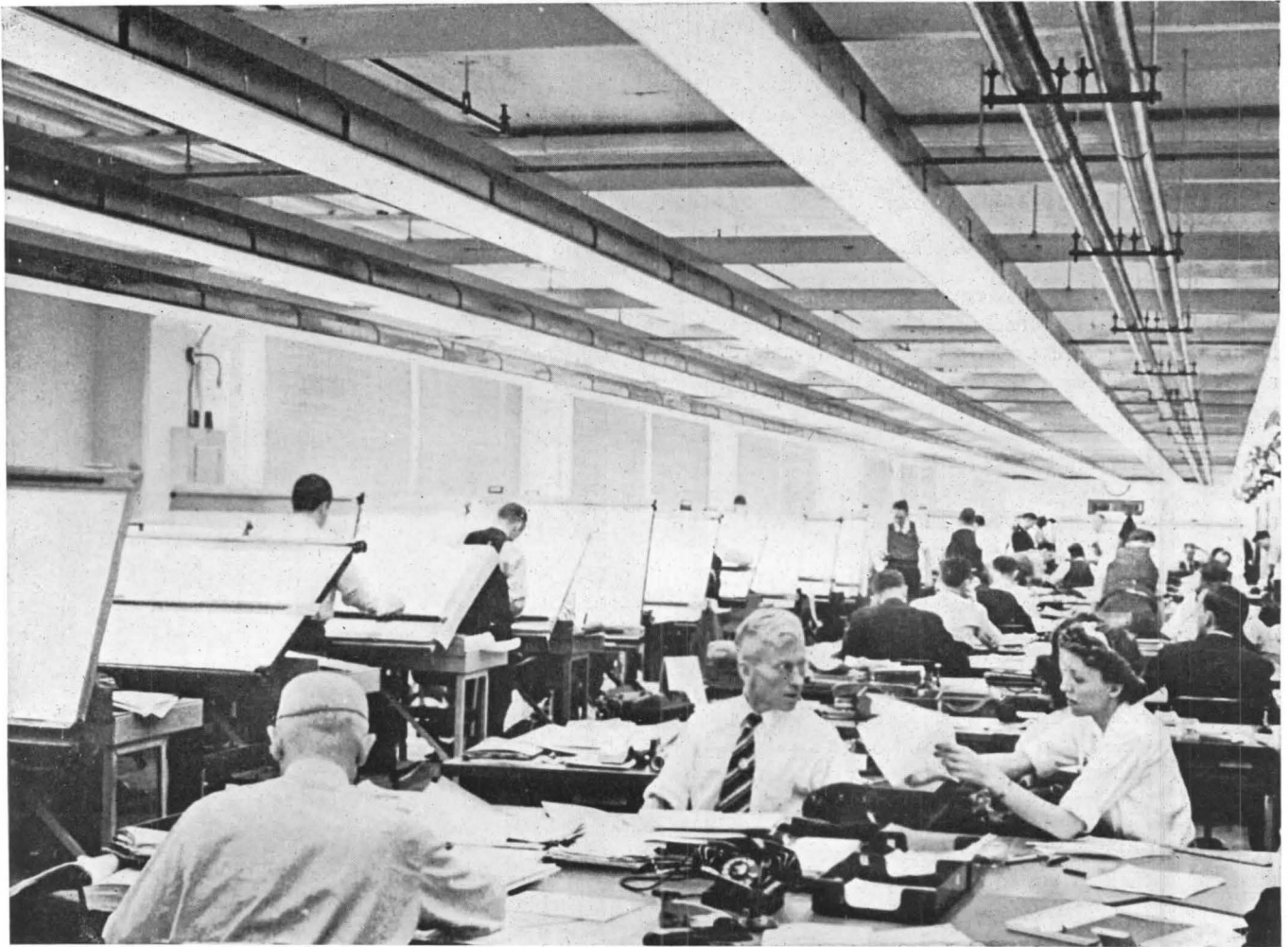
In this continuous row installation, one 40-watt fluorescent lamp in each troffer section provides an illumination of 50 foot-candles for this combined drafting room and office of a defense plant
