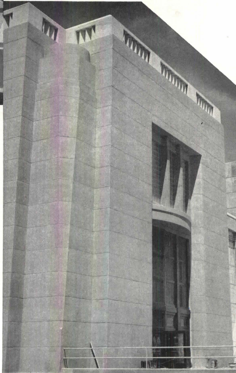
Rustication lines give scale to mass walls of Santee-Cooper powerhouse. Building designed by Harza Engineering Co., Chicago. Built by Central Engineering Co., Davenport, Iowa.
