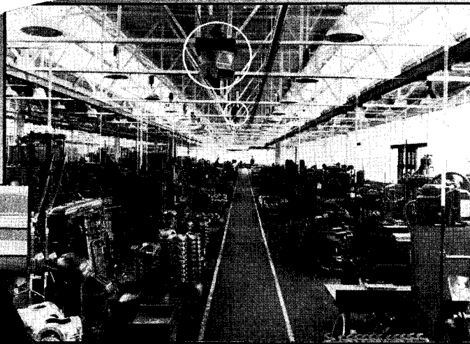
Wing Revolving Unit Heaters in modern defense plant. Note congested areas that would obstruct heat from fixed discharge heaters.
