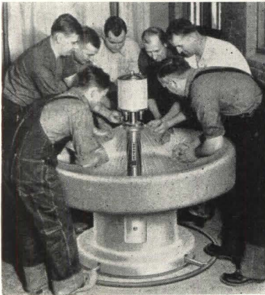
Section of modern ordnance plant washroom—showing Bradley Washfountains in foreground and Bradley 5-stall Shower at rear.
