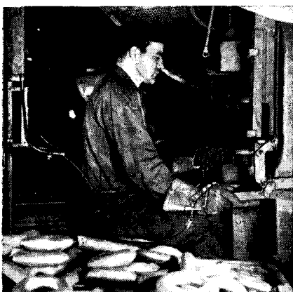
AUTOMATIC HAND GUARD —This man is operating a trimming press. If he should absent-mindedly let his hands move too near the danger zone, the two cables will automatically whisk them back to safety, before the ram of the press descends.
