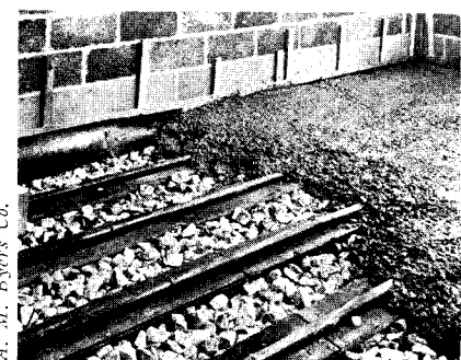
Pipes for panel heating run in floor fill
