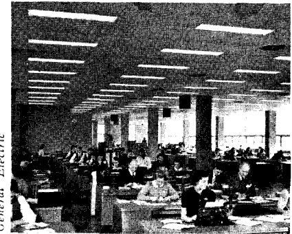
Flush-mounted troffers on 6 ft. centers
