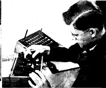
Taking Temperature Readings with Potentiometer at 43 Thermocouples.
