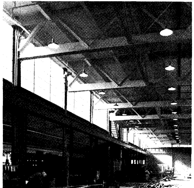
Warren type steel trusses have main chords of 18" T's (half of 36" I), eliminating gusset plates and vertical unstressed members
