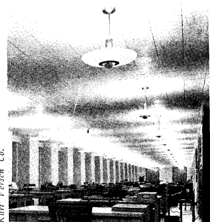
Plastic luminous-bowl ceiling fixtures
