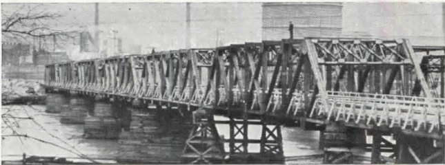
PITTSBURGH. Fleming Park Bridge—756' (six 126' spans) was built for 12-ton trucks and 30-ton street cars. Designed by Allegheny County, Pennsylvania. Detailed, prefabricated by Timber Structures, Inc. Erected by J. F. Casey Co., Inc. and McCrady Construction Co., Aspinwall, Pa. Verne Ketchum, Engineer for Timber Structures, Inc.
