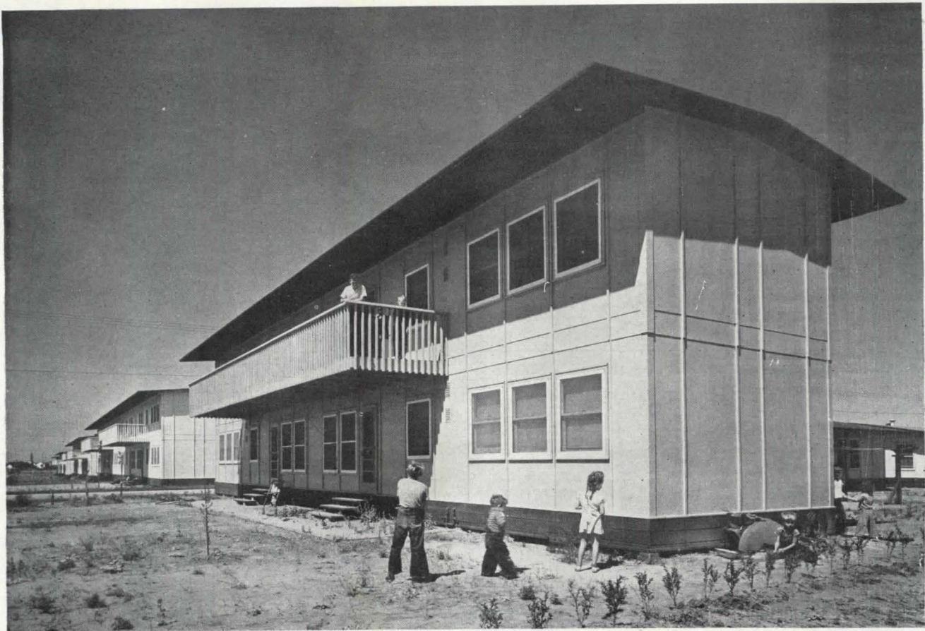
In the multi-family units there is no "back door;" stairways run directly through to a balcony on the garden side, with apartment entrances on either side of the stairs. Experimental houses proved the merit of Wurster's railing design; there are no cross pieces for children to climb. Balconies are wide enough for a couch
