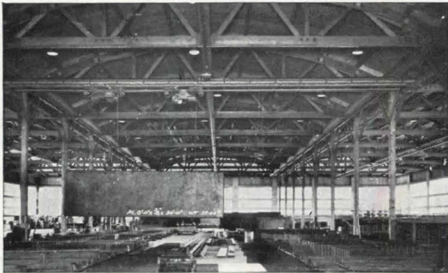
PORTLAND. Steel warehouse for Woodbury & Co. The roof of this 200'x300' building is supported by 35-67' trusses, 15 lb. dead load, 40 lb. live load, plus 14,000 lb. concentration at center line of bottom chord and adjacent to each end of the truss. Concentration supports a three-point suspended traveling crane. Architect: Richard Sundeleaf. Contractor: Wegman & Son.
