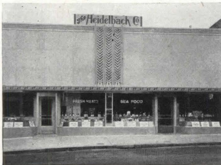
↓ ARCHITECTURAL CONCRETE SLABS , precast with an attractive design carried out in colors—brick red and black on buff—give distinction to the Heidelbach Company store, Baltimore, Md. Architect: J. R. Kennedy; slabs by John J. Earley; both of Washington, D. C.
