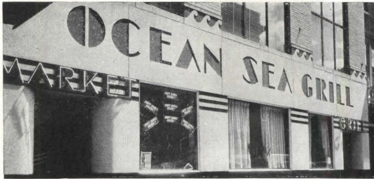
↑ OCEAN SEA GRILL , Bridgeport, Conn., modernized with a facing of Architectural Concrete Slabs. Base—polished black; field—white quartz tinted to a light green; stripes, large letters and water wave—red vitreous aggregate. Architect: Herbert C. Elton, Bridgeport; slabs by the Dextone Co., New Haven.
