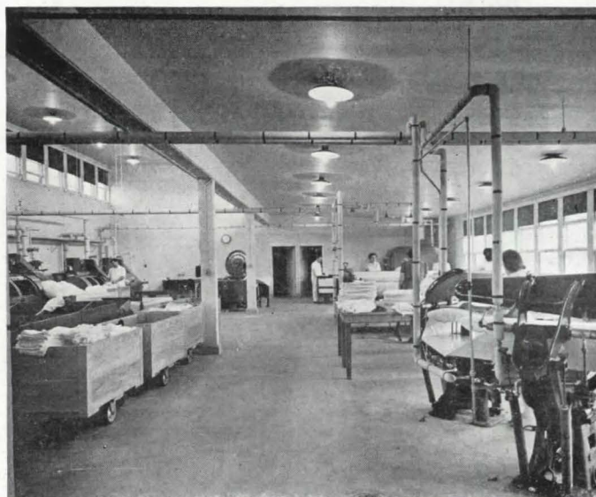
Right center: the nursery is equipped with cubicles made of shatter proof glass and plywood. At the bottom is a general view of the laundry. Note large windows near the ironers, and monitor type over the washing machine area
