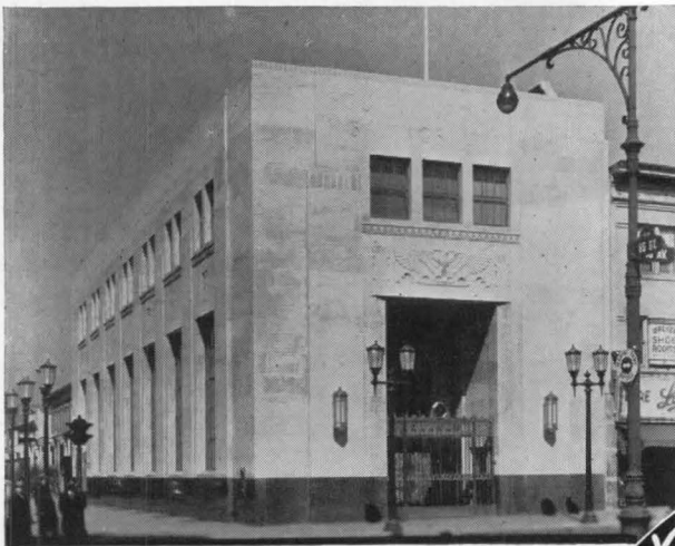
South Brooklyn Savings Bank (Brooklyn, N. Y.), Dudley E. Soper, Architect. Child & Scott-Donohue Inc., Heating Contractors. BOILER PLANT — 2 — H. B. SMITH No. 34 "MILLS" BOILERS.
