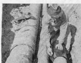
Installing connector band. All necessary accessories are pre-fabricated and shipped with order.
