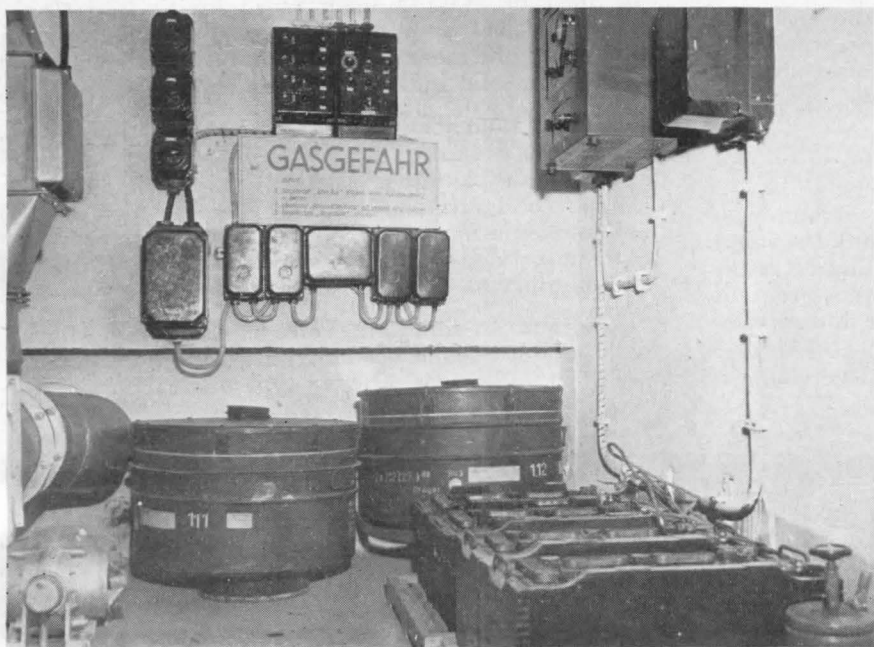
Below: the air conditioning and gas filtering units inside the air raid bunkers. Intake and outlet pipes are on the left. Spare filter units are seen in the lower center. At the right are batteries for emergency power
