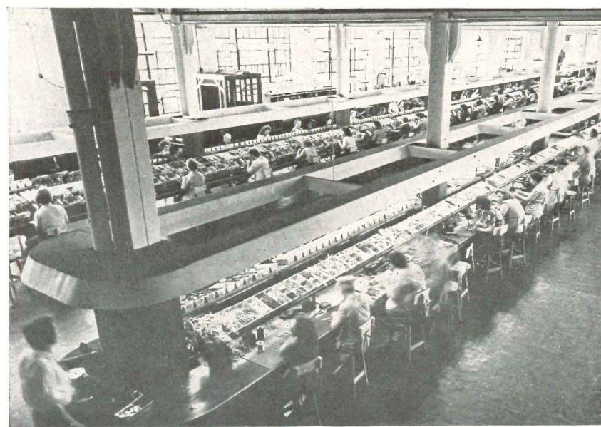
12. In this installation (same one shown above) the problem is complicated by the double assembly line; workers must face light from the opposite fixtures
