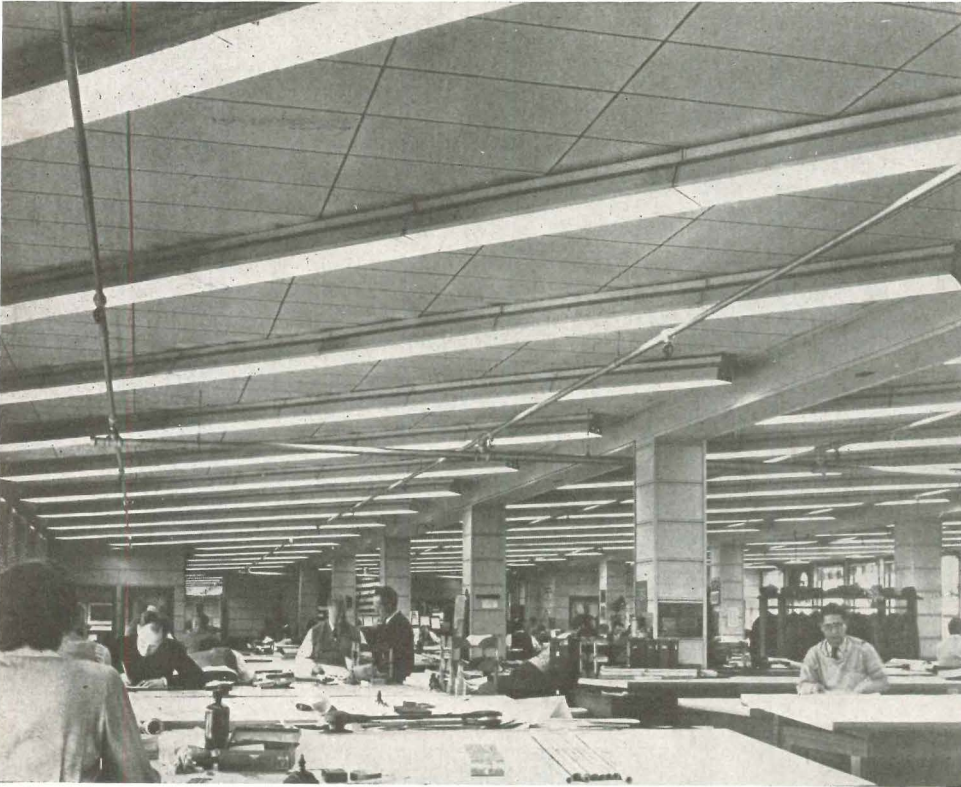
16. Fixtures placed diagonally minimize shadows across drafting boards for the Willamette Iron and Steel Shipbuilding Co. Photo courtesy Edwin F. Guth Co.
