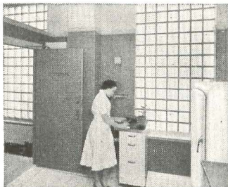
IN FACTORIES —Panels of Insulux help solve problems of light, temperature, humidity and dust control.
