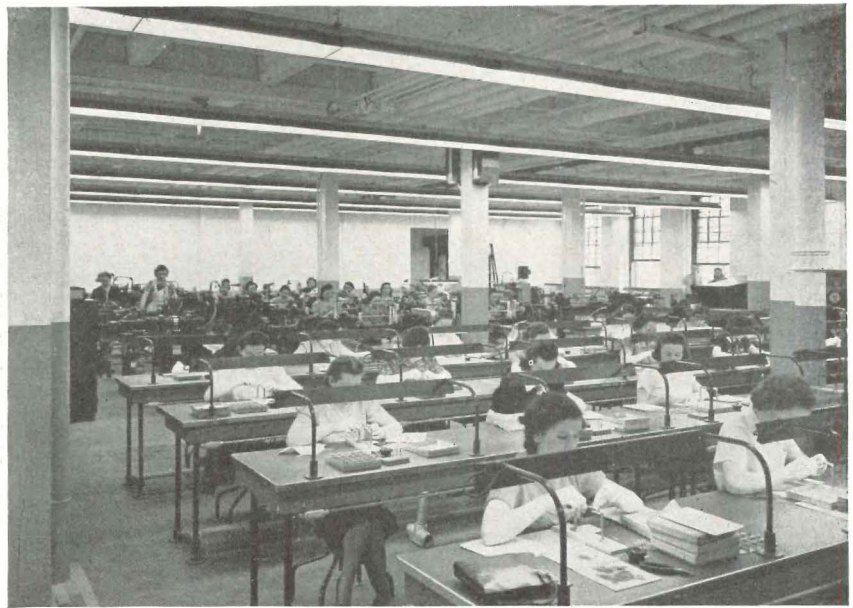
13. For extremely critical seeing tasks it is good practice to add localized lighting to the general lighting. Long fluorescent fixtures are usually good
