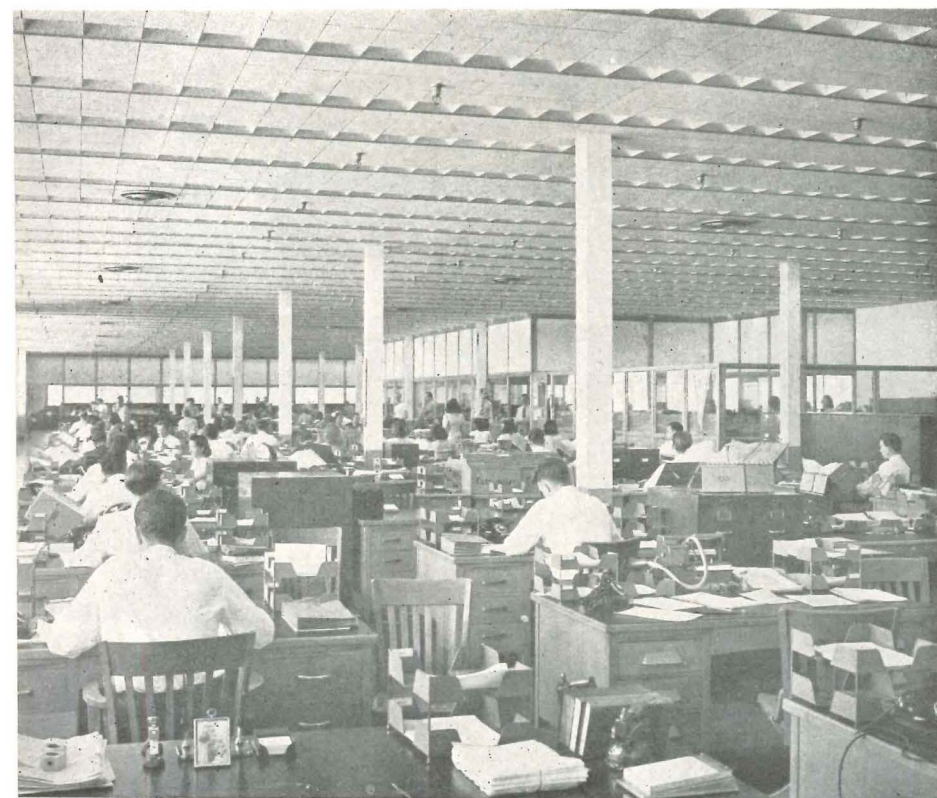
21. Daylight view of same office (above). The author points out that the troffers do not look much brighter at night than when the lights are out, by day
