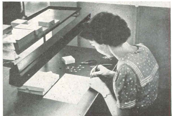
14-15. With good supplemental lighting the worker can either utilize or avoid specular reflections from polished objects. White background increases visibility
