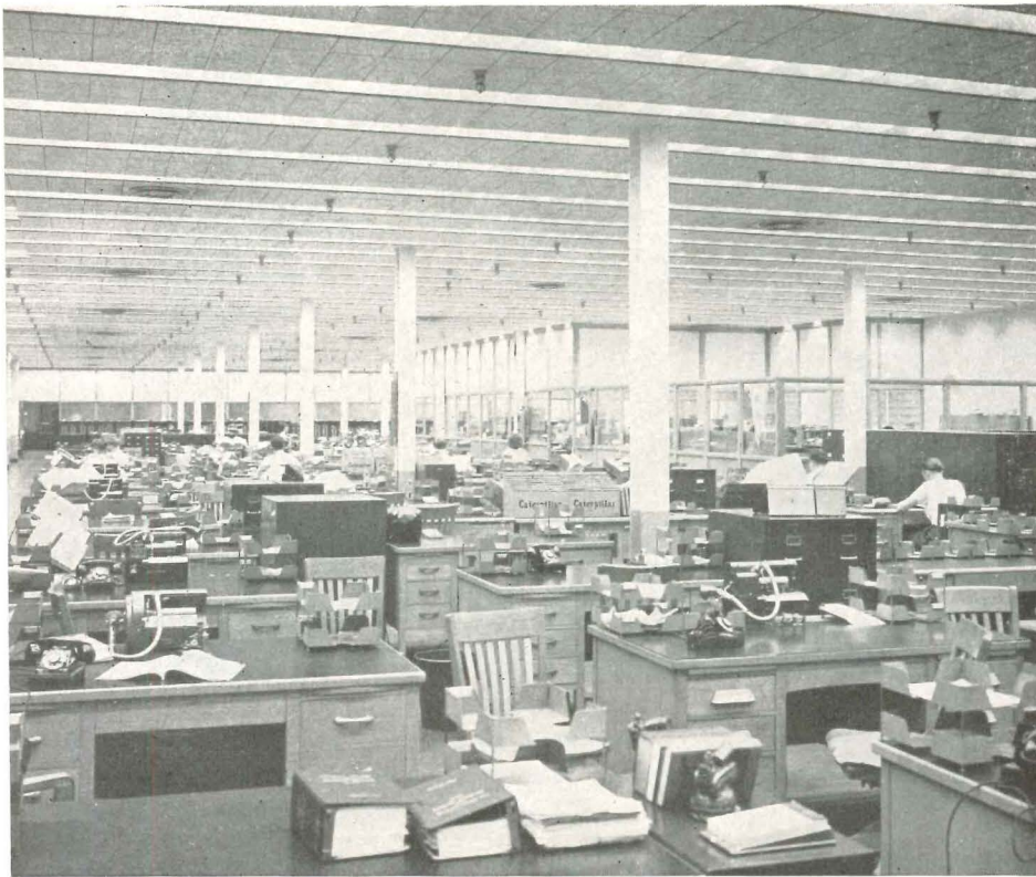
20. Night view of Caterpillar Tractor Co. offices, Peoria. Adequate, even lighting from open troffers, with baffles, aluminum finished, recessed in ceiling
