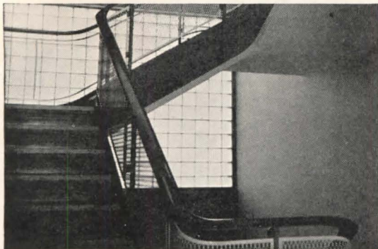
SPERRY GYROSCOPE COMPANY , precision manufacturing, Long Island, New York. Insulux panels bring light to stairways and other dark corners in factories or homes. Insulux transmits and diffuses light better than ordinary windows.
