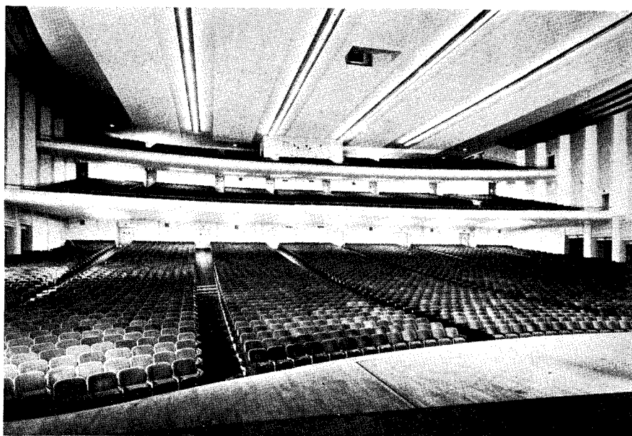
Fig. 11 and 12: Two views of Purdue University Music Hall, Walter Scholer, architect. Reflections broken by balconies, paneled rear wall surfaces, and sound-absorbing materials
