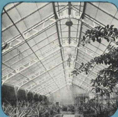
Here is structural strength combined with lightweight -- a job for which Alcoa Aluminum is ideally fitted.
