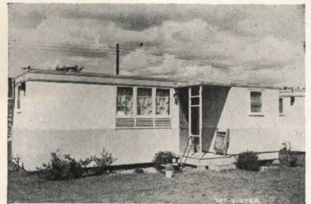
Wingfoot's two-bedroom prefab has telescopic wings to permit delivery by truck
