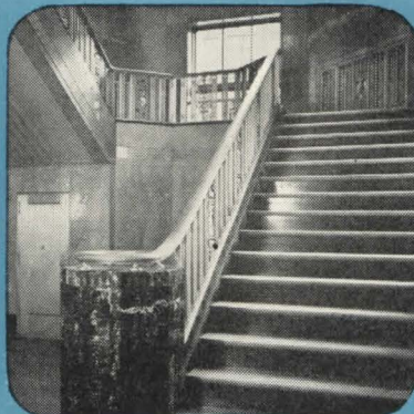
Utility and beauty are combined in aluminum guardrails. With little maintenance, these will keep their attractive appearance for years.
