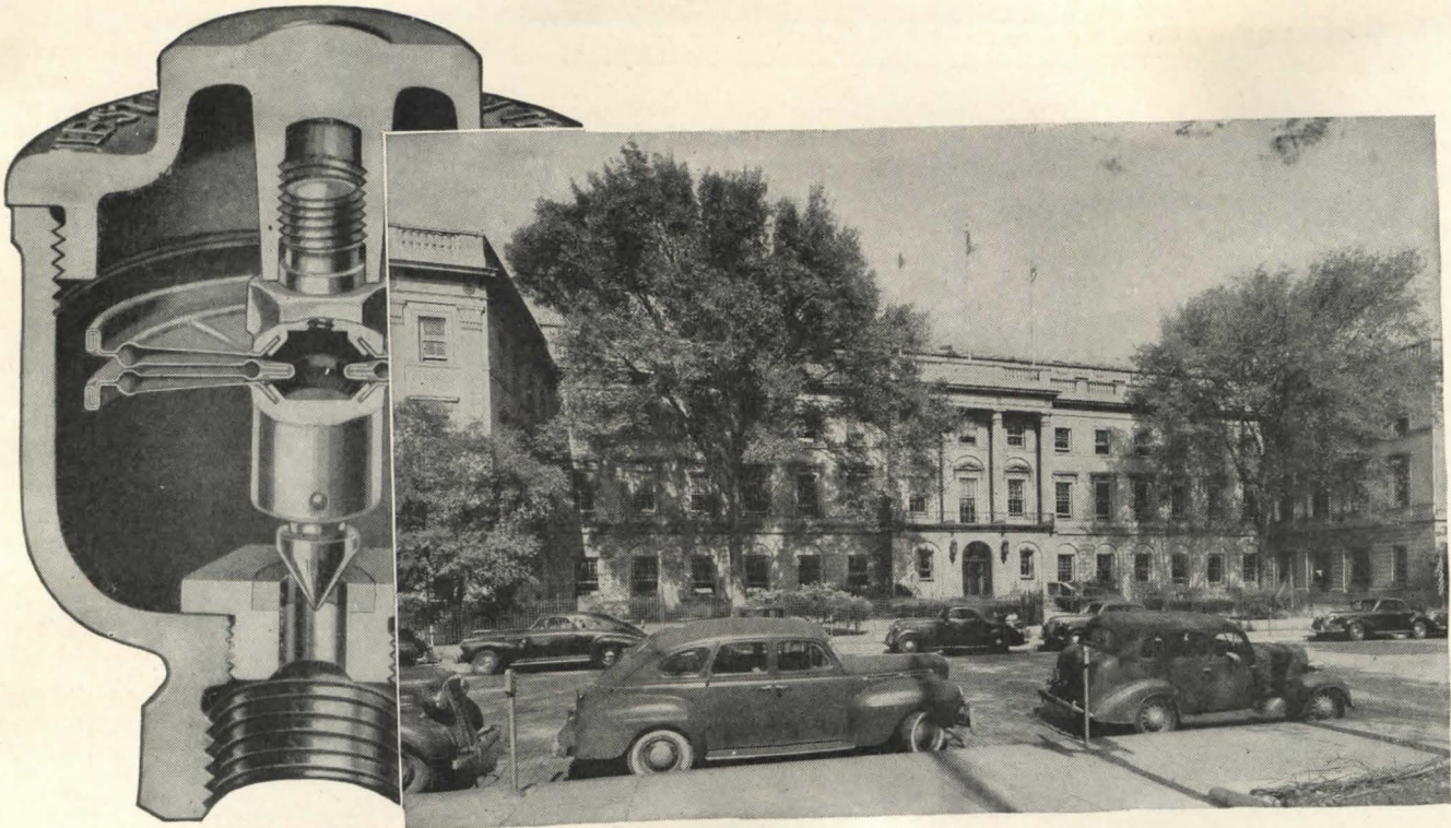
Twenty-six years' service! Initial installation in 1918... interior "thermostats" replaced in 1944! That's the record of Webster Thermostatic Traps in the office building of the Chase Brass & Copper Co., Waterbury, Conn.
