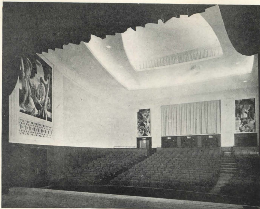
Fig. 15: Indiana University Theater. Walls funnel in toward the stage, walls and ceiling being paneled with sound-absorbing material and broken surfaces to control sound
