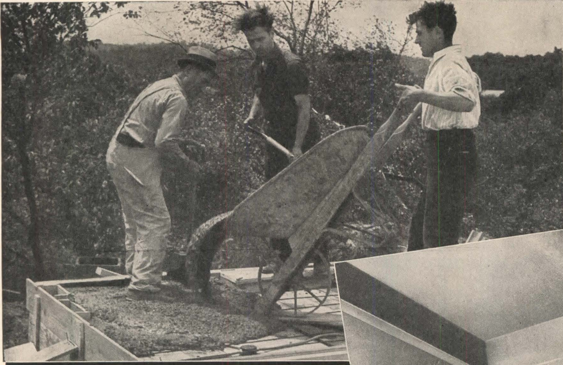
Pouring concrete to encase the ends and top flanges of the beams which provides a rigid, non-shrinking base under the whole house. Boxes in the left corner are for heat ducts. Supports for studs are provided around the stair well.
