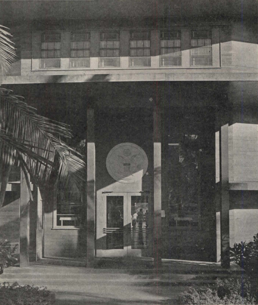
Left: Main entrance to Building "A" has two-story wood columns and recessed lanai. The great seal of the United States is made of built-up plywood finished with aluminum paint. The lobby opens to the main passage to Building "B". Left below: main entrance lobby of Building "A". Fluted columns are painted a rich blue-green. The mural was designed by Master Sergeant William R. Domaratus. Site conditions at the entrance, and the road elevation in front of the building, made it necessary to keep the entrance high to prevent having the building appear to be down in a hole. The lobby floor was therefore raised two steps above the rest of the first floor. Center: this view of the Commanding General's office shows the plywood wall finish, asphalt tile floor and acoustical ceiling. Fluorescent lighting is recessed in a 6-in. furred space in the ceiling; this space is available throughout the building for the complicated communications wiring. Right below: main axis corridor from lobby of Building "A" to third floor balcony of Building "B"
